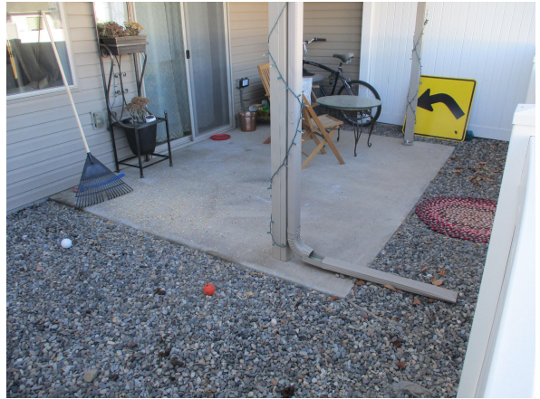
Typical rear patio
