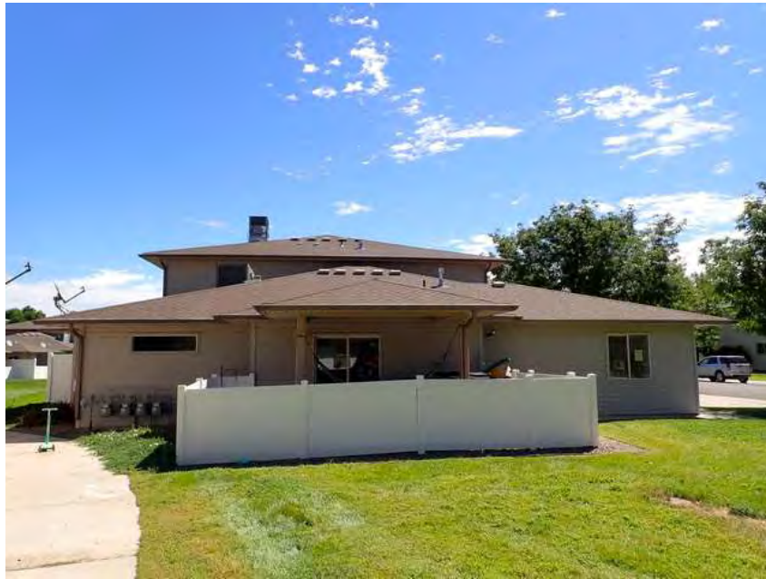
201. Building 12. Left overview.
