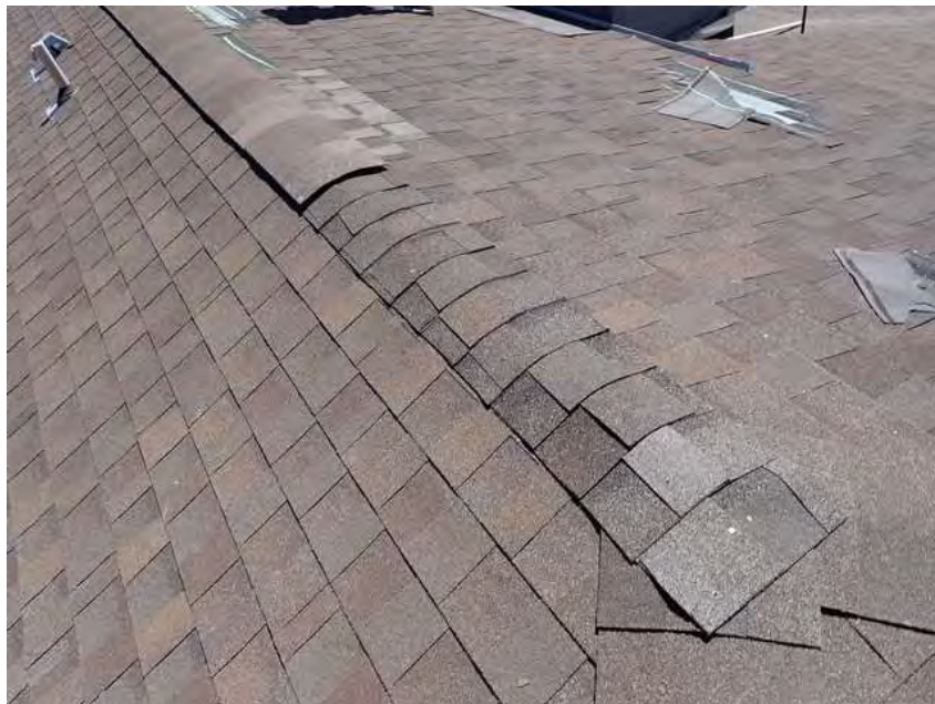
108. Building 6 Repair to ridge with cut shingles.
