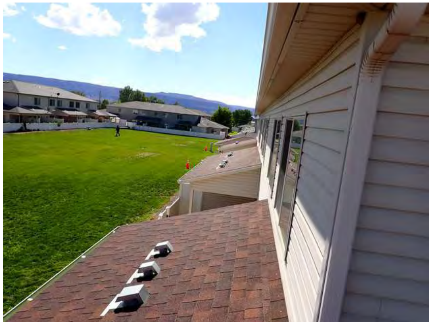
294. Building 17. Lower roof overview.
