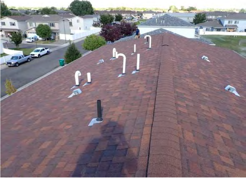
303. Building 17. Roof overview.
