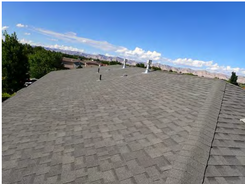
266. Building 15. Roof overview.
