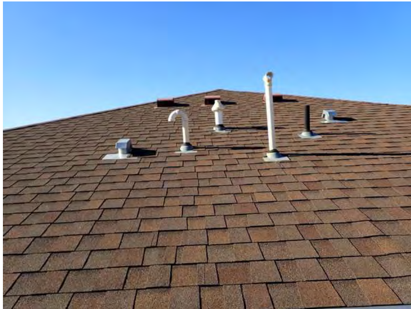
357. Building 21. Roof overview.
