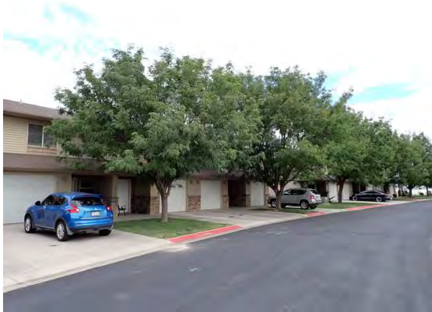
1. Building 1. Front overview.
