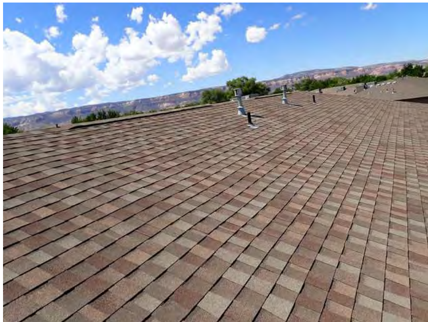
88. Building 5. Roof overview.
