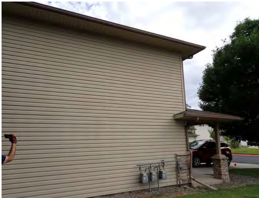
10. Building 1. Left overview.
