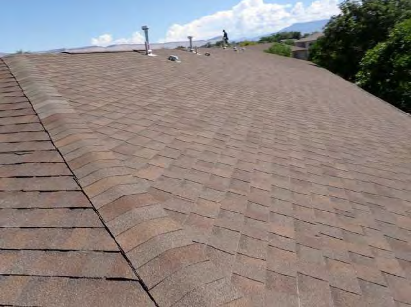
179. Building 10. Roof overview.
