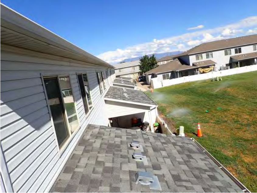
314. Building 18. Lower roof overview.
