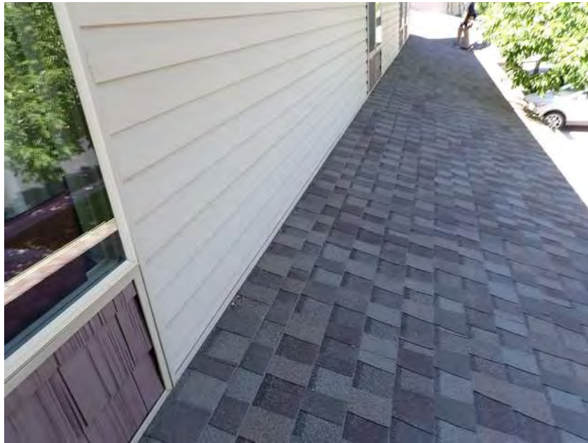
83. Building 5. Lower roof overview.
