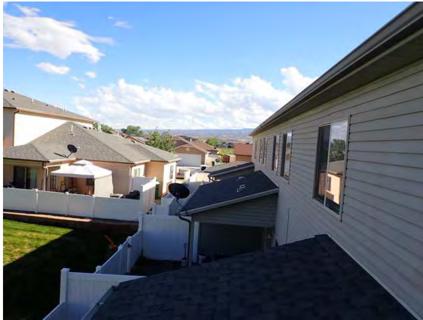
263. Building 15. Lower roof overview.
