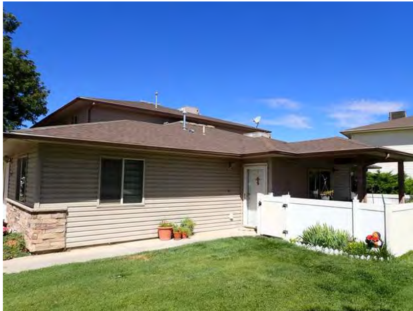
169. Building 10. Right overview.
