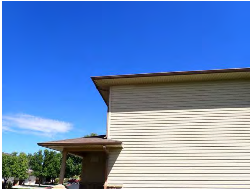
157. Building 9. Siding repair.
