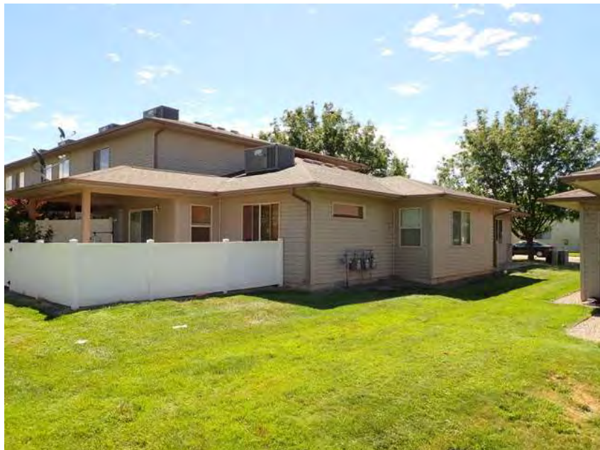
186. Building 11. Left overview.
