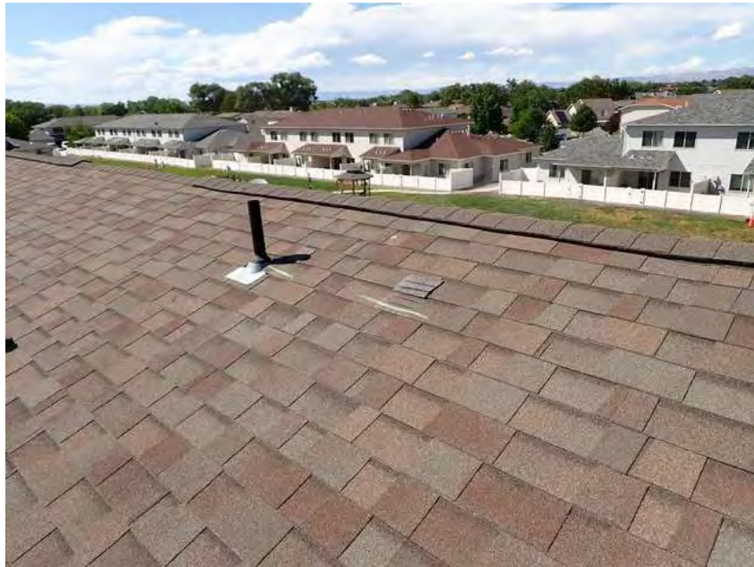
381. Building 22. Roof overview.
