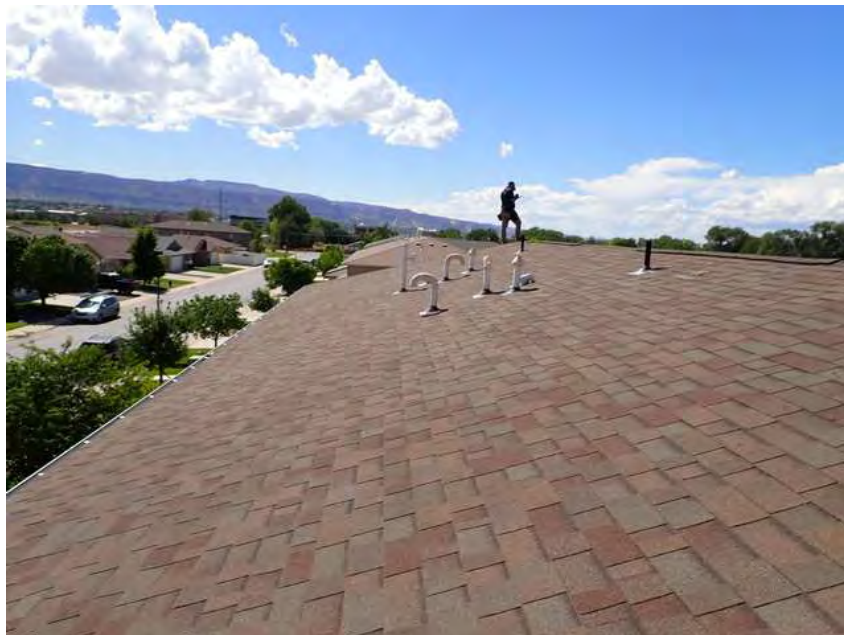
380. Building 22. Roof overview.
