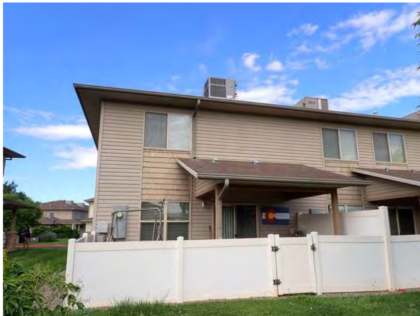
144. Building 8. Back overview.
