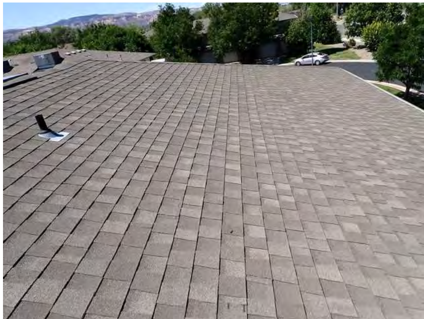
70. Building 4. Roof overview.
