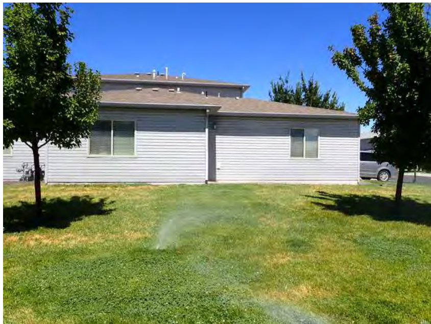
324. Building 19. Left overview.
