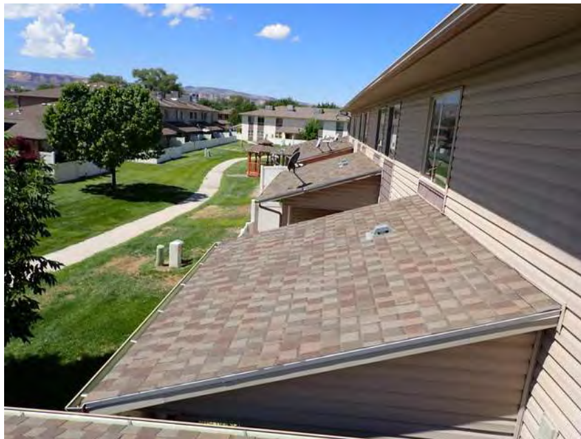
82. Building 5. Lower roof overview.
