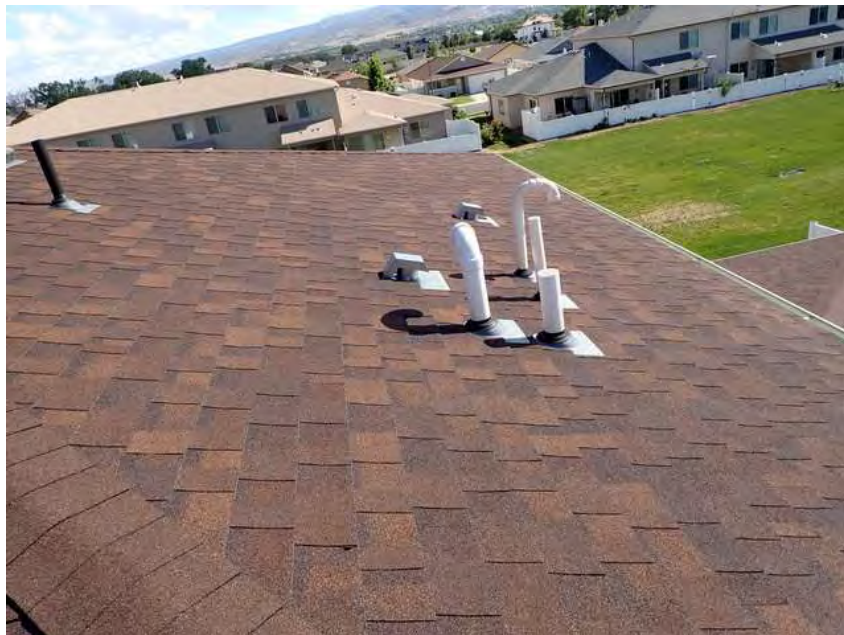
300. Building 17. Roof overview.
