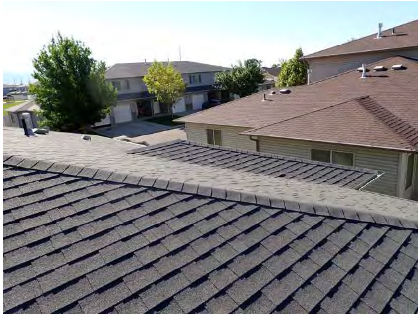
226. Building 13. Roof overview.
