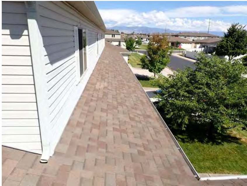
375. Building 22. Lower roof overview.
