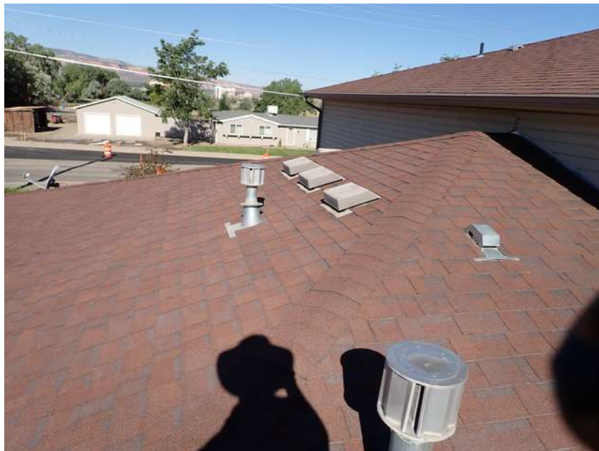
248. Building 14. Roof overview.
