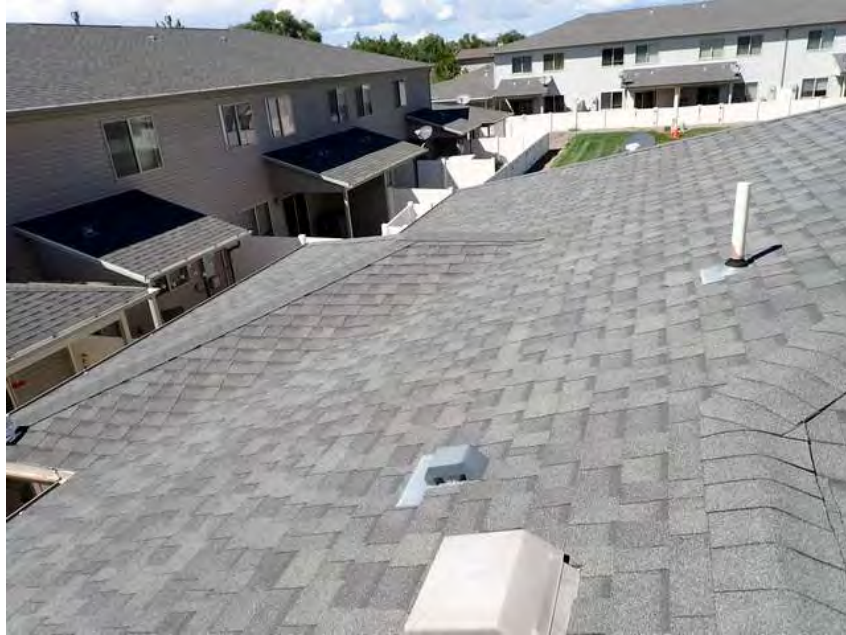
421. Building 24. Roof overview.
