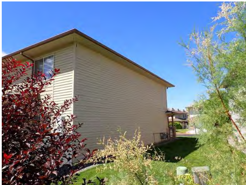
162. Building 9. Left overview.
