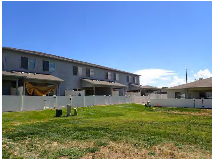
322. Building 19. Back overview.
