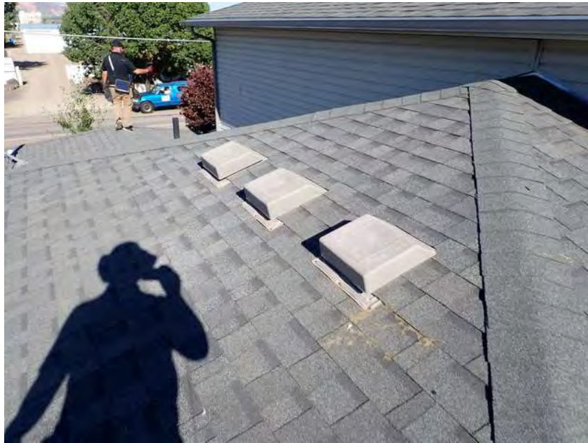
223. Building 13. Roof overview.
