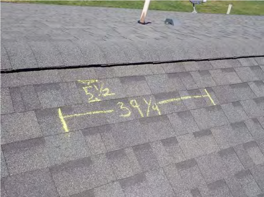
432. Building 24. Shingle dimensions.
