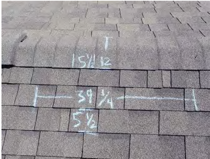
285. Building 16. Shingle dimensions.
