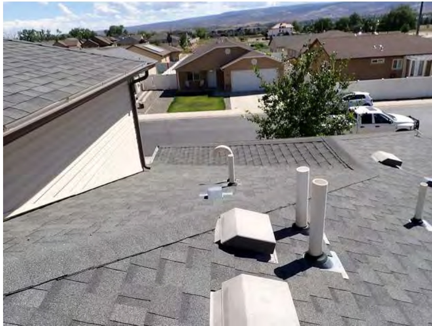
427. Building 24. Roof overview.
