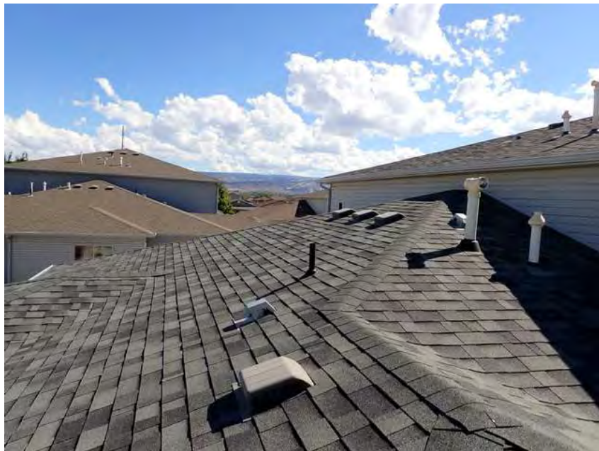
310. Building 18. Roof overview.
