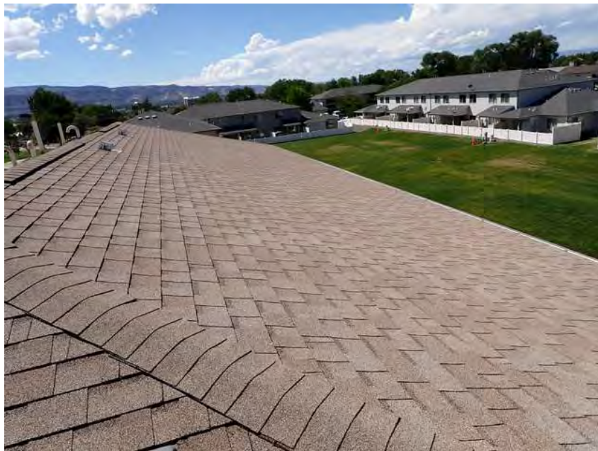
412. Building 23. Roof overview.
