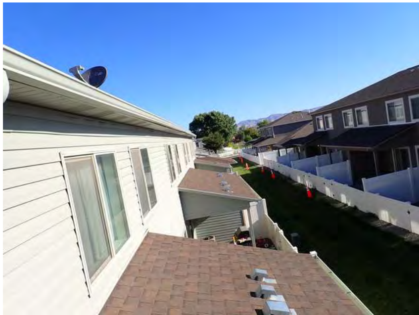
364. Building 21. Lower roof overview.
