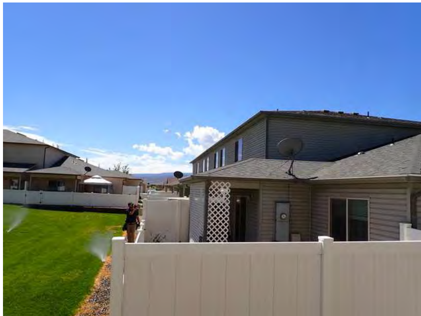
258. Building 15. Left overview.
