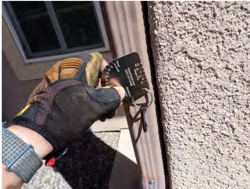
439. Club House. Gutters made from aluminum.
