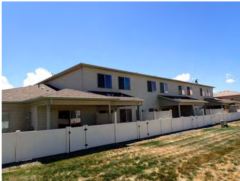
366. Building 22. Back overview.
