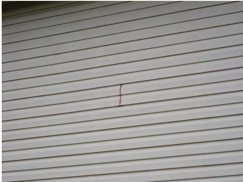
130. Building 7. Sealed gap in siding.
