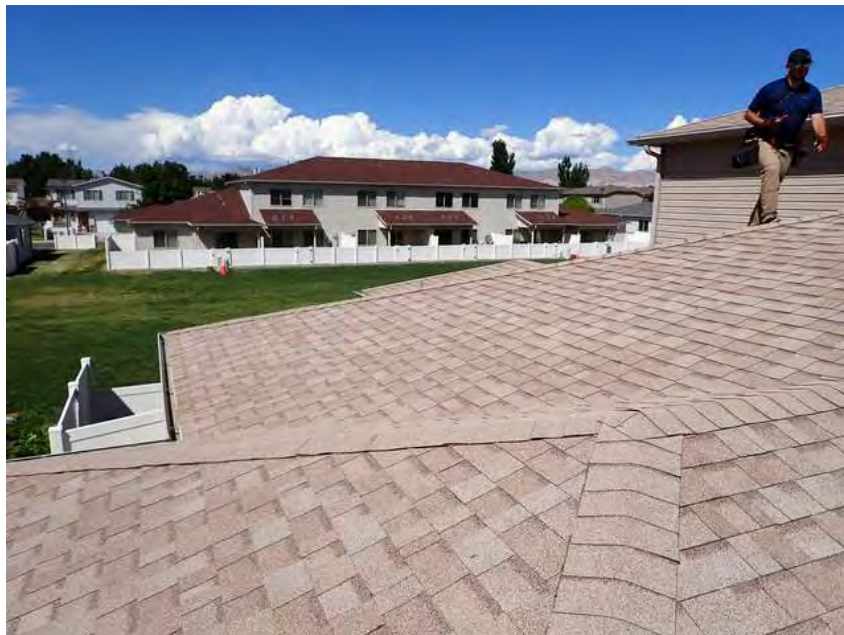
404. Building 23. Roof overview.
