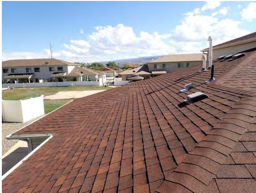
291. Building 17. Roof overview.
