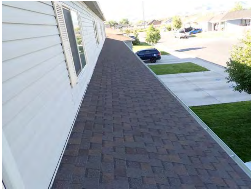
363. Building 21. Lower roof overview.
