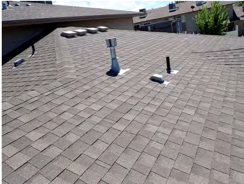
65. Building 4. Roof overview.
