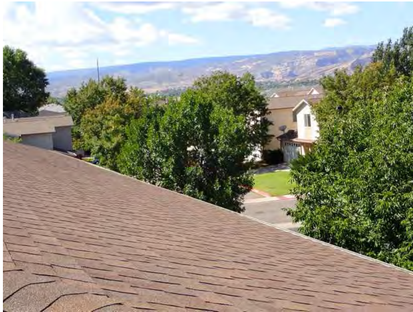
163. Building 9. Roof overview.
