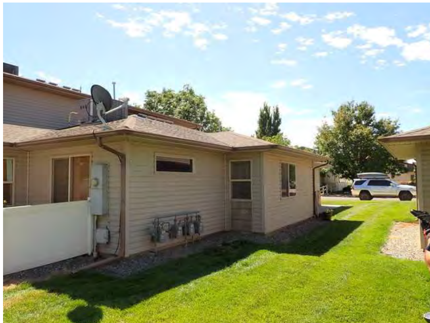
172. Building 10. Left overview.
