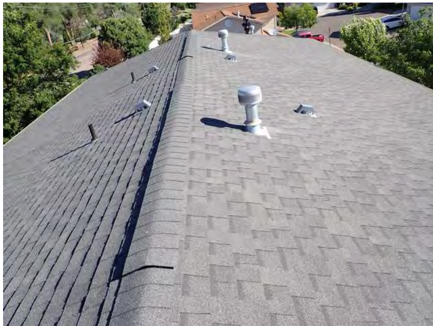
236. Building 13. Roof overview.
