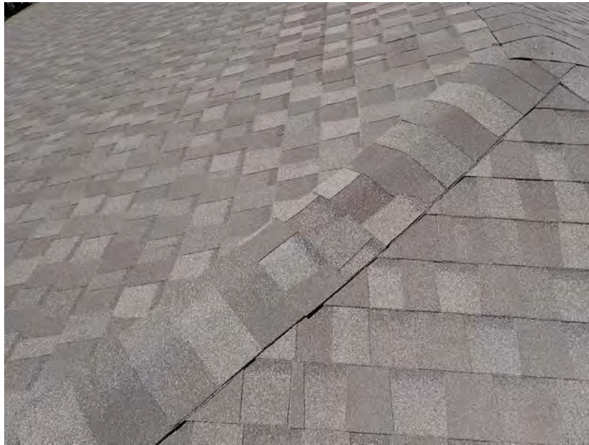
193. Building 11. Repair to ridge cap with cut shingles.
