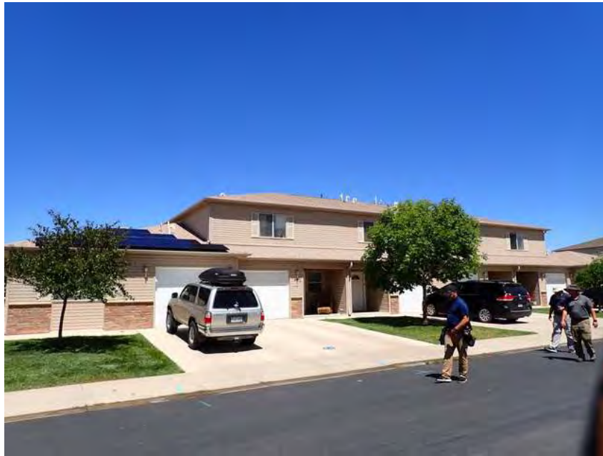
399. Building 23. Front overview.
