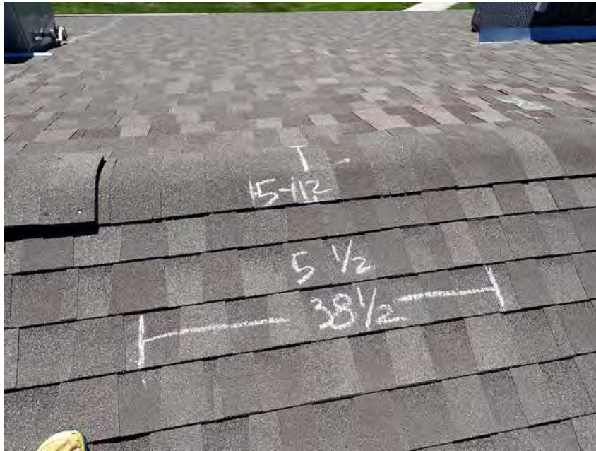
71. Building 4. Shingle dimensions.
