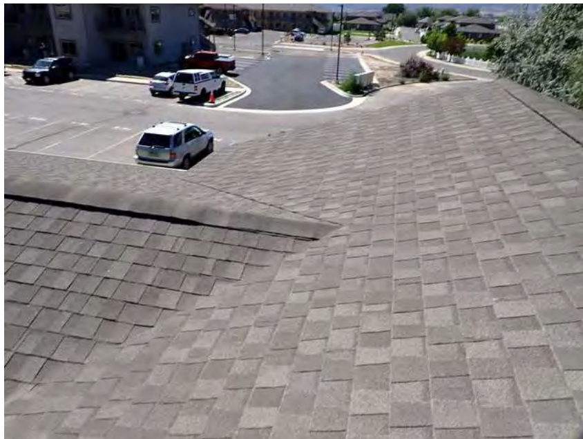
448. Club House. Roof overview.
