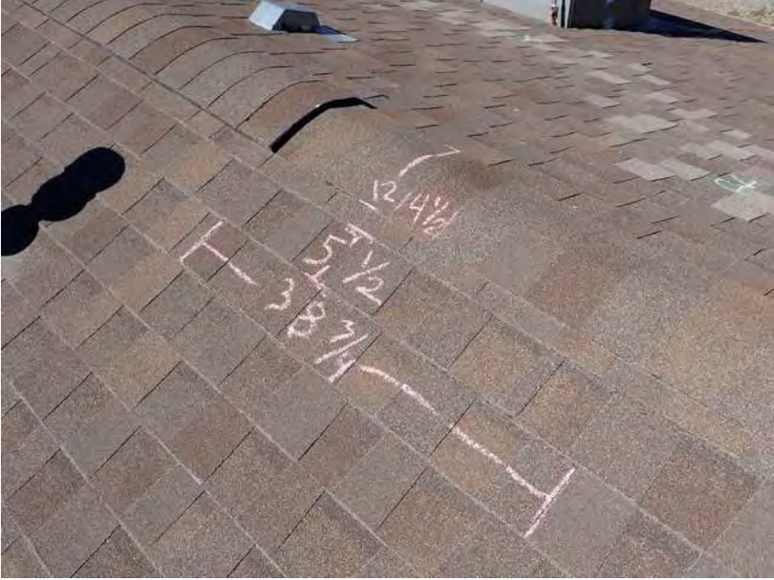
25. Building 1. Dimensions of primary shingle.
