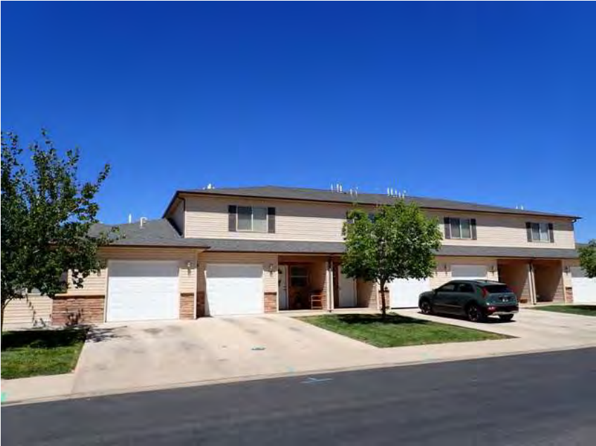
414. Building 24. Front overview.
