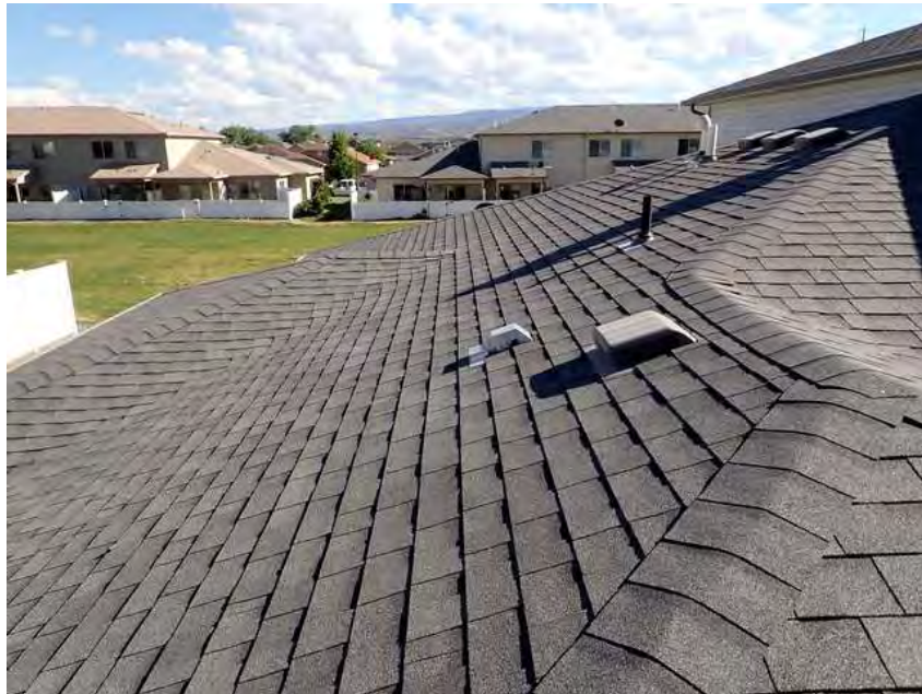
279. Building 16. Roof overview.
