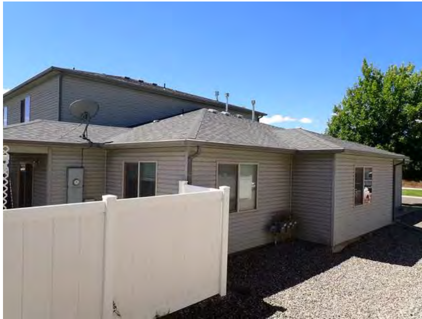
259. Building 15. Left overview.
