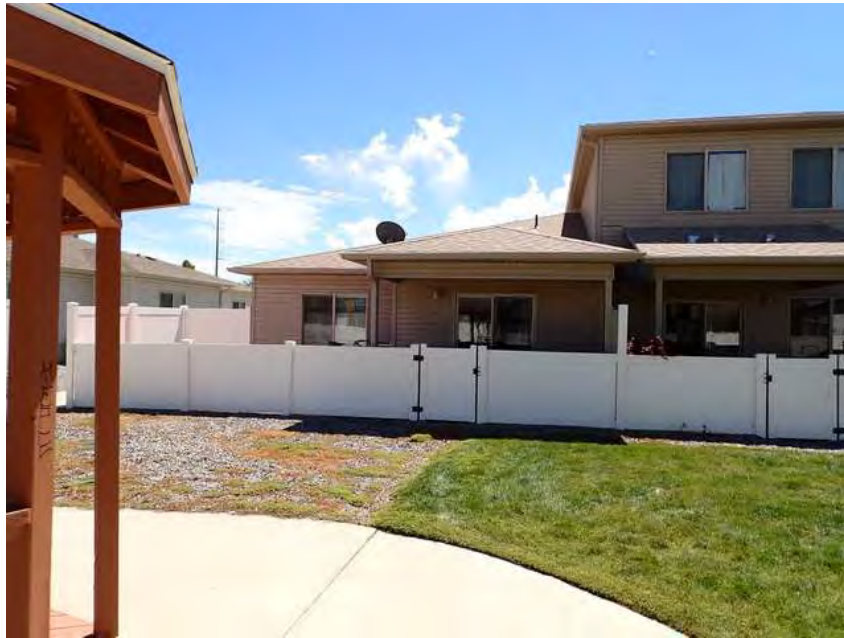
401. Building 23. Back overview.
