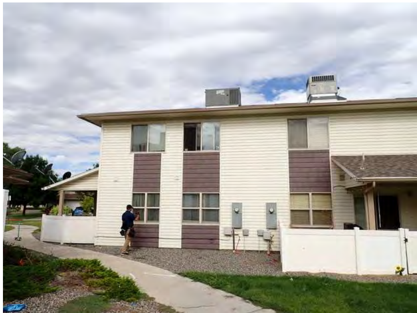
46. Building 3. Back overview.
