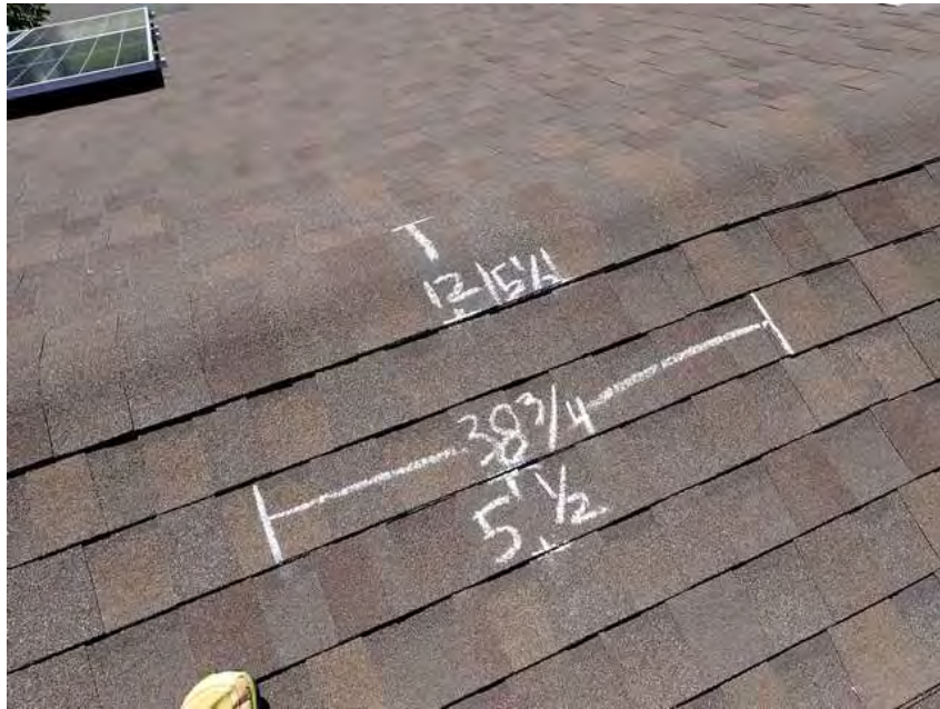
217. Building 12. Shingle dimensions.
