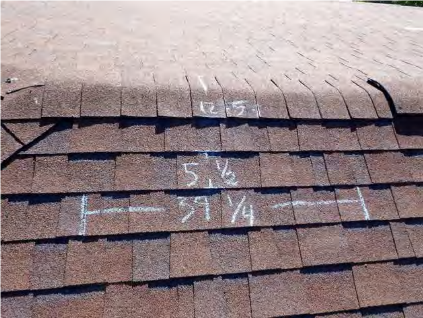
252. Building 14. Shingle dimensions.
