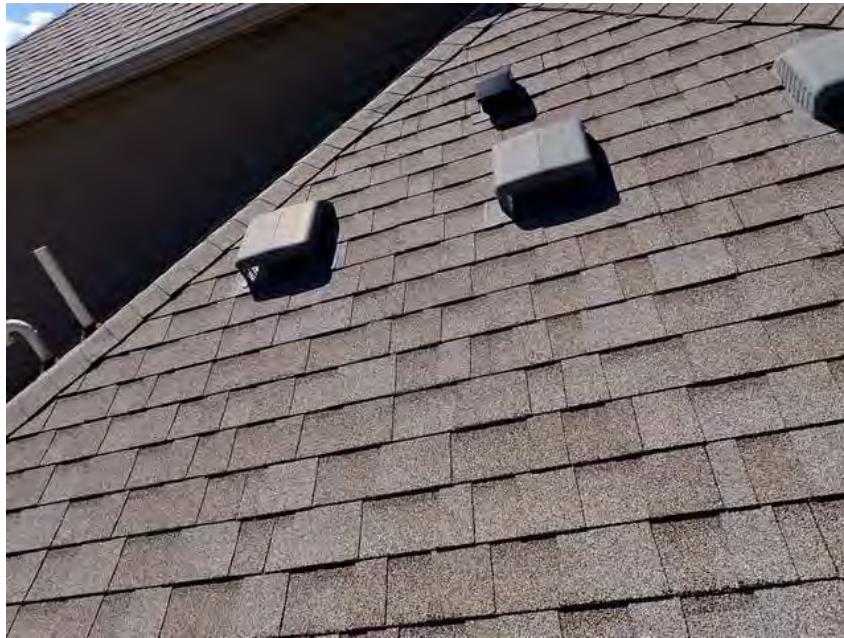
411. Building 23. Roof overview.
