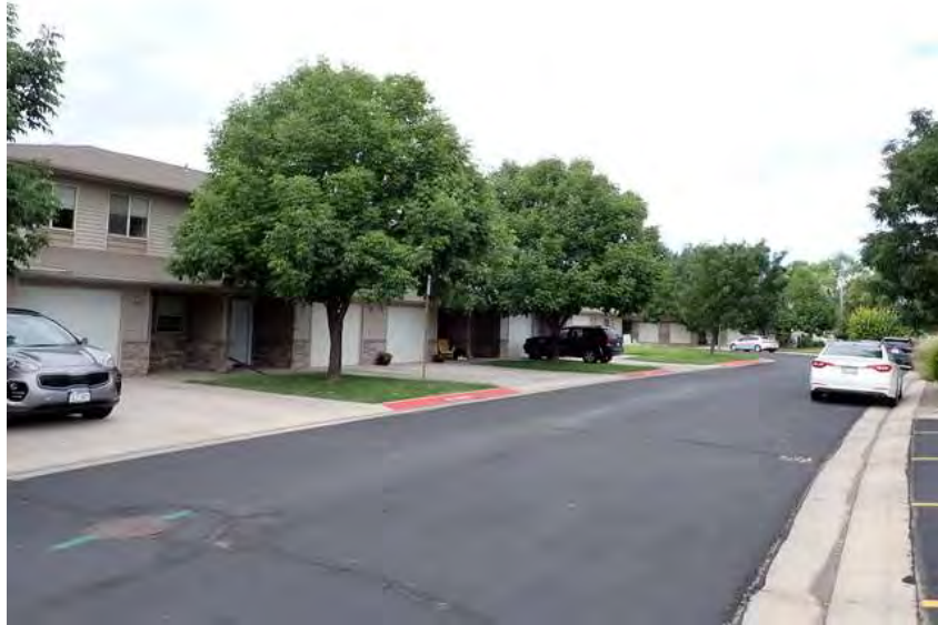
57. Building 4. Front overview.
