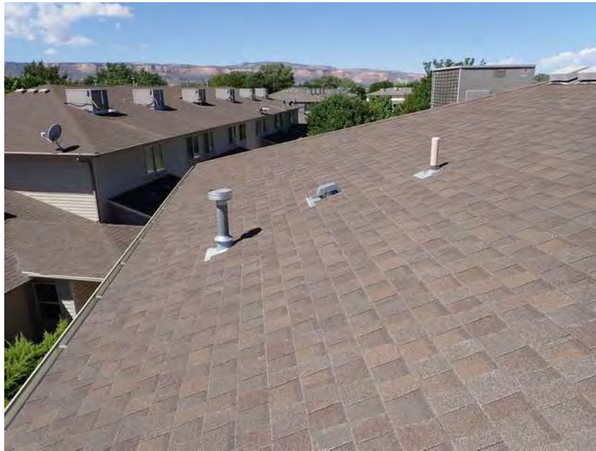
137. Building 7. Roof overview.
