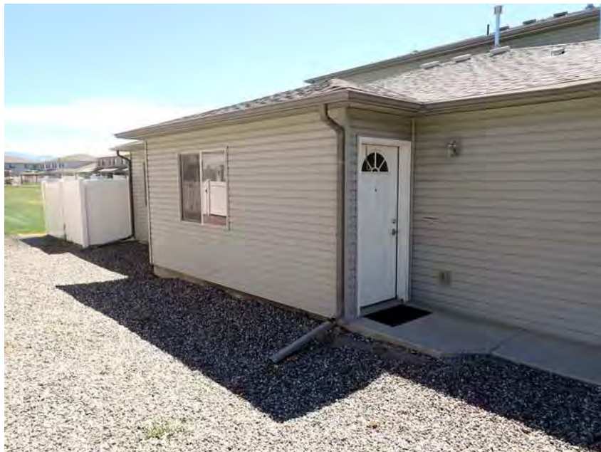
260. Building 15. Left overview.
