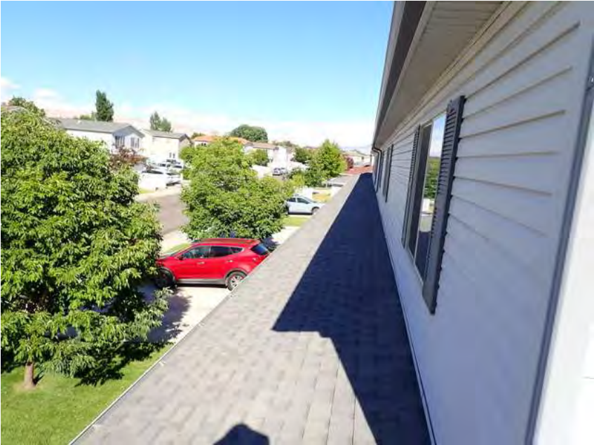
278. Building 16. Lower roof overview.
