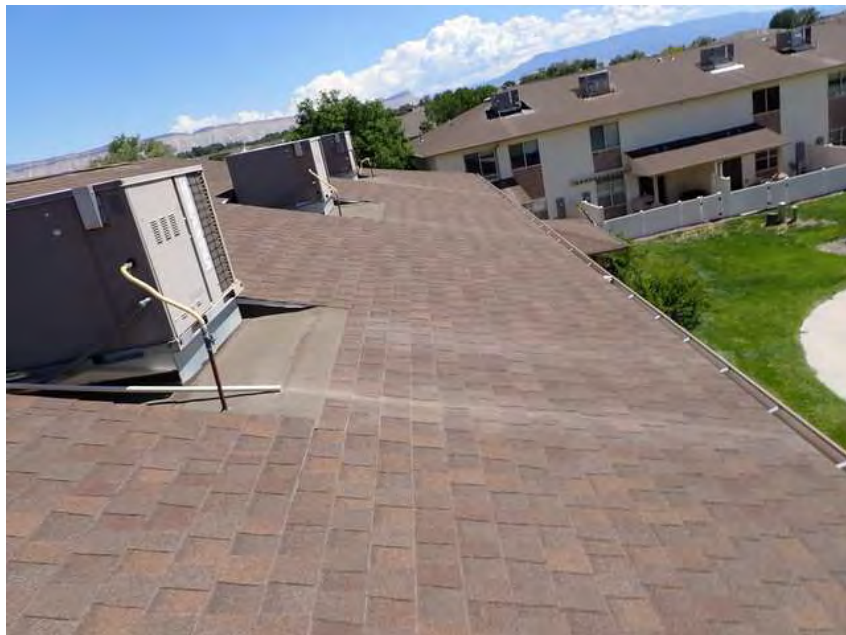
102. Building 6 Roof overview.
