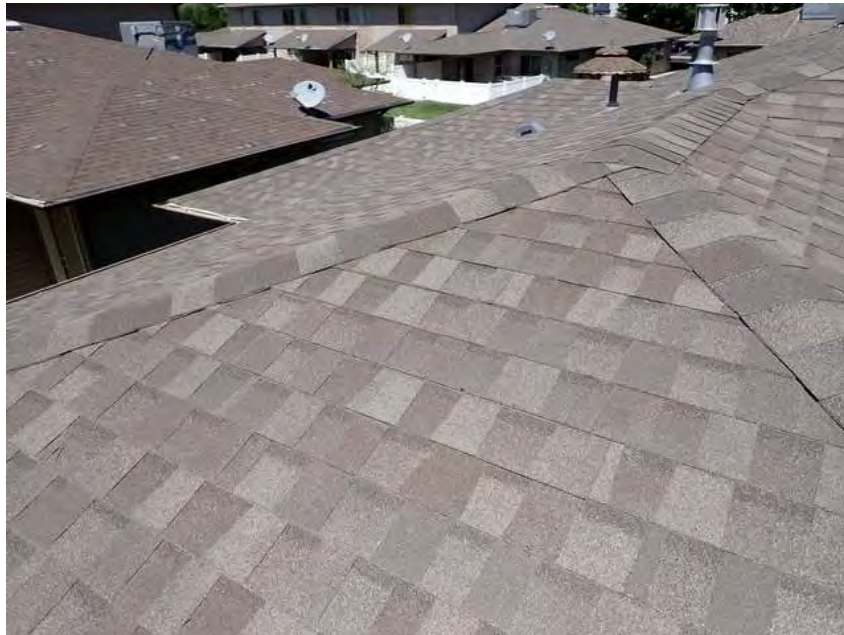
190. Building 11. Roof overview.
