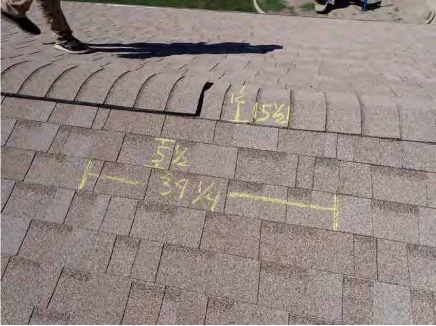
413. Building 23. Shingle dimensions.
