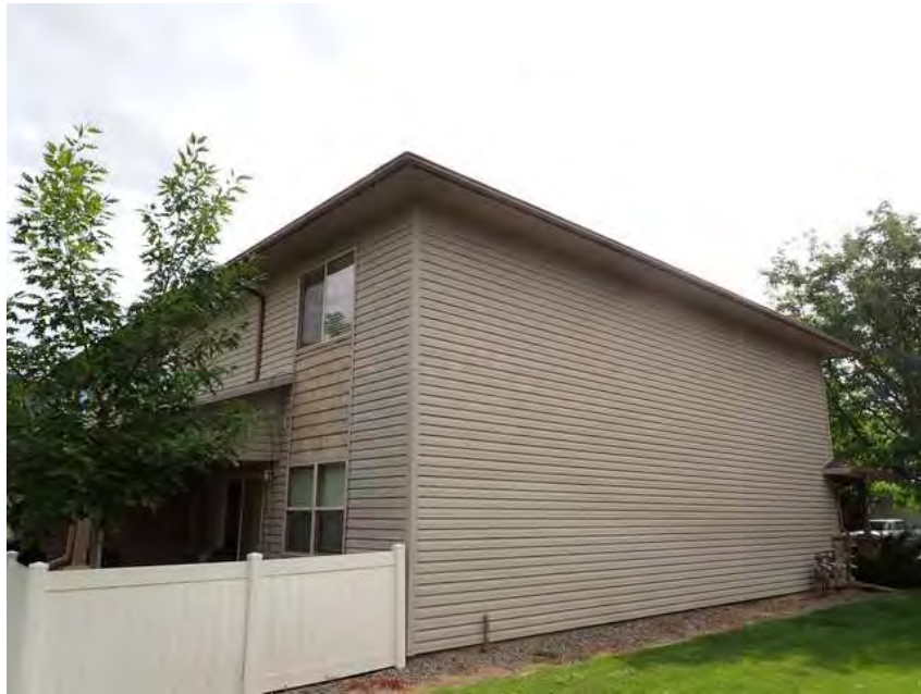
37. Building 2. Left overview.
