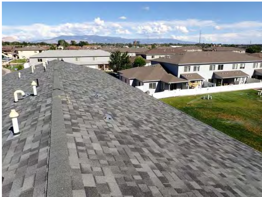
318. Building 18. Roof overview.
