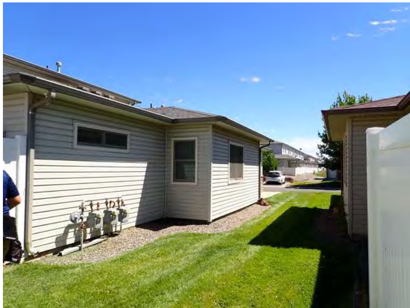
220. Building 13. Right overview.
