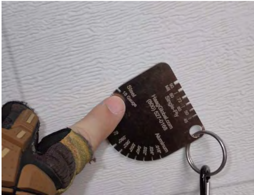
3. Building 1. Garage doors made from steel, typical throughout property.
