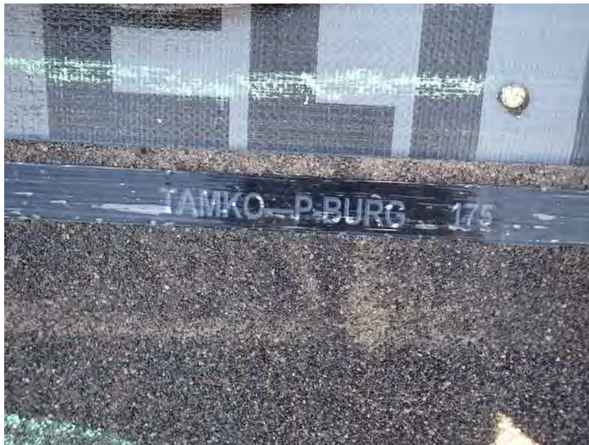
114. Building 6 Shingles on this building made by Tamko.
