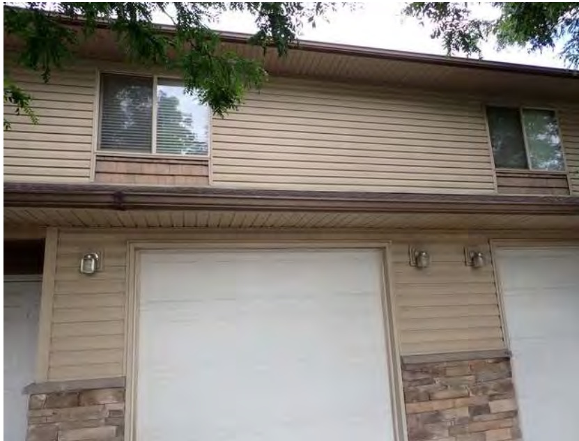
4. Building 1. Buildings 1-12 had a vinyl shake accent below windows.
