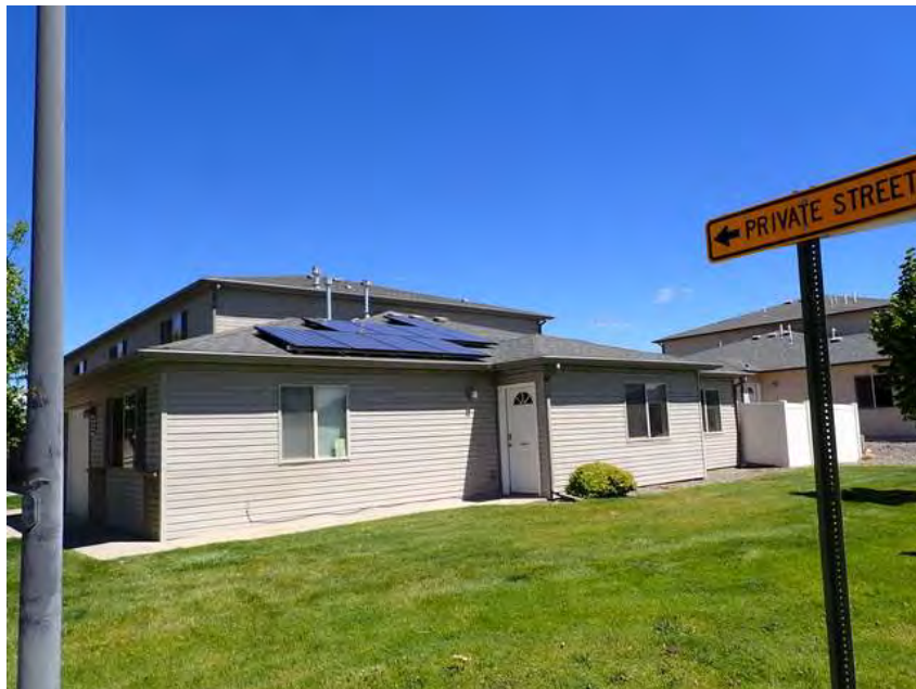
254. Building 15. Right overview.
