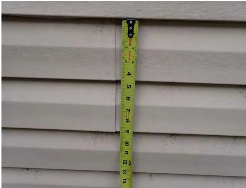
7. Building 1. Vinyl siding measured 9 inches tall.
