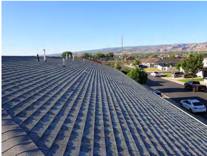
339. Building 20. Roof overview.
