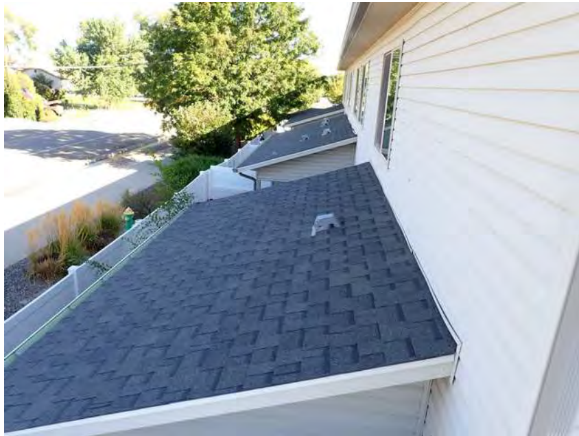
225. Building 13. Lower roof overview.
