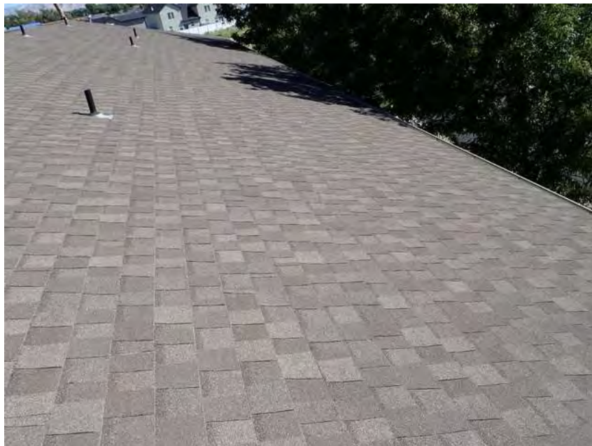
40. Building 2. Roof overview.
