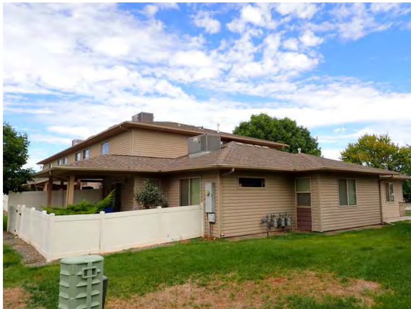
80. Building 5. Left overview.
