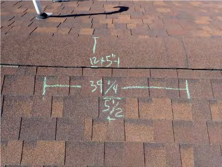
304. Building 17. Shingle dimensions.
