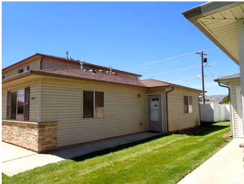
240. Building 14. Right overview.
