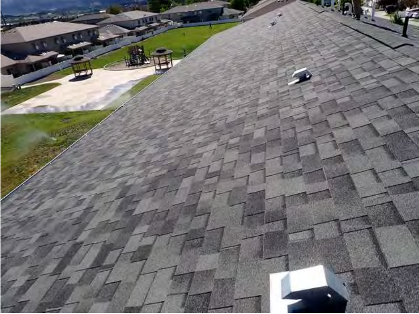
315. Building 18. Roof overview.
