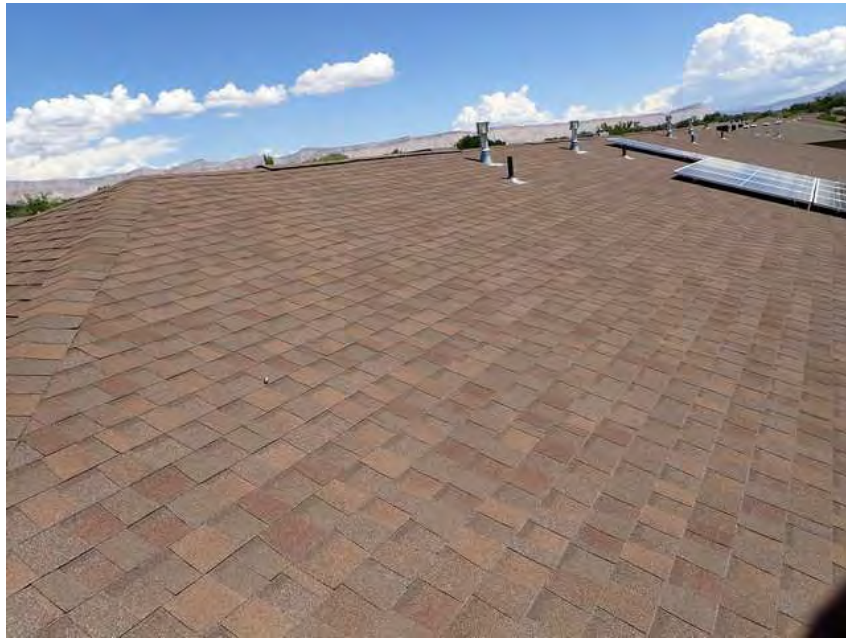
209. Building 12. Roof overview.
