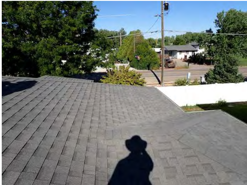
230. Building 13. Roof overview.
