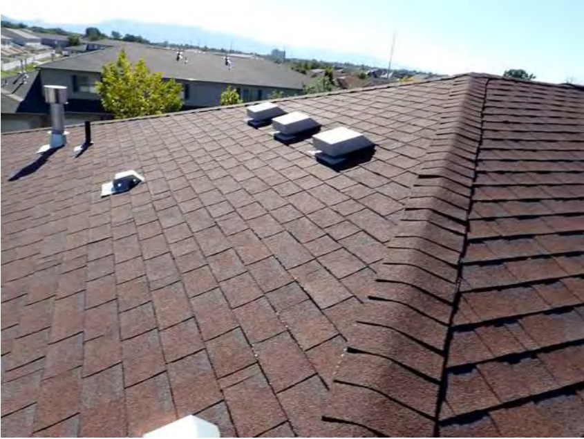
251. Building 14. Roof overview.
