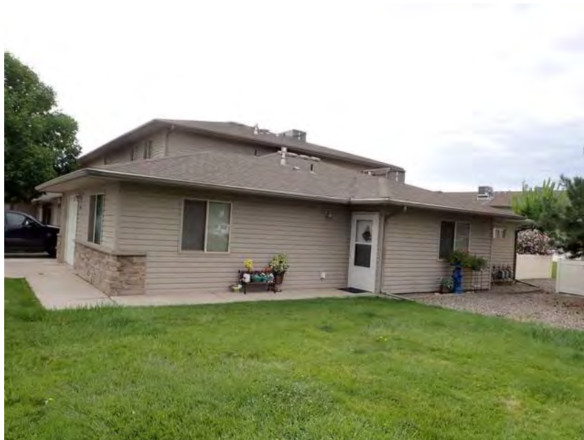
58. Building 4. Right overview.
