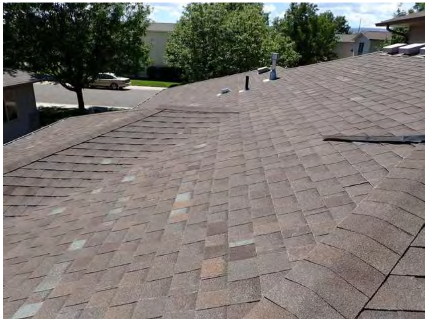
204. Building 12. Roof overview.
