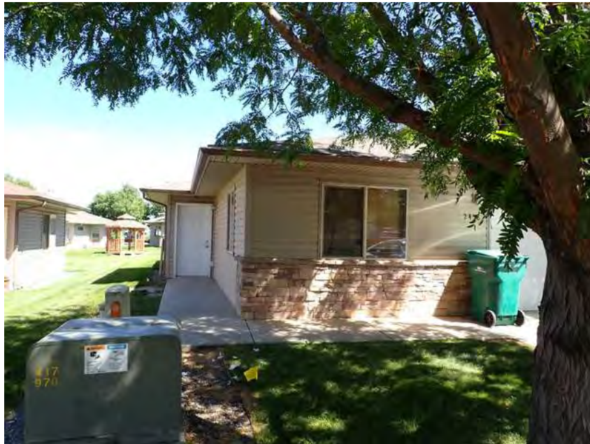
182. Building 11. Front overview.
