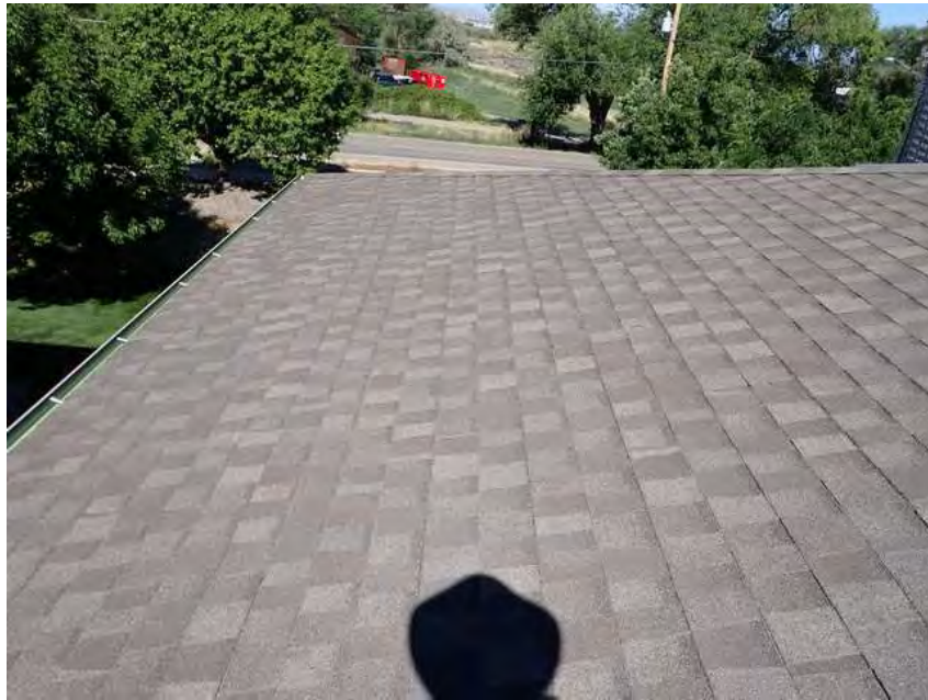
39. Building 2. Roof overview.
