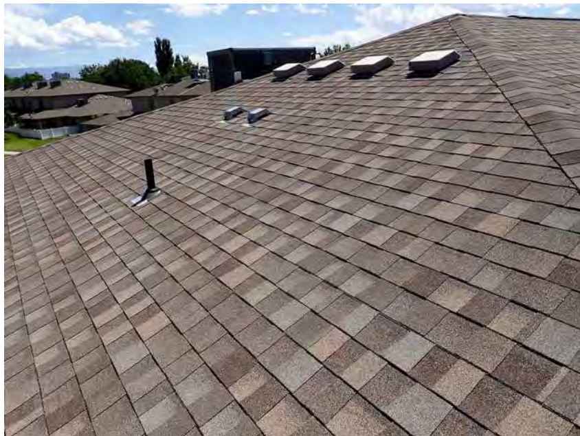
52. Building 3. Vent boxes and other appurtenances.
