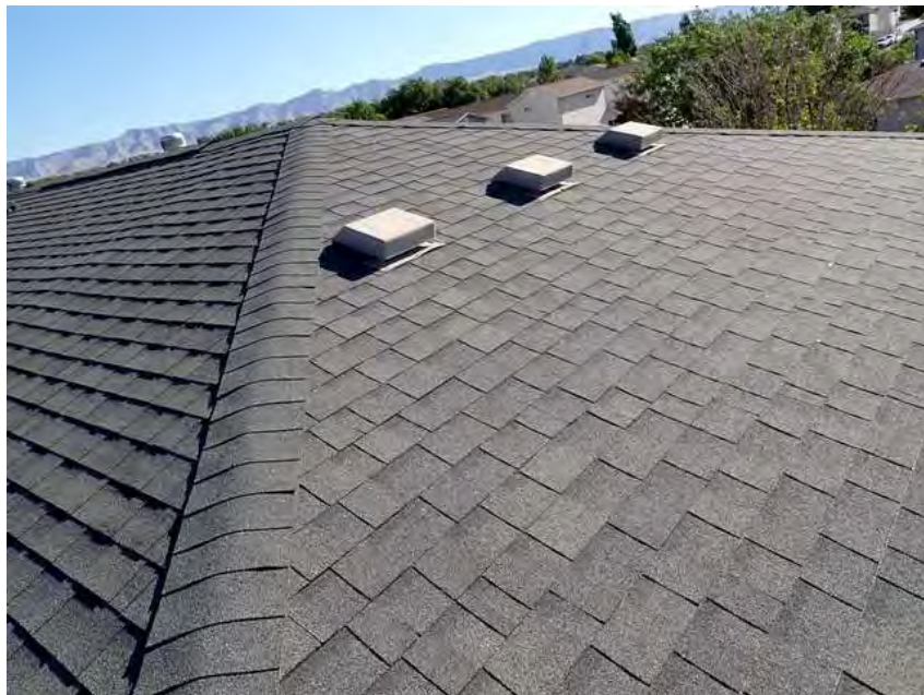
234. Building 13. Roof overview.
