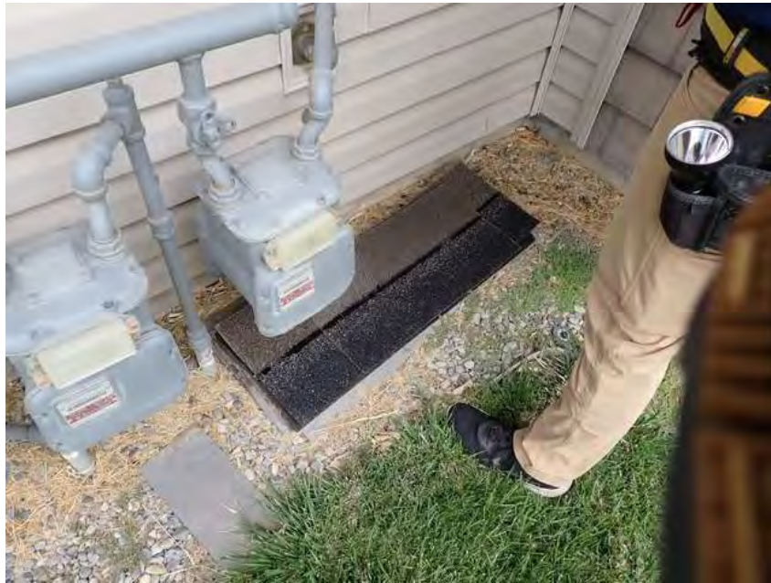
61. Building 4. Found shingles.
