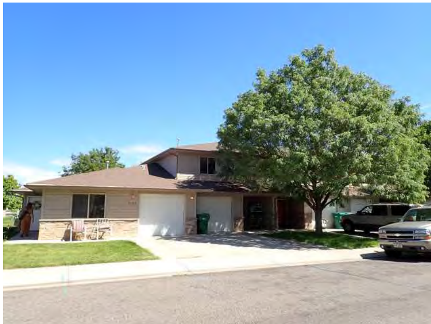
168. Building 10. Front overview.
