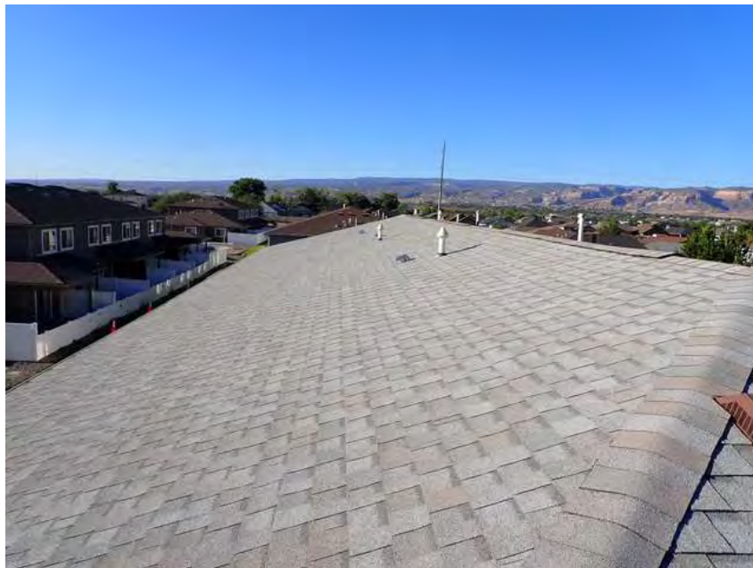
342. Building 20. Roof overview.
