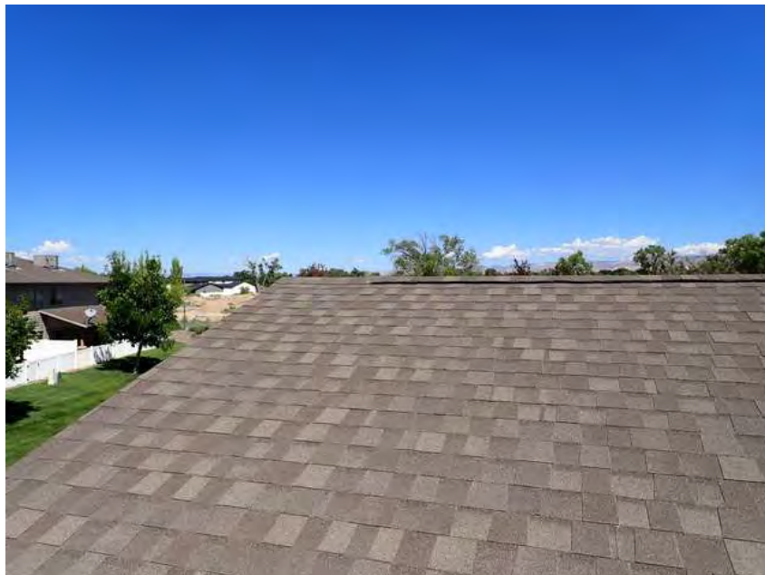
444. Club House. Roof overview.
