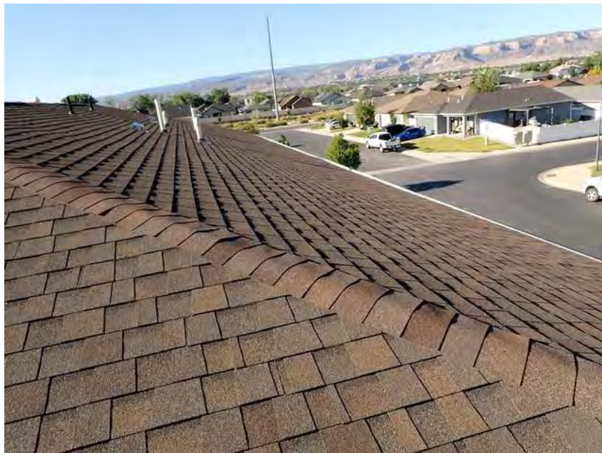
358. Building 21. Roof overview.
