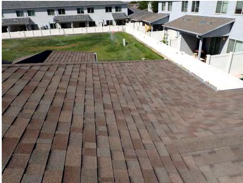
377. Building 22. Roof overview.
