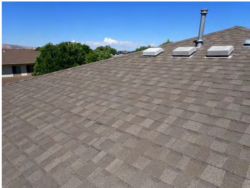
148. Building 8. Roof overview.
