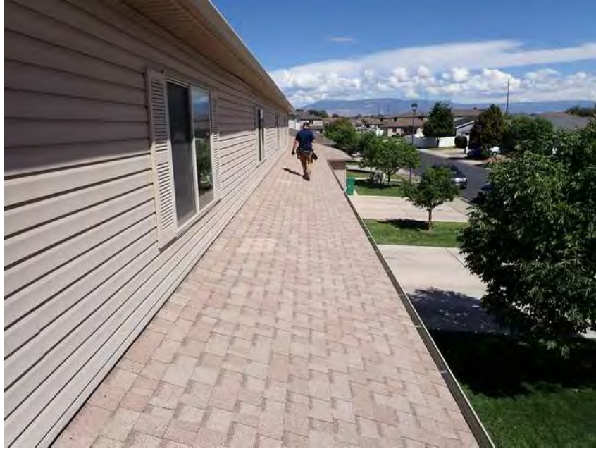
409. Building 23. Lower roof overview.
