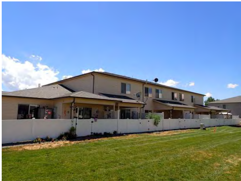
416. Building 24. Back overview.
