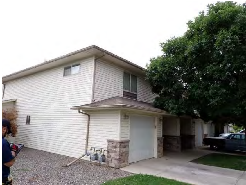
49. Building 3. Left overview.
