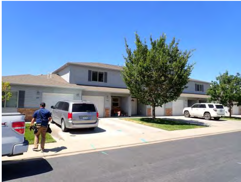
319. Building 19. Front overview.
