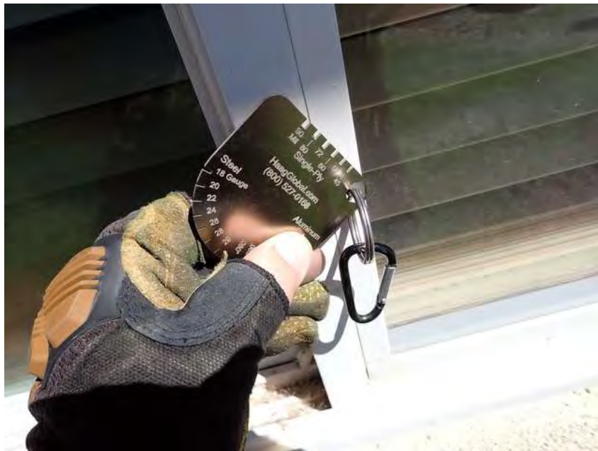
438. Club House. Gutters made from aluminum.
