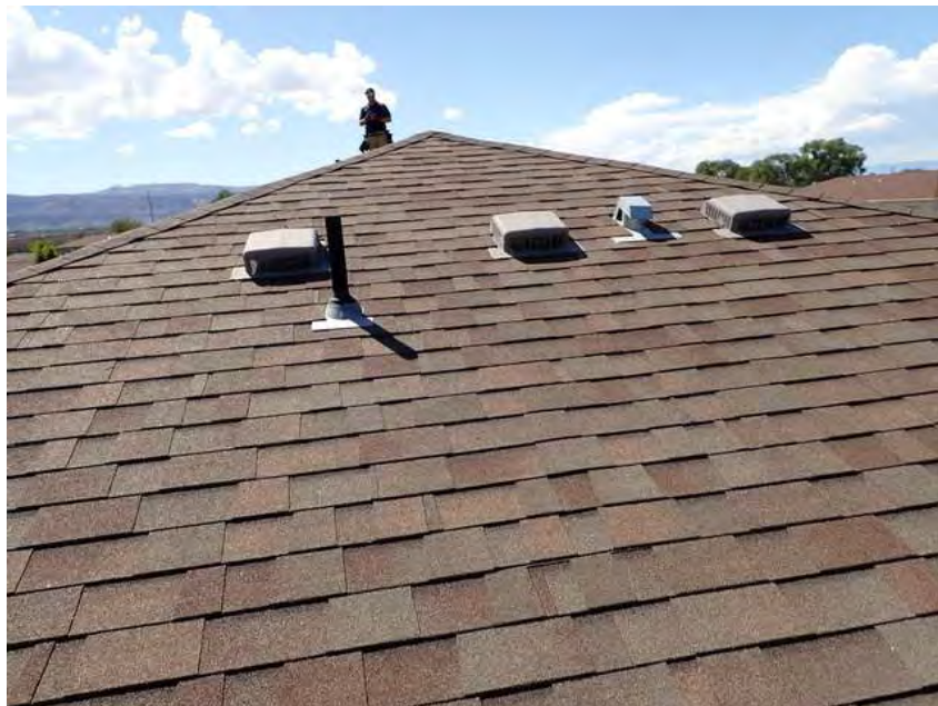
378. Building 22. Roof overview.
