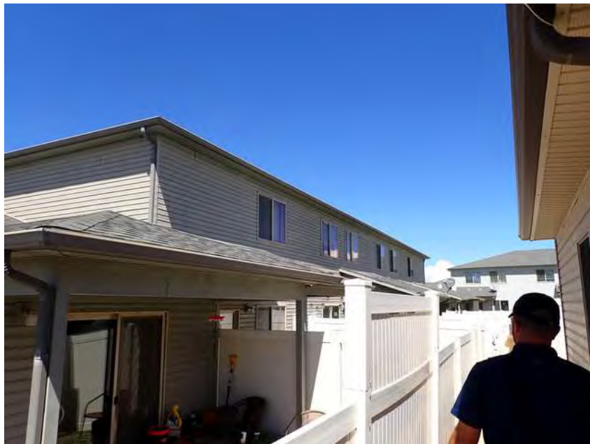
256. Building 15. Back overview.
