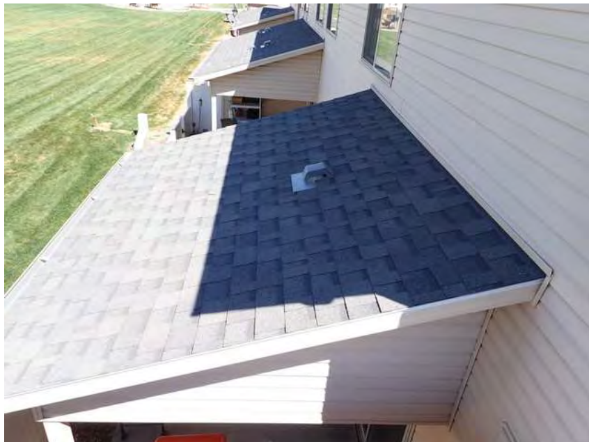
422. Building 24. Lower roof overview.
