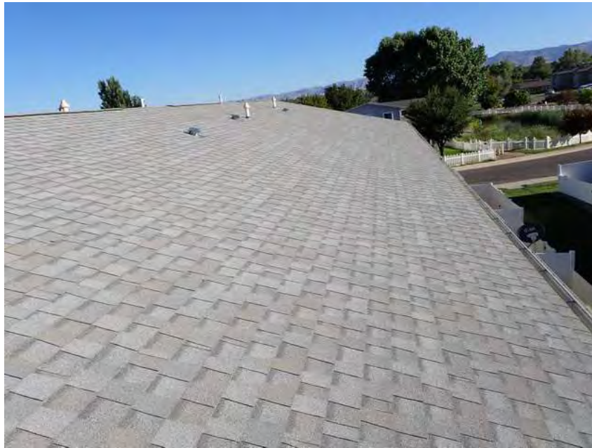
341. Building 20. Roof overview.
