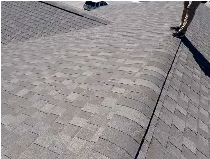
447. Club House. Roof overview.
