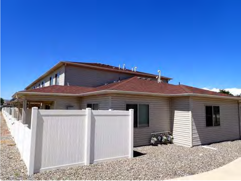
289. Building 17. Left overview.
