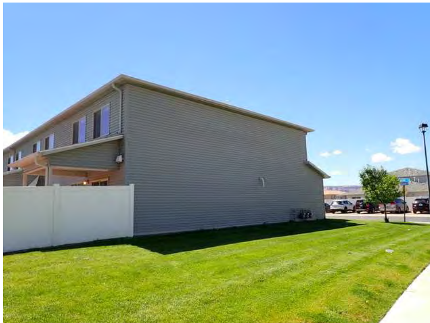
338. Building 20. Left overview.
