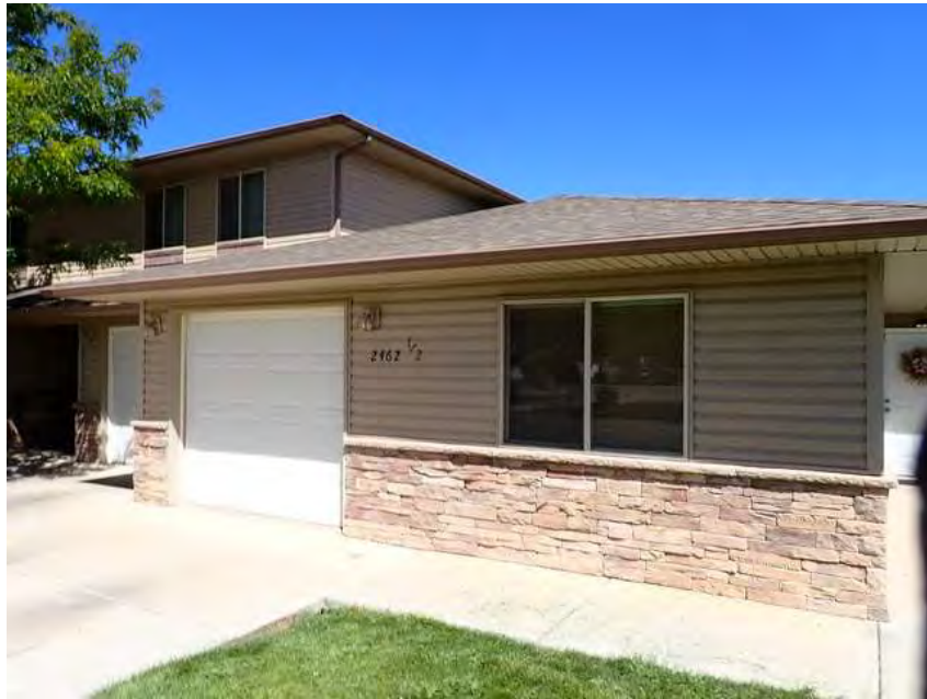
183. Building 11. Front overview.
