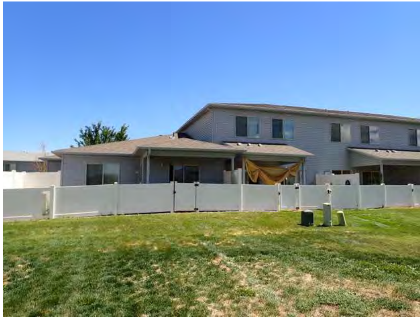
321. Building 19. Back overview.
