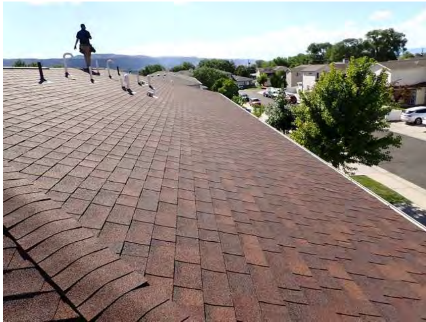
299. Building 17. Roof overview.
