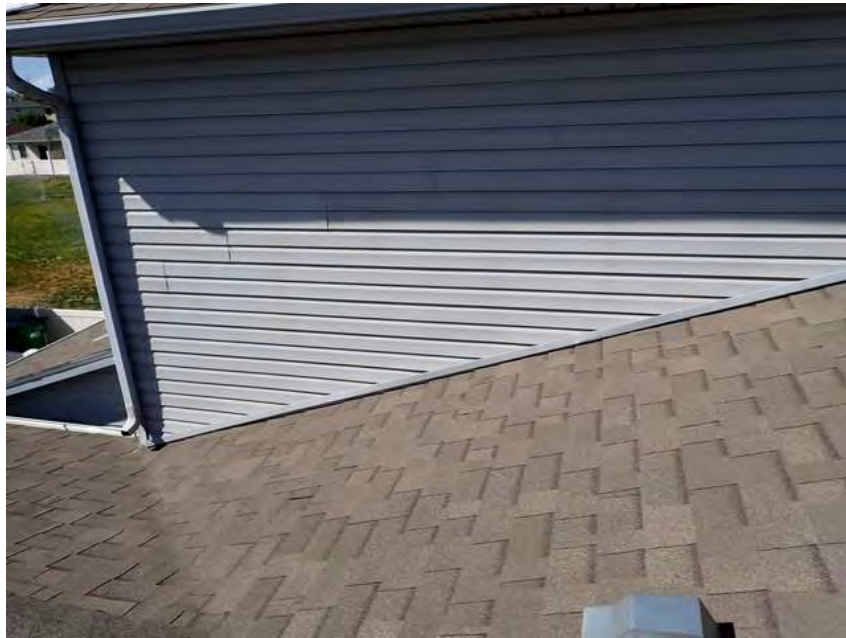
325. Building 19. Roof overview.
