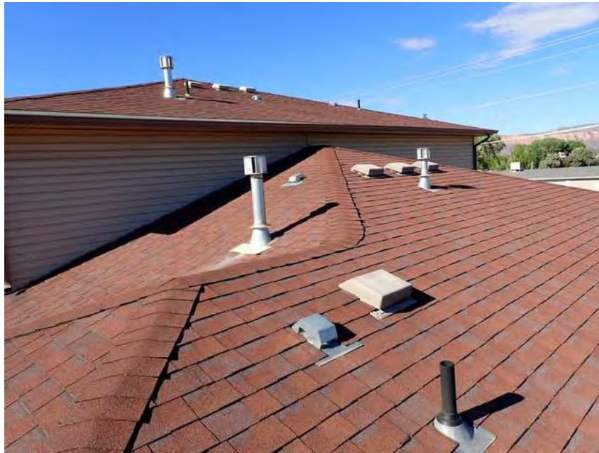
245. Building 14. Roof overview.
