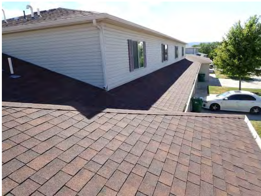
292. Building 17. Lower roof overview.
