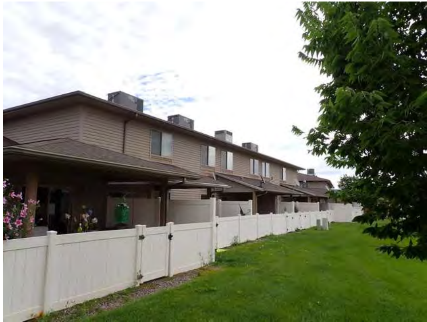
59. Building 4. Back overview.
