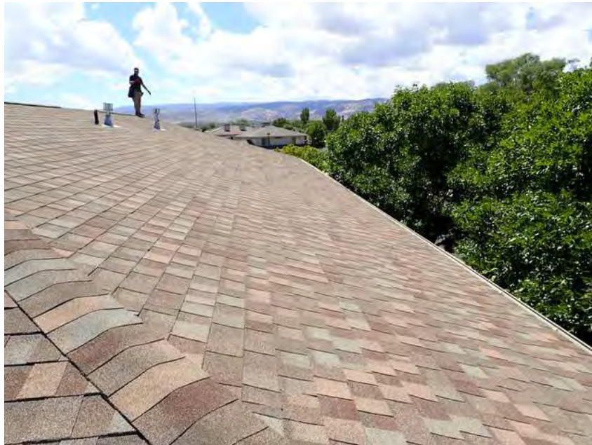
51. Building 3. Roof overview.
