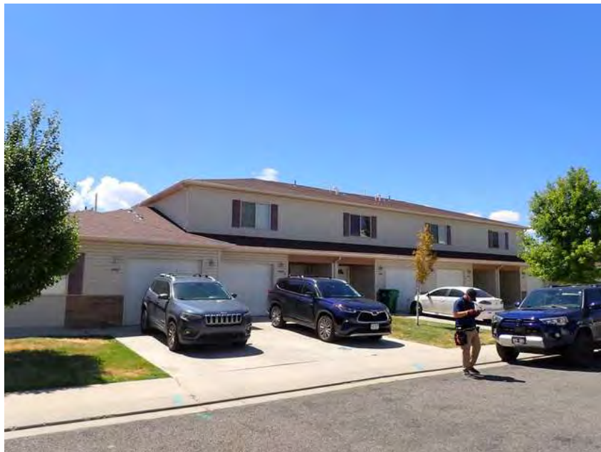
286. Building 17. Front overview.
