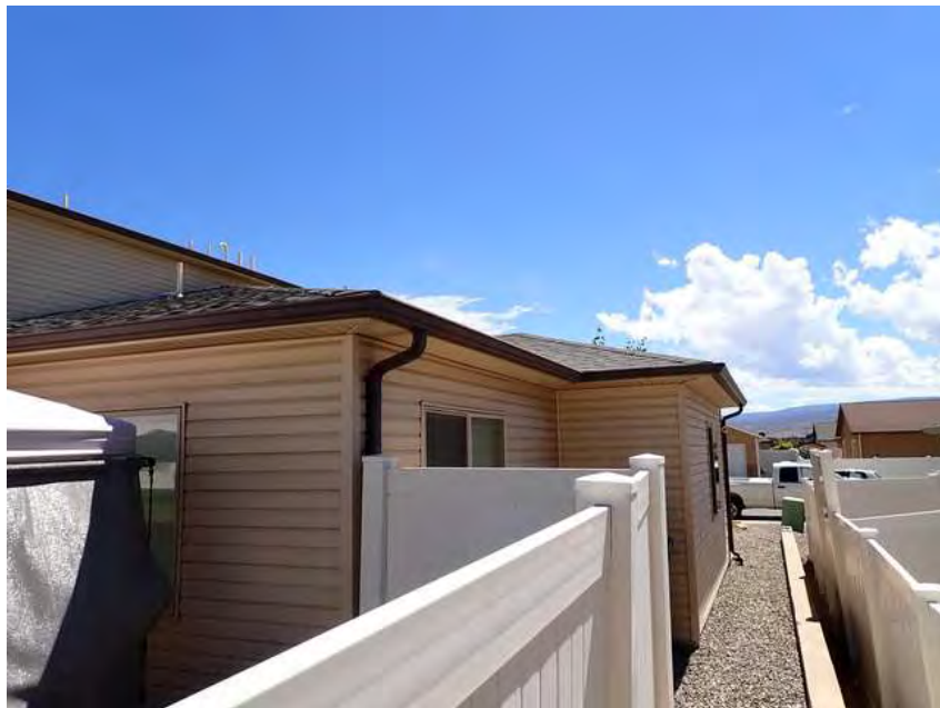
418. Building 24. Left overview.
