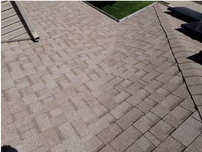
408. Building 23. Roof overview.
