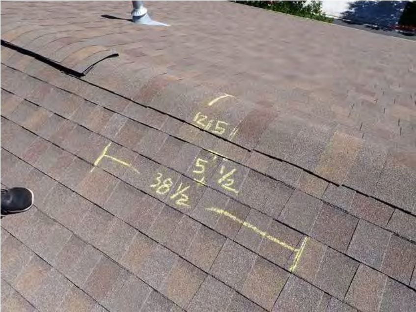
140. Building 7. Shingle dimensions.
