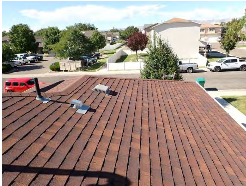
293. Building 17. Roof overview.
