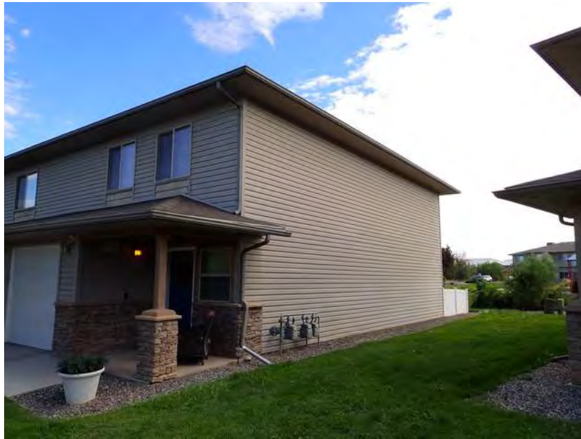
143. Building 8. Right overview.
