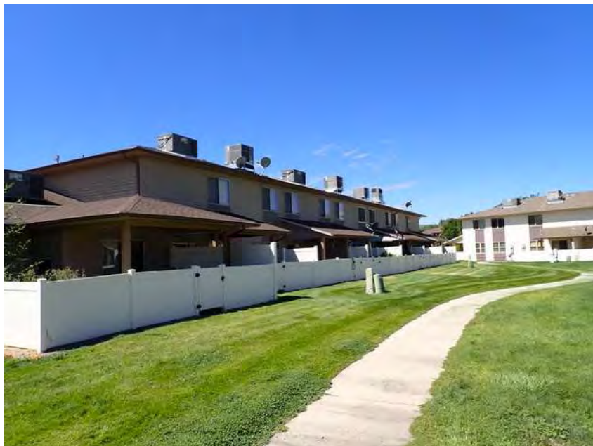
200. Building 12. Back overview.
