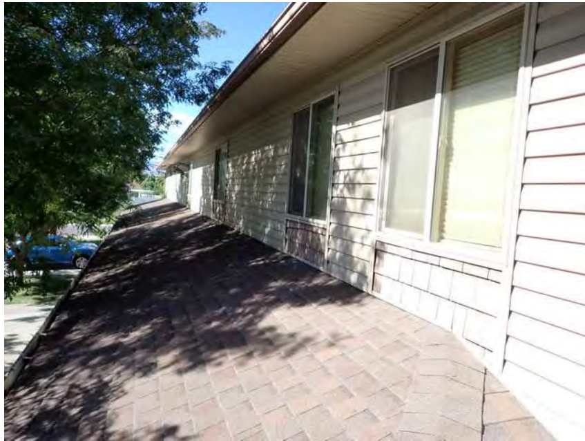
11. Building 1. Lower roof overview.
