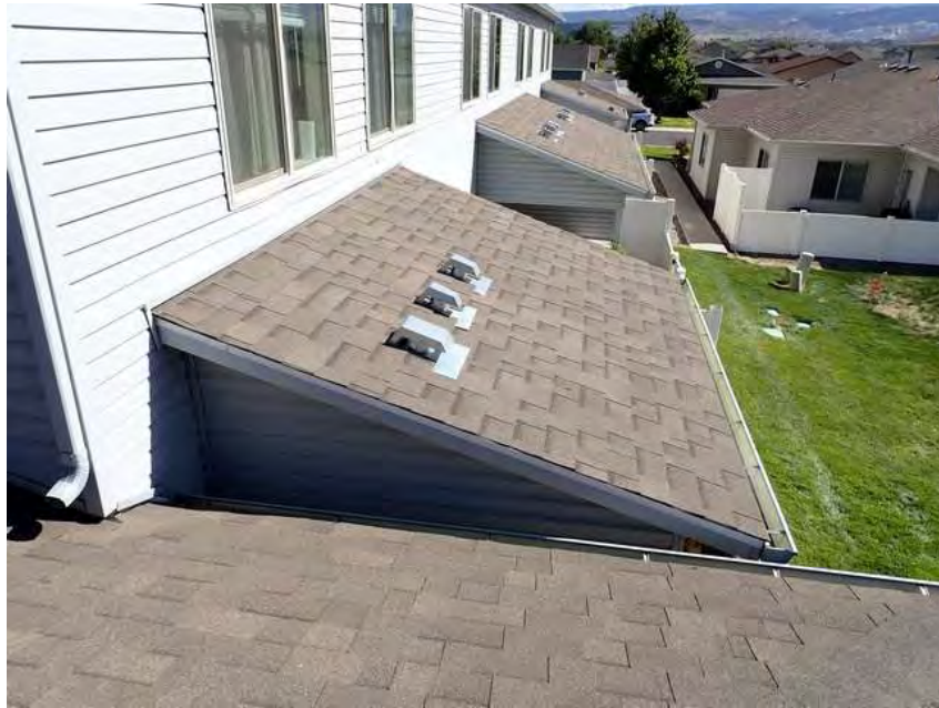
329. Building 19. Lower roof overview.
