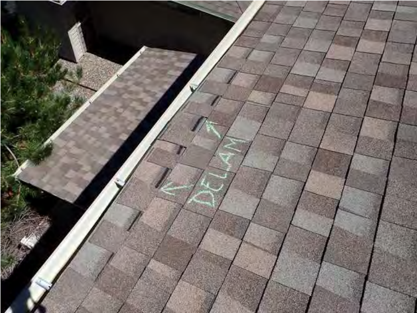
56. Building 3. Delamination.
