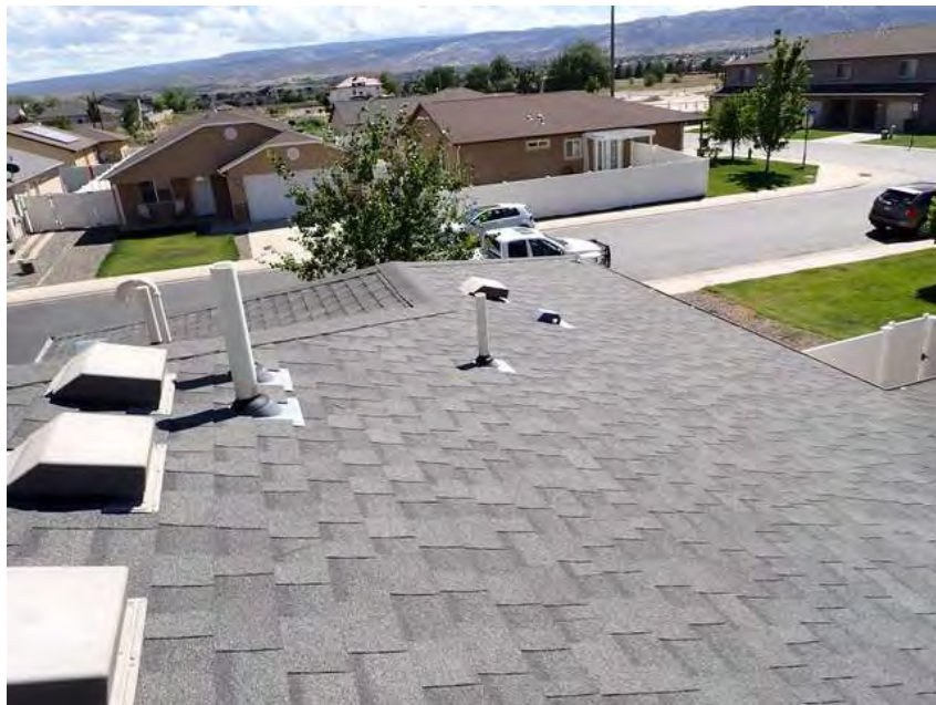
426. Building 24. Roof overview.
