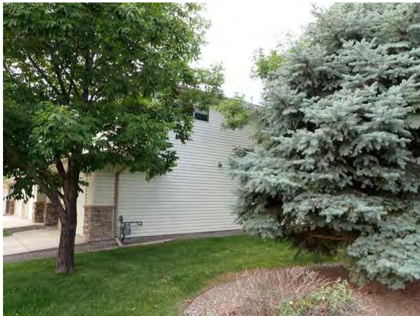
126. Building 7. Right overview.
