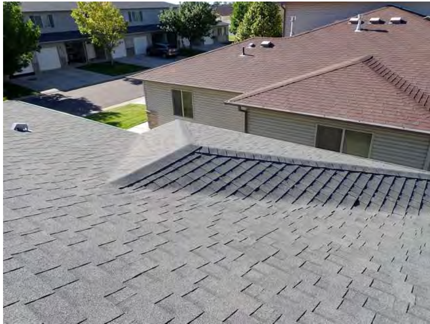
227. Building 13. Roof overview.
