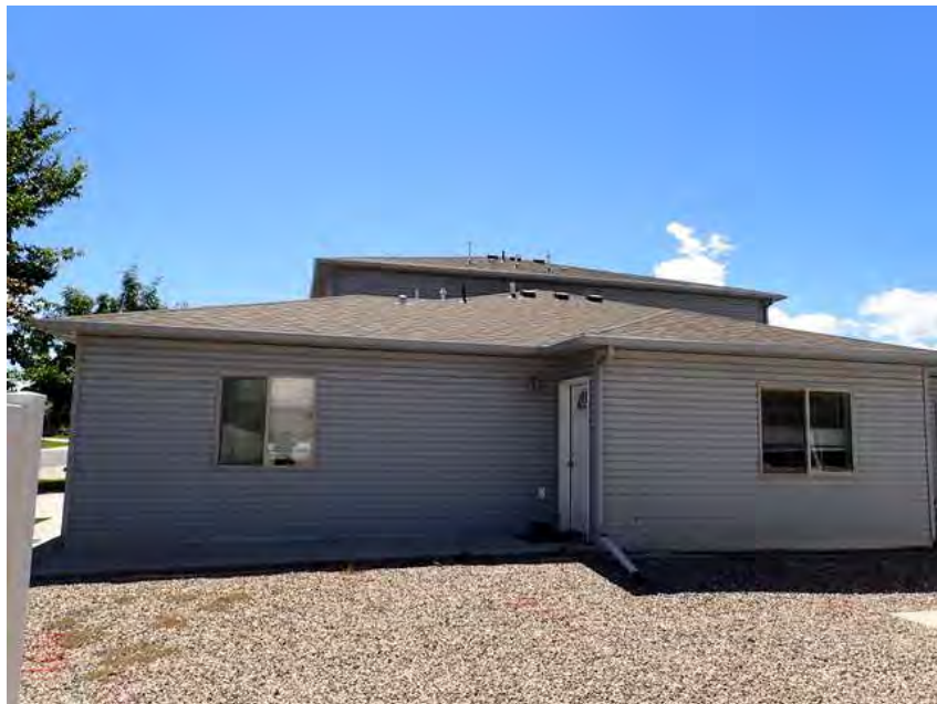
320. Building 19. Right overview.
