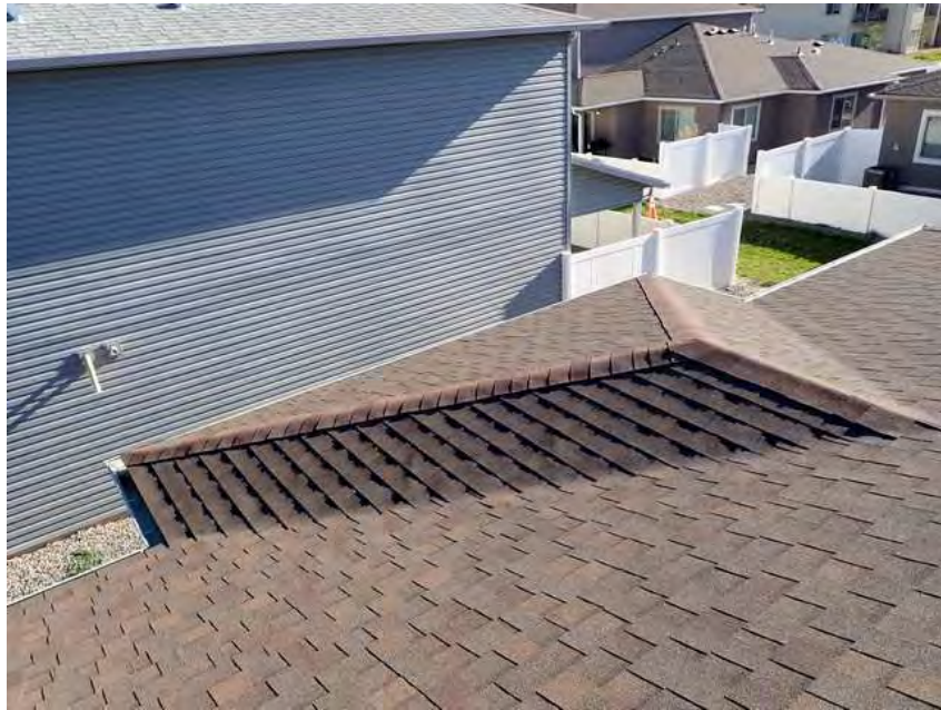
355. Building 21. Roof overview.
