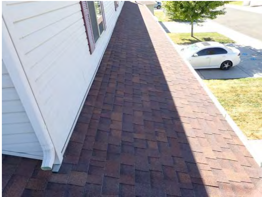
295. Building 17. Lower roof overview.
