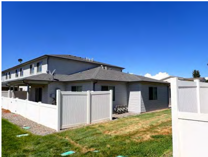
272. Building 16. Left overview.
