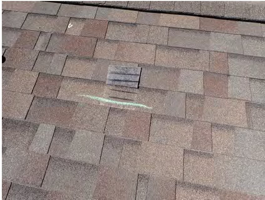
383. Building 22. Creased tooth on shingle.
