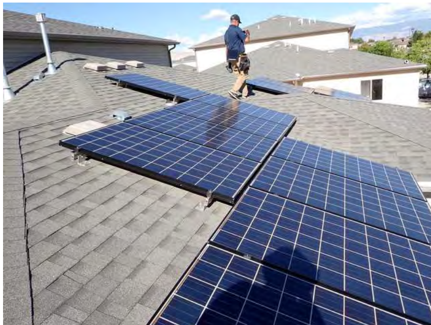
264. Building 15. Roof overview.
