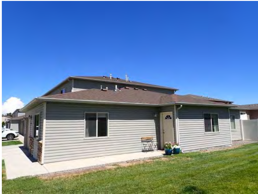
351. Building 21. Right overview.
