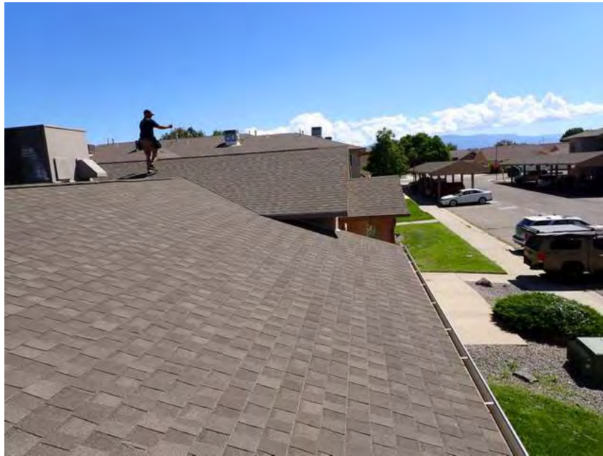
443. Club House. Roof overview.
