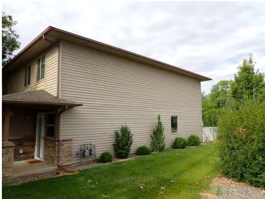
32. Building 2. Right overview.
