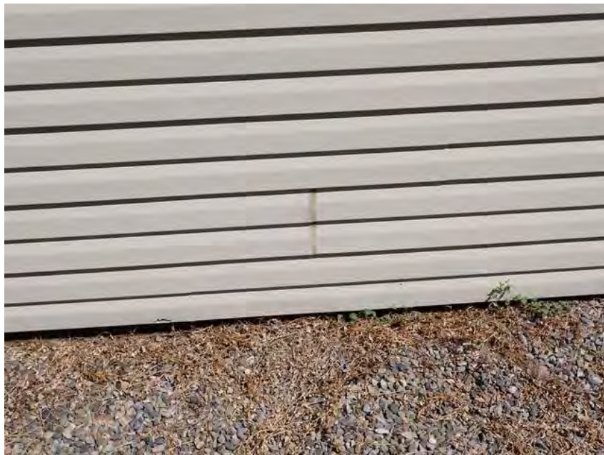
158. Building 9. Sealed gap in siding.
