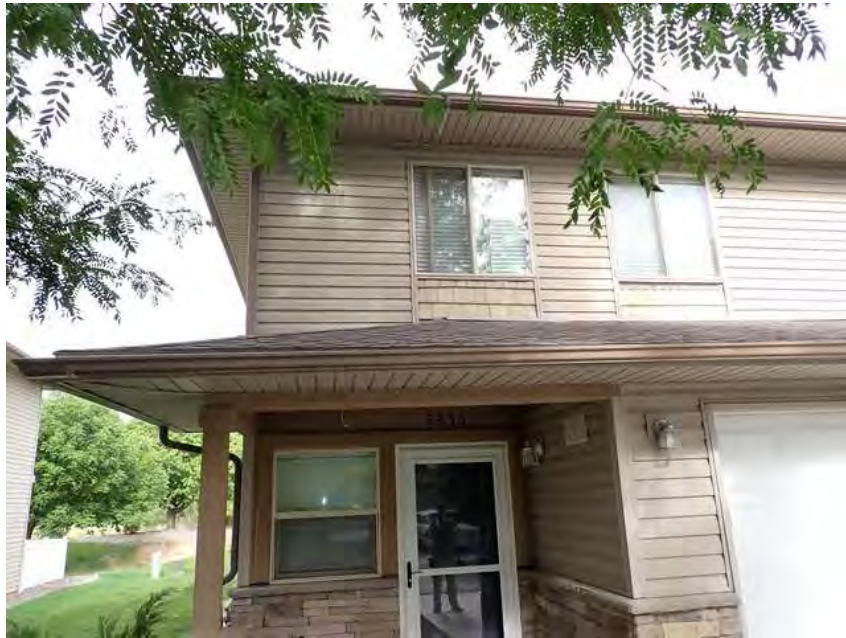
31. Building 2. Front overview.
