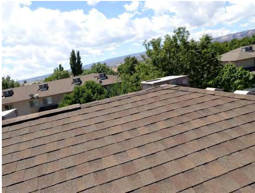
107. Building 6 Repair to ridge with cut shingles.
