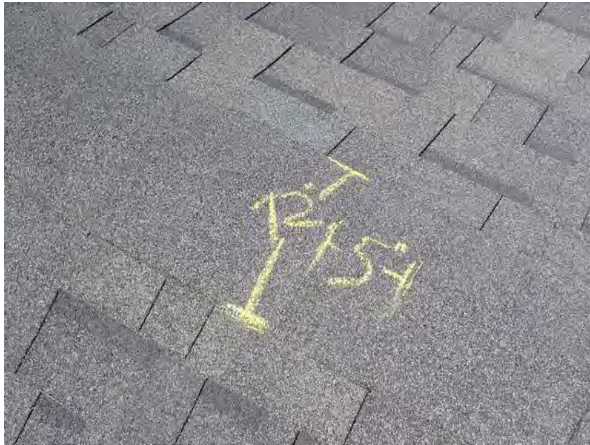
433. Building 24. Shingle dimensions.
