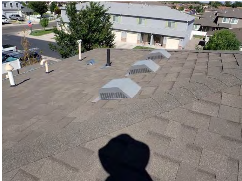
330. Building 19. Roof overview.
