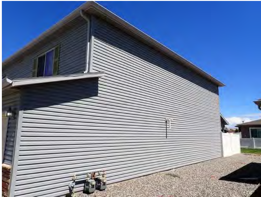
337. Building 20. Right overview.
