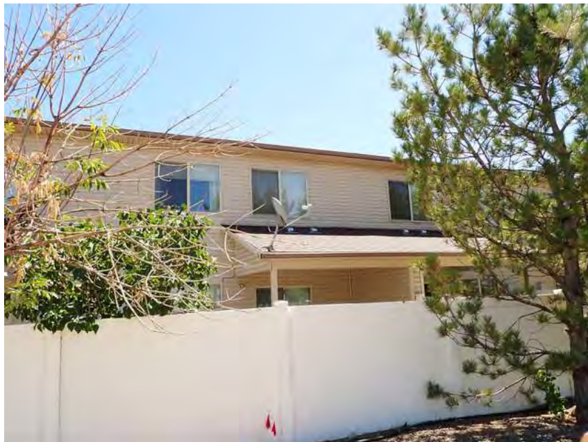
242. Building 14. Back overview.
