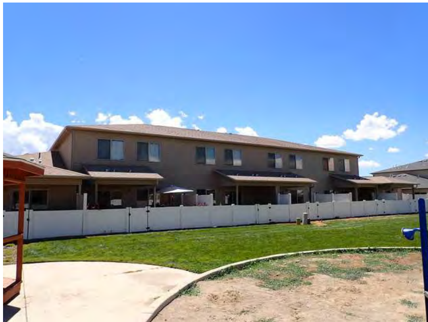
400. Building 23. Back overview.
