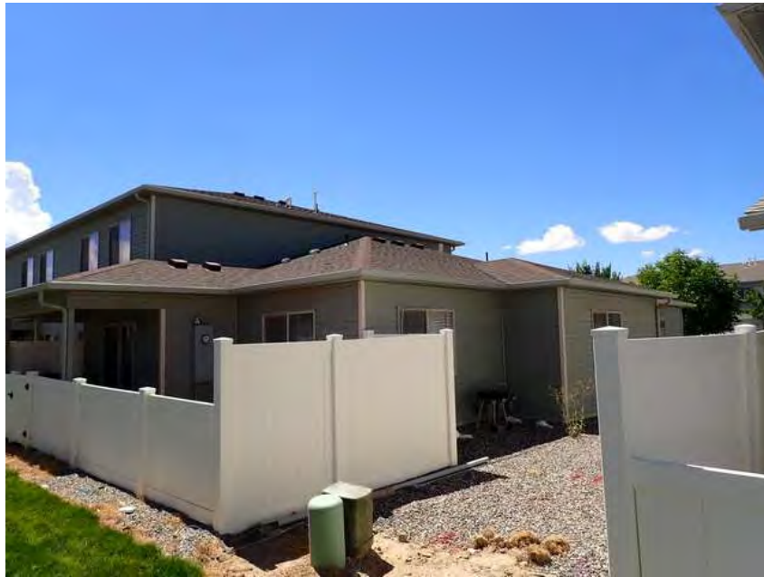
353. Building 21. Left overview.
