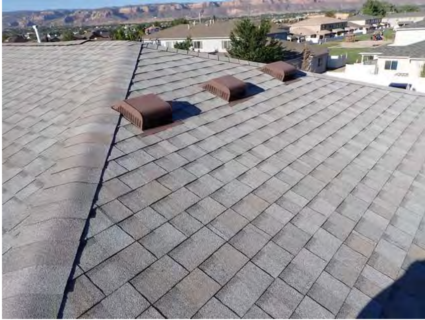
343. Building 20. Roof overview.
