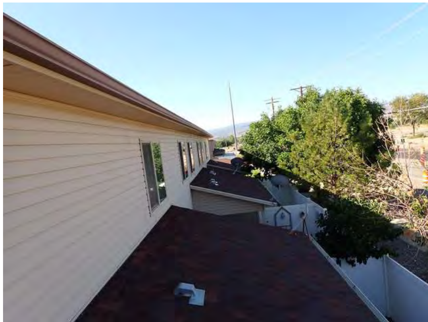
246. Building 14. Lower roof overview.
