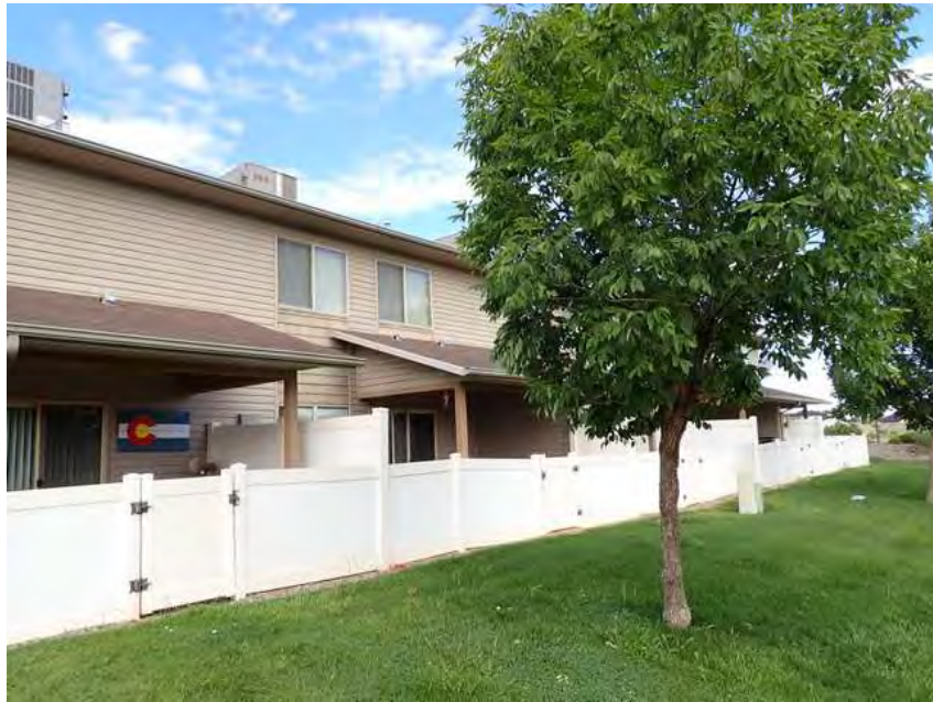
145. Building 8. Back overview.
