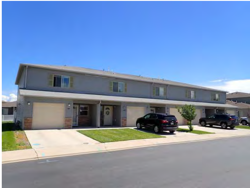
333. Building 20. Front overview.
