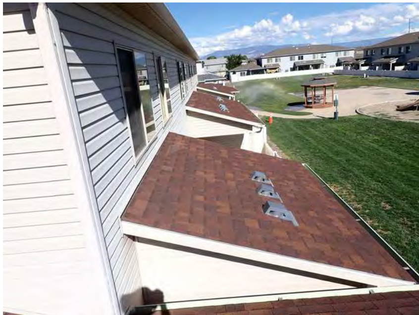
296. Building 17. Lower roof overview.
