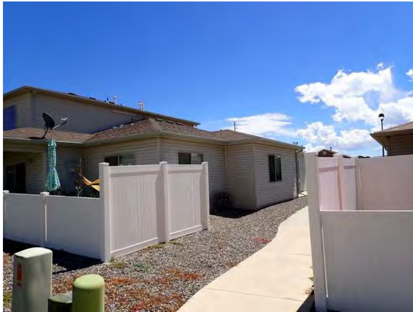
367. Building 22. Left overview.
