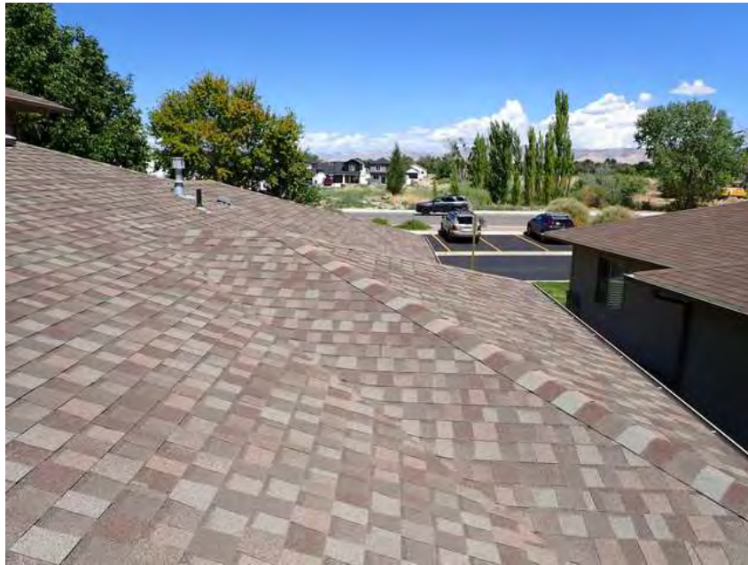
81. Building 5. Roof overview.
