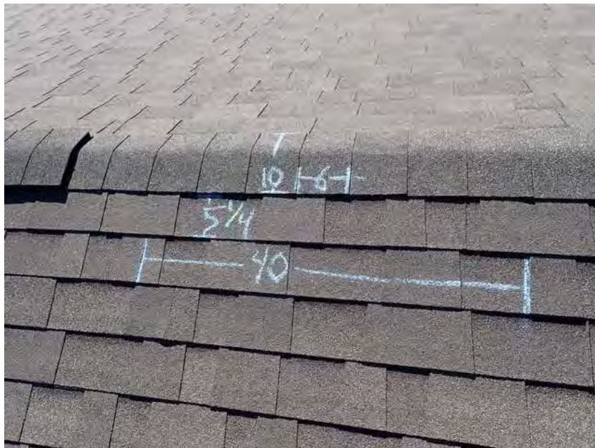
332. Building 19. Shingle dimensions.
