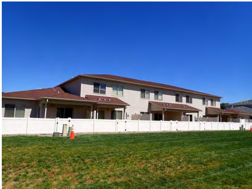
288. Building 17. Back overview.
