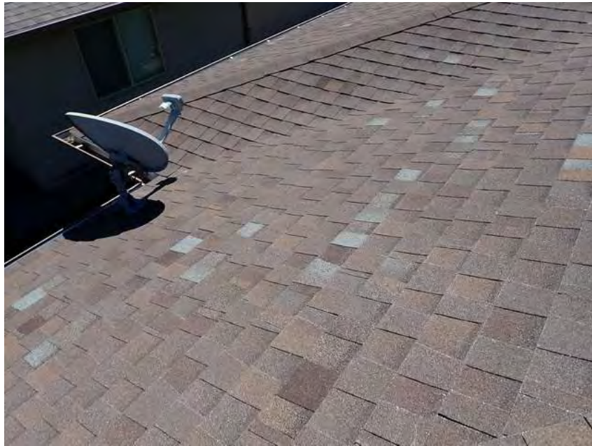
203. Building 12. Roof overview.
