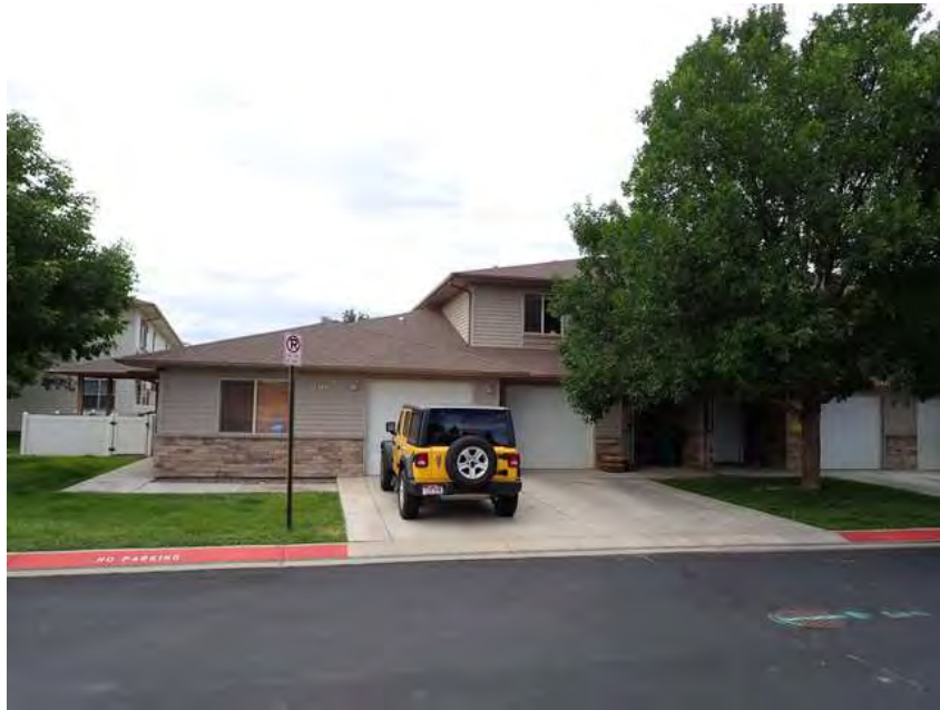
91. Building 6 Front overview.
