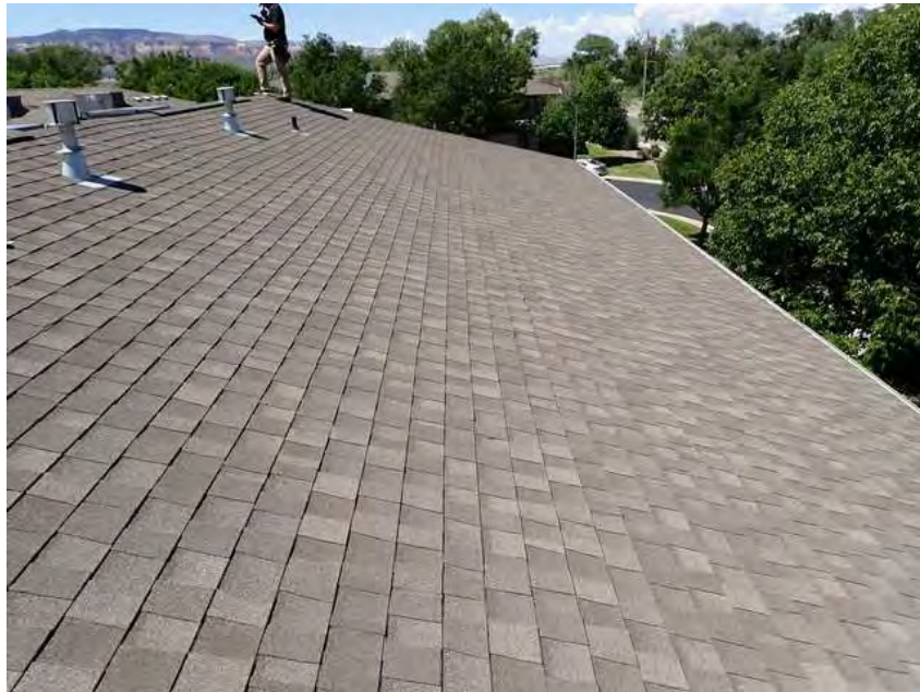
69. Building 4. Roof overview.
