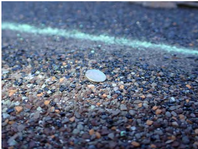
112. Building 6 Fasteners appear correctly installed.
