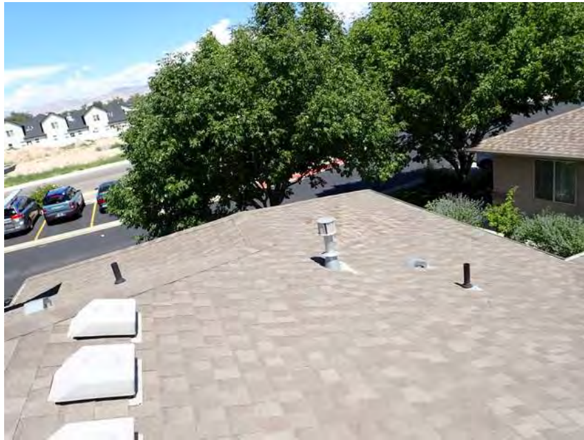
63. Building 4. Roof overview.
