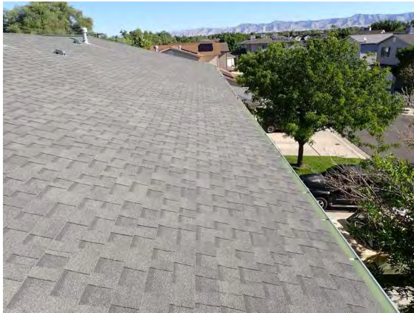
235. Building 13. Roof overview.
