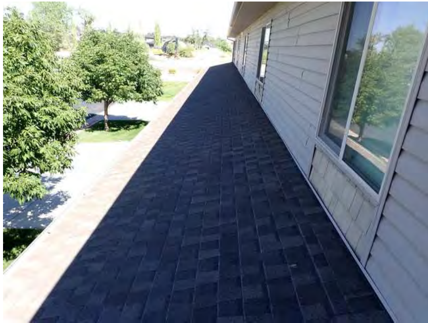
147. Building 8. Lower roof overview.
