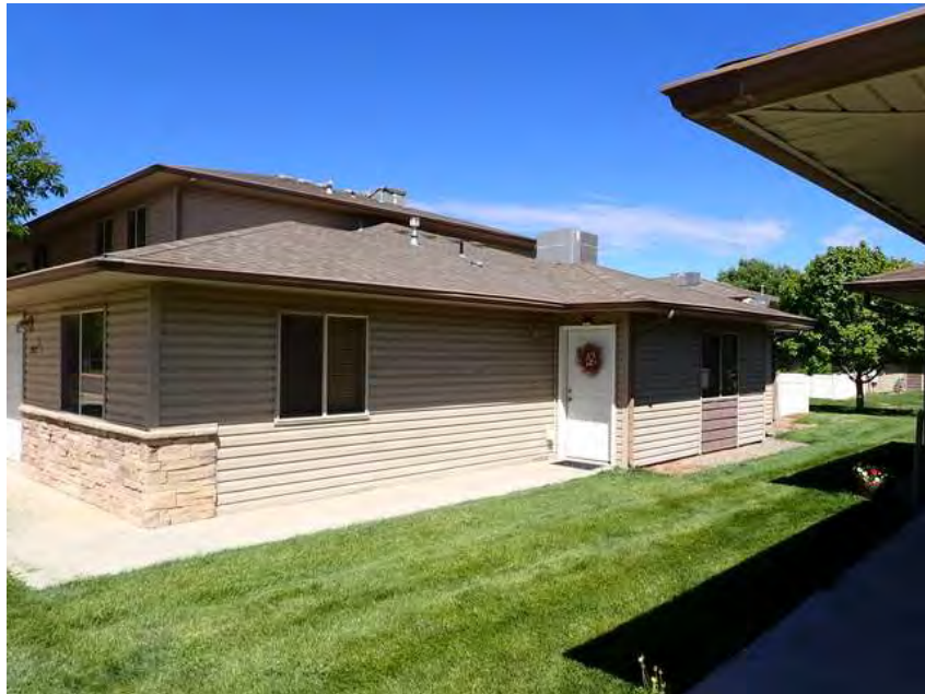
184. Building 11. Right overview.
