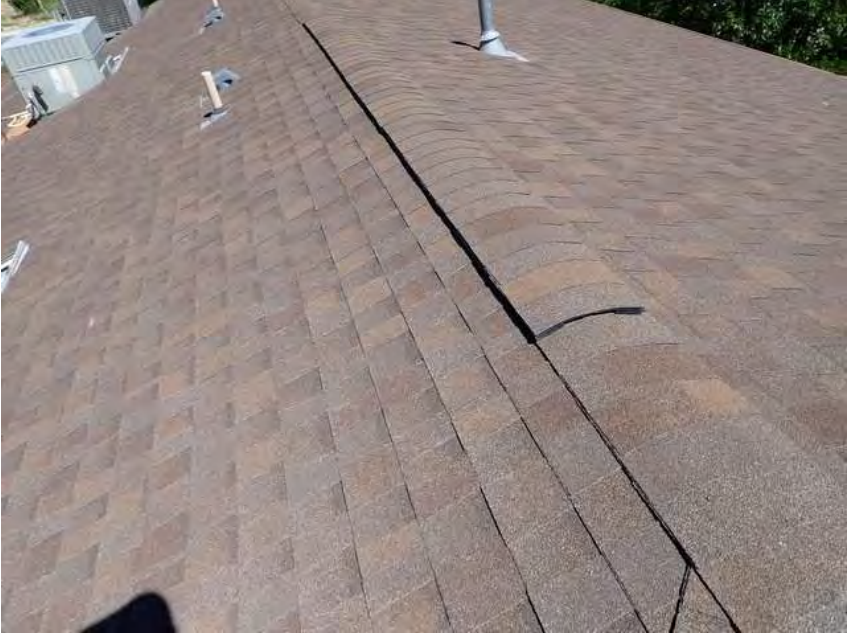
139. Building 7. Ridge overview.
