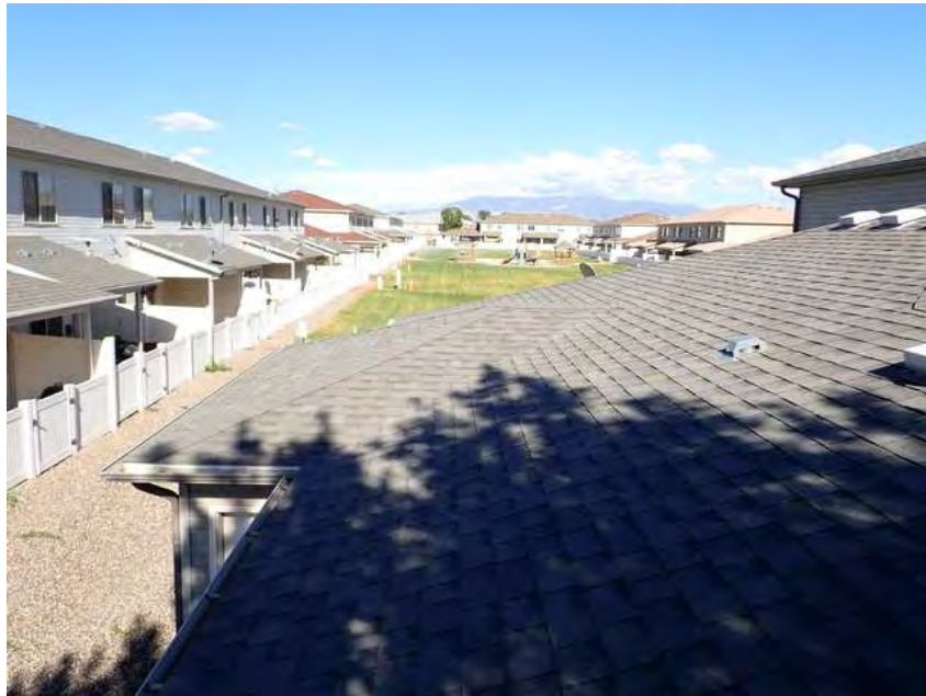
261. Building 15. Roof overview.
