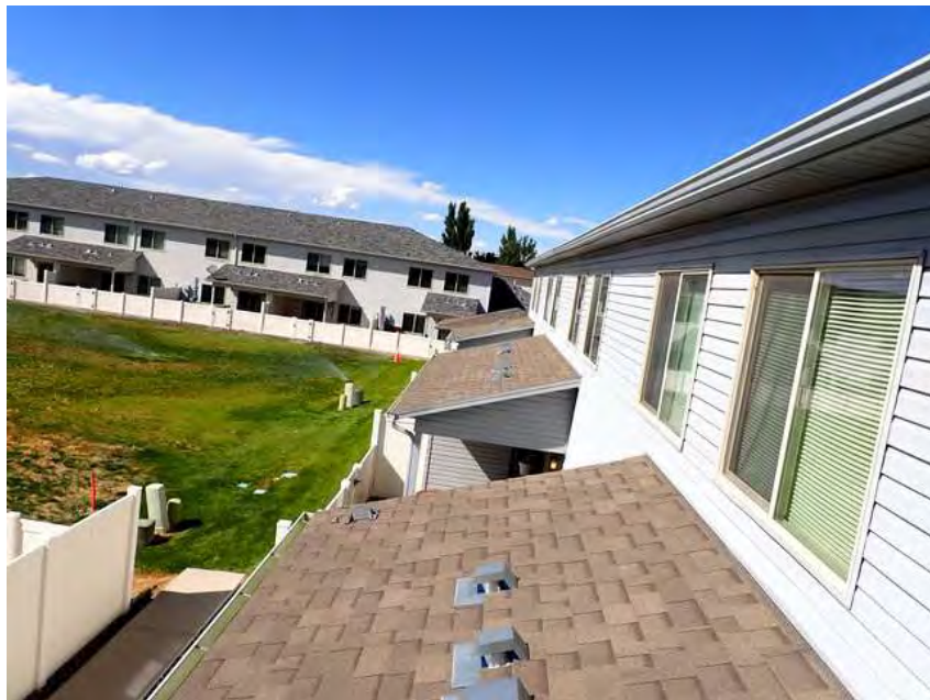
326. Building 19. Lower roof overview.
