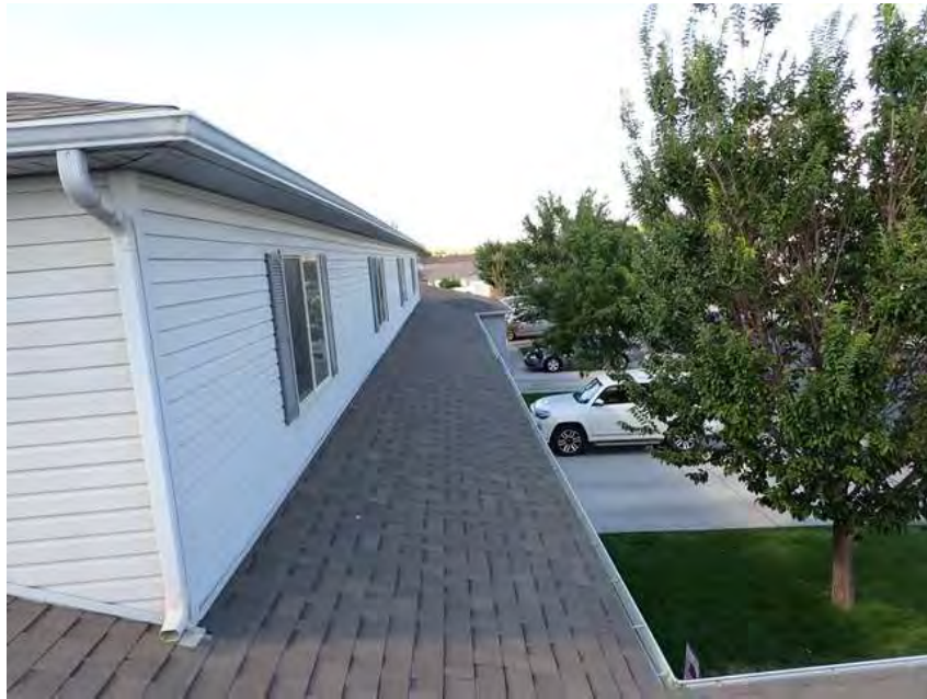
327. Building 19. Lower roof overview.
