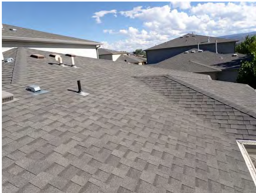
274. Building 16. Roof overview.
