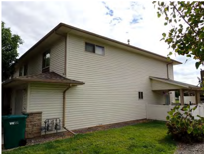
44. Building 3. Right overview.
