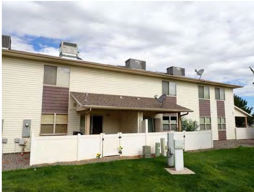
47. Building 3. Back overview.
