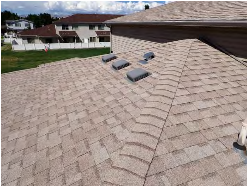
407. Building 23. Roof overview.
