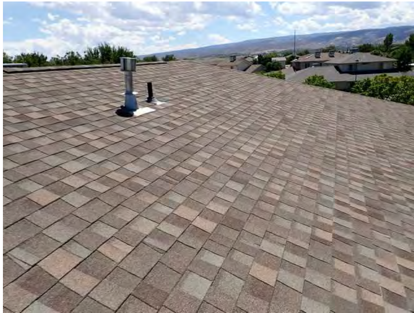
53. Building 3. Flue and plumbing stack.
