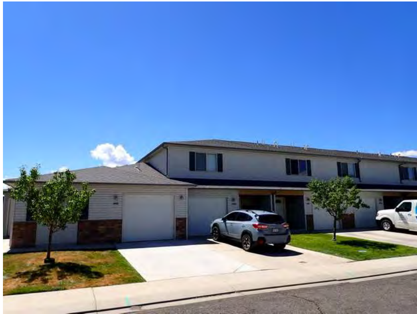
269. Building 16. Front overview.
