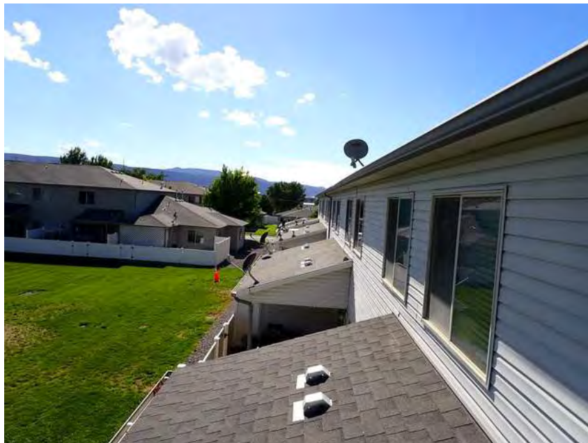
280. Building 16. Lower roof overview.
