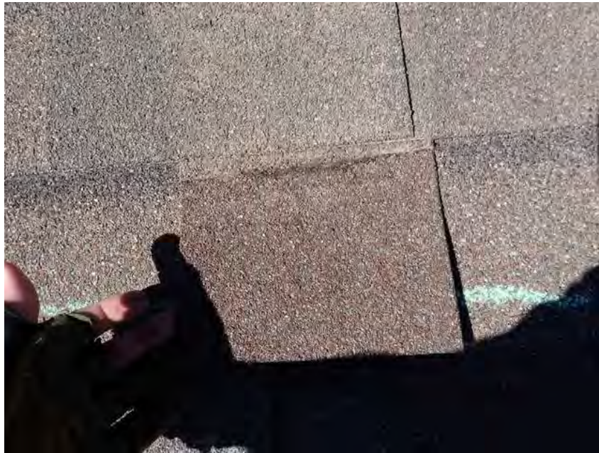
385. Building 22. Tooth back in place.
