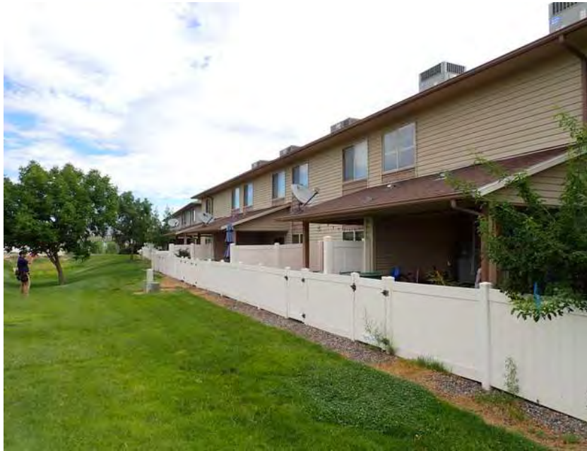
9. Building 1. Back overview.
