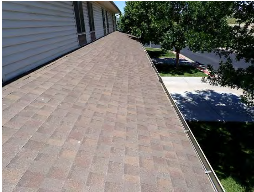
135. Building 7. Lower roof overview.
