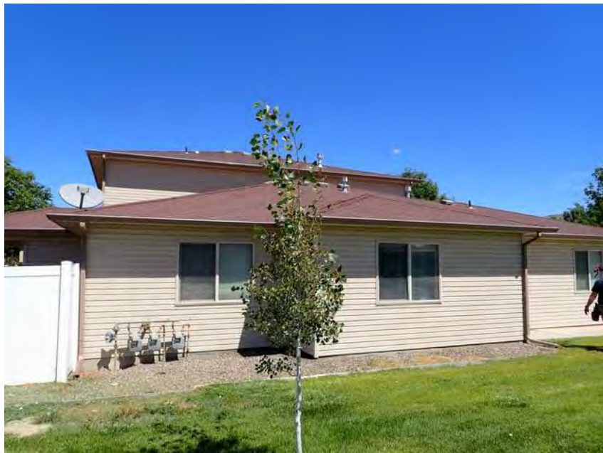
244. Building 14. Left overview.
