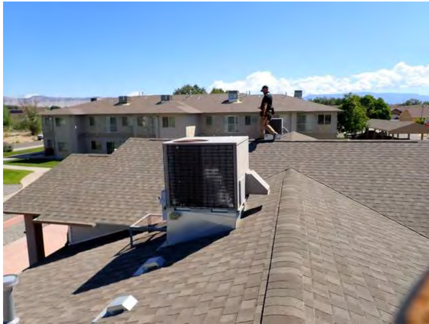
445. Club House. Roof overview.
