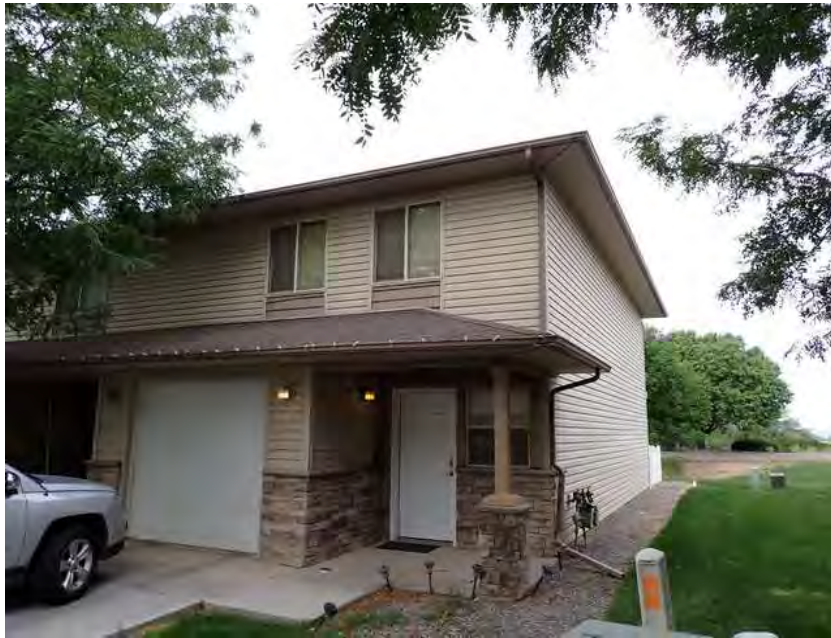
5. Building 1. Right overview.
