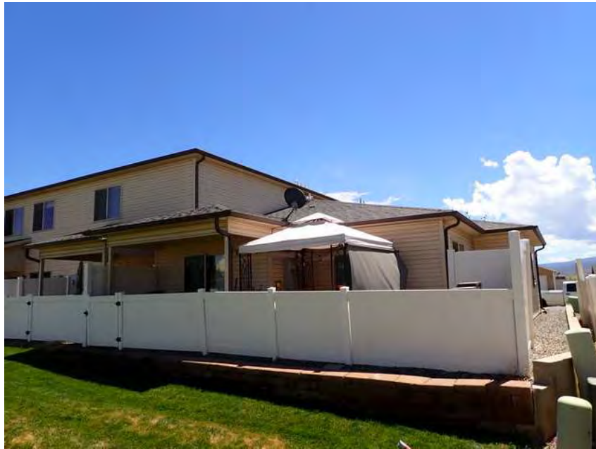
417. Building 24. Back overview.
