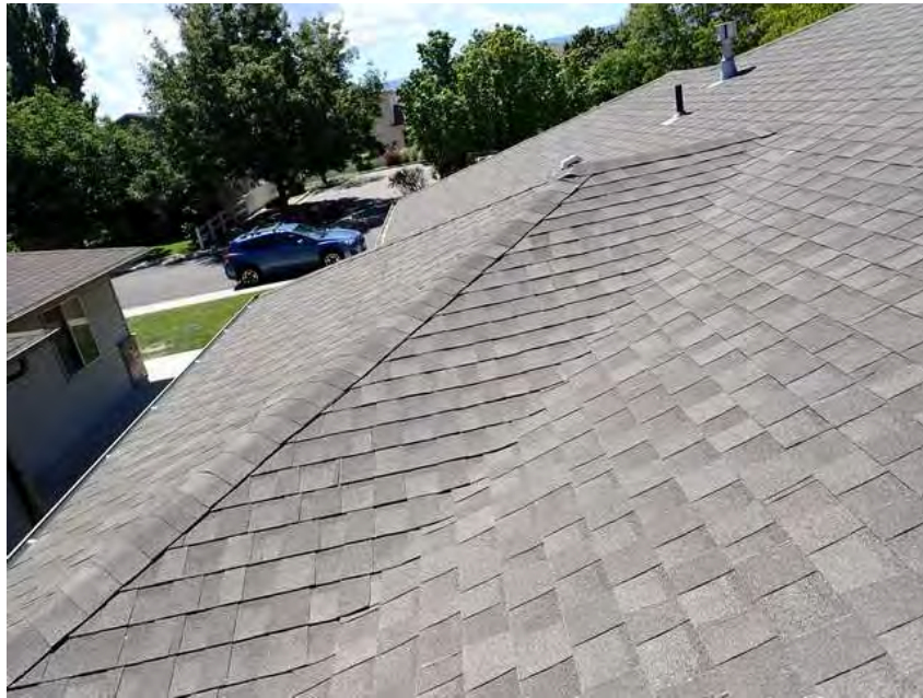
187. Building 11. Roof overview.
