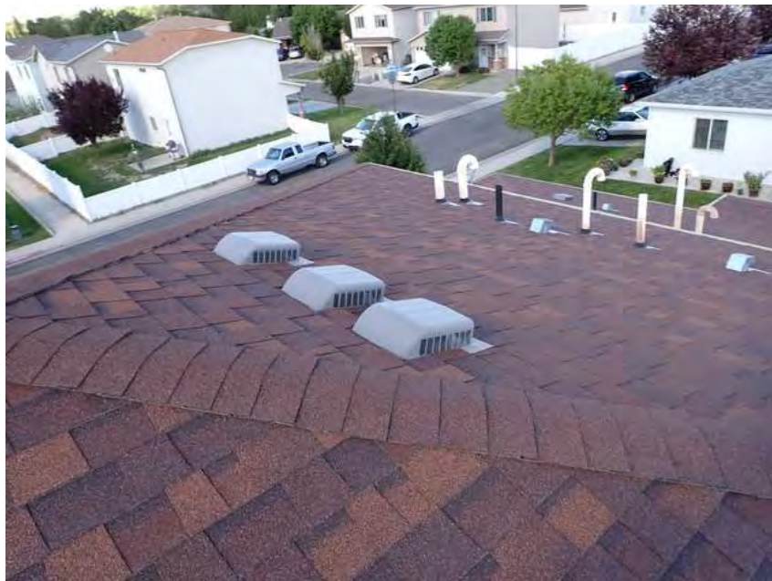
302. Building 17. Roof overview.
