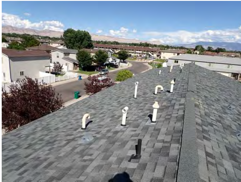
317. Building 18. Roof overview.
