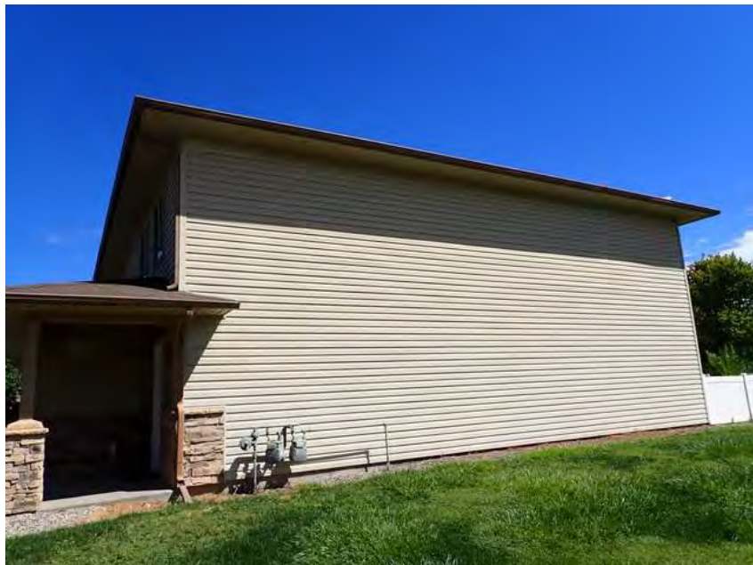
156. Building 9. Right overview.
