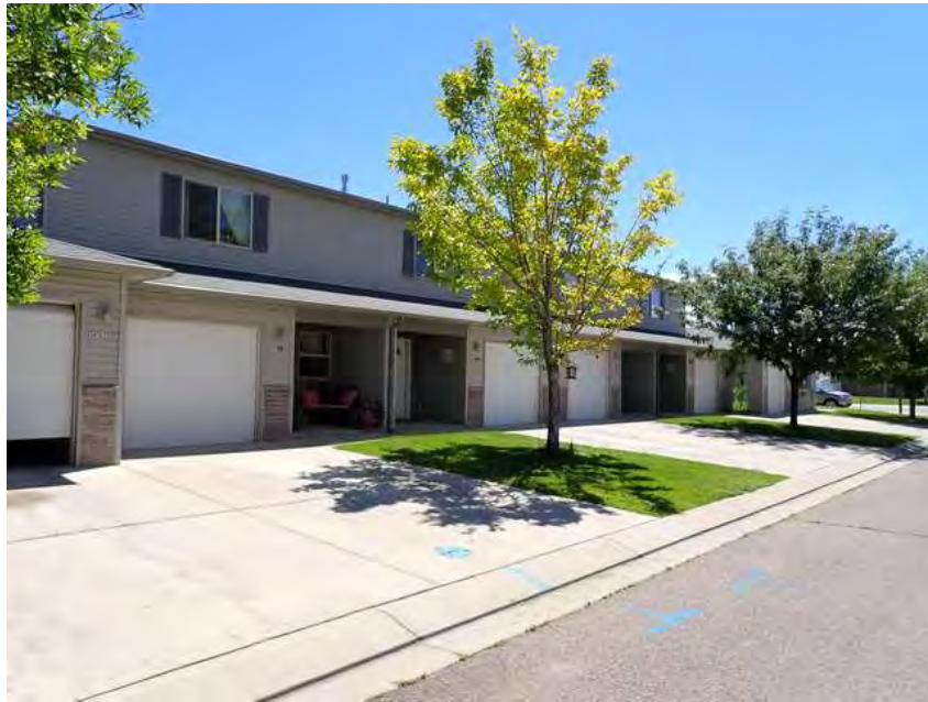
253. Building 15. Front overview.
