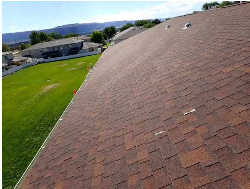
297. Building 17. Roof overview.
