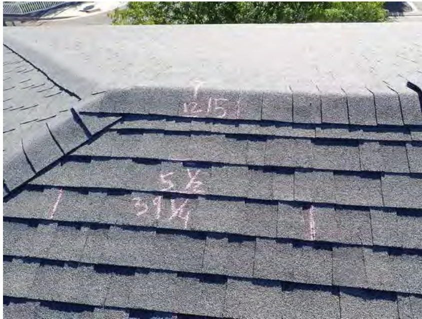
237. Building 13. Shingle dimensions.
