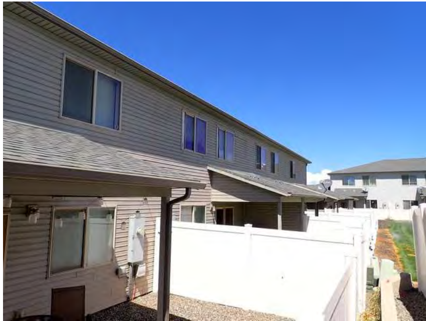
257. Building 15. Back overview.
