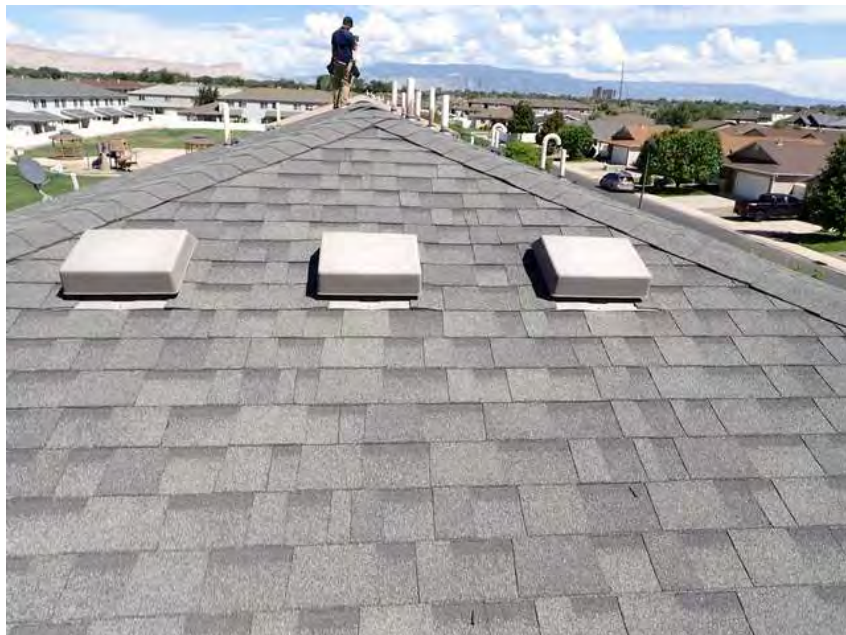
428. Building 24. Roof overview.
