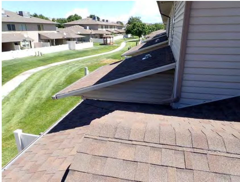
207. Building 12. Lower roof overview.
