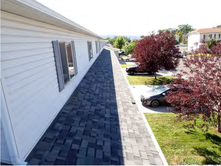
313. Building 18. Lower roof overview.
