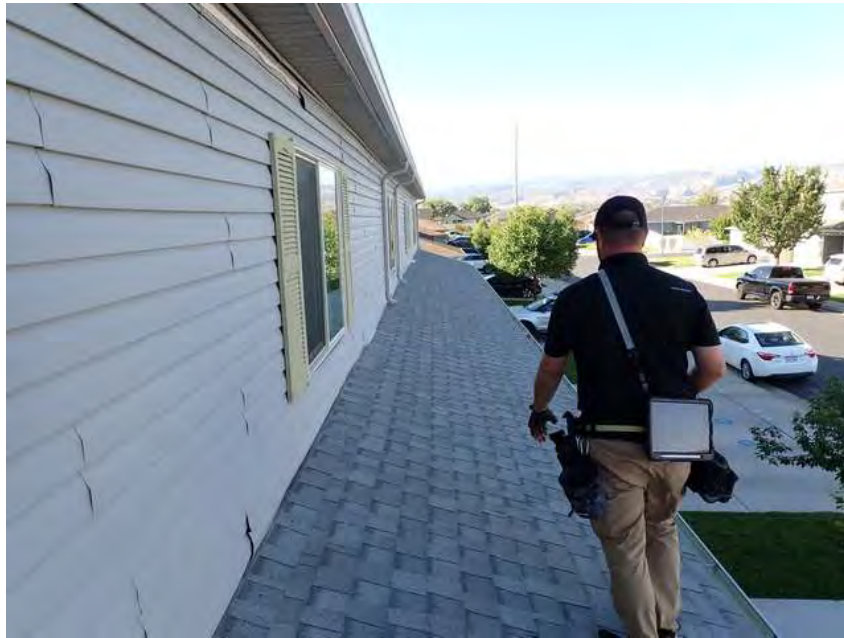
347. Building 20. Lower roof overview.
