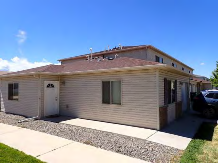
290. Building 17. Left overview.
