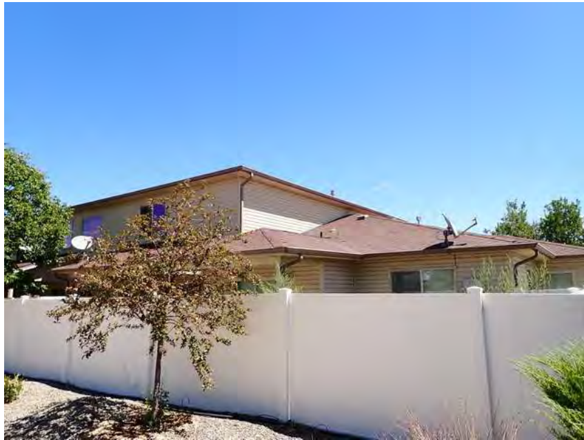
241. Building 14. Back overview.
