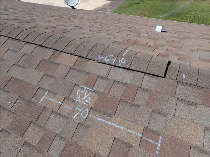
392. Building 22. Shingle dimensions.
