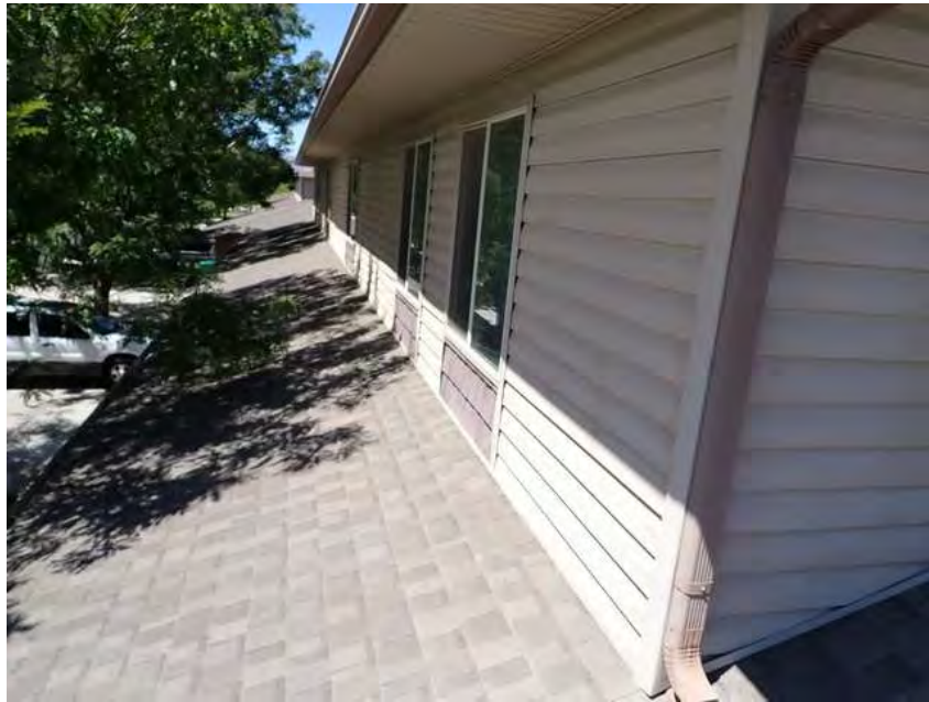
189. Building 11. Lower roof overview.
