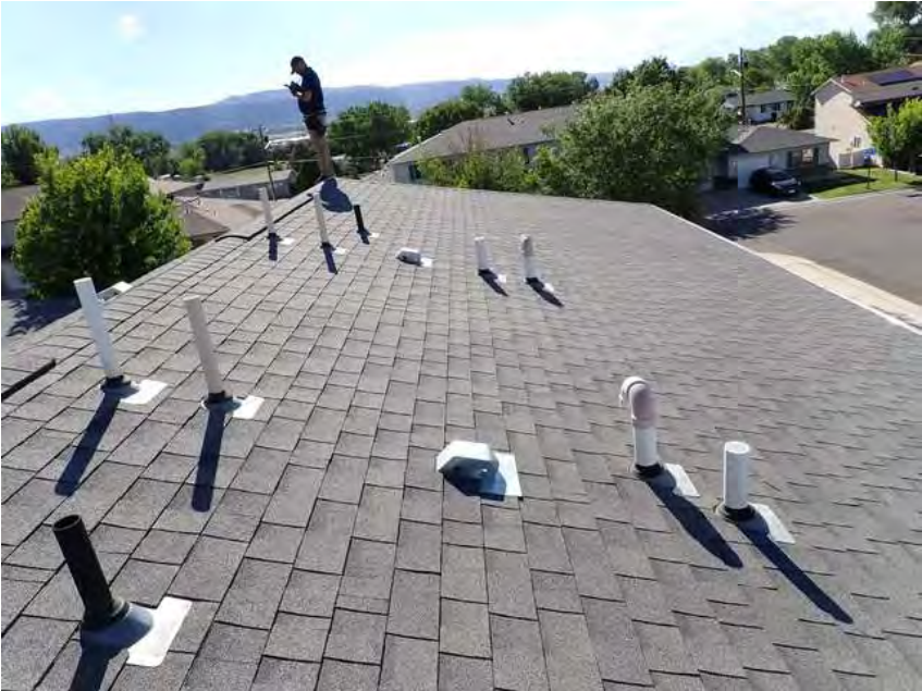
284. Building 16. Roof overview.
