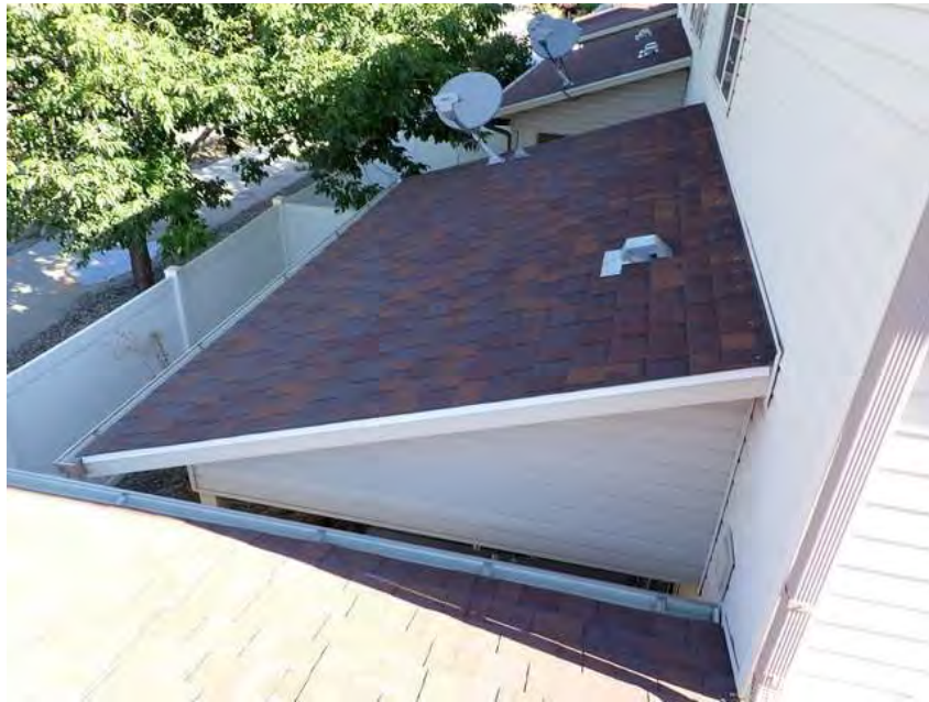
249. Building 14. Lower roof overview.
