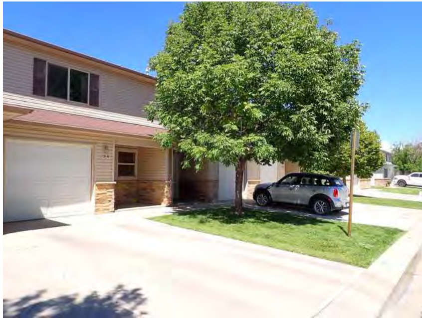
239. Building 14. Front overview.
