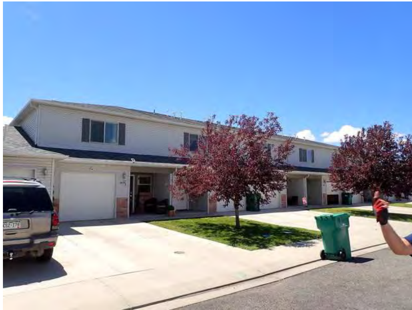
305. Building 18. Front overview.
