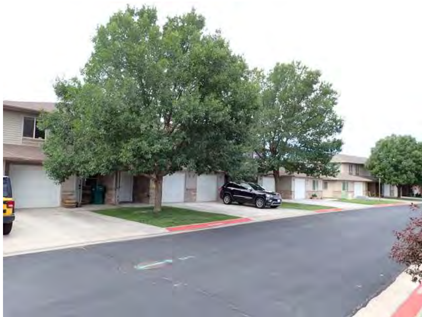
92. Building 6 Front overview.
