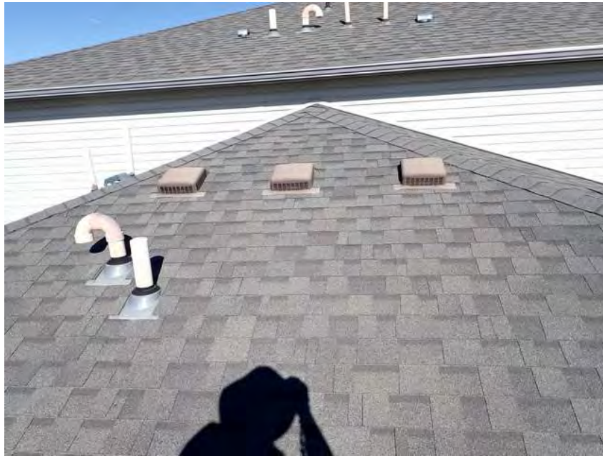
275. Building 16. Roof overview.
