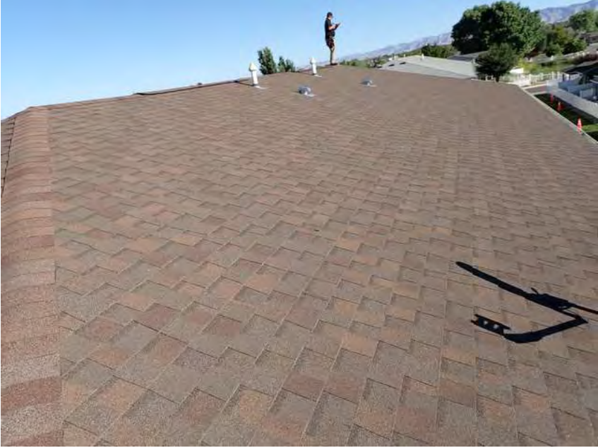
361. Building 21. Roof overview.
