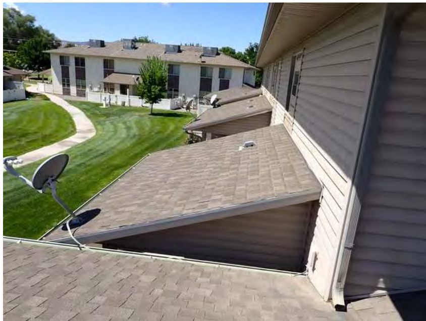
62. Building 4. Lower roof overview.
