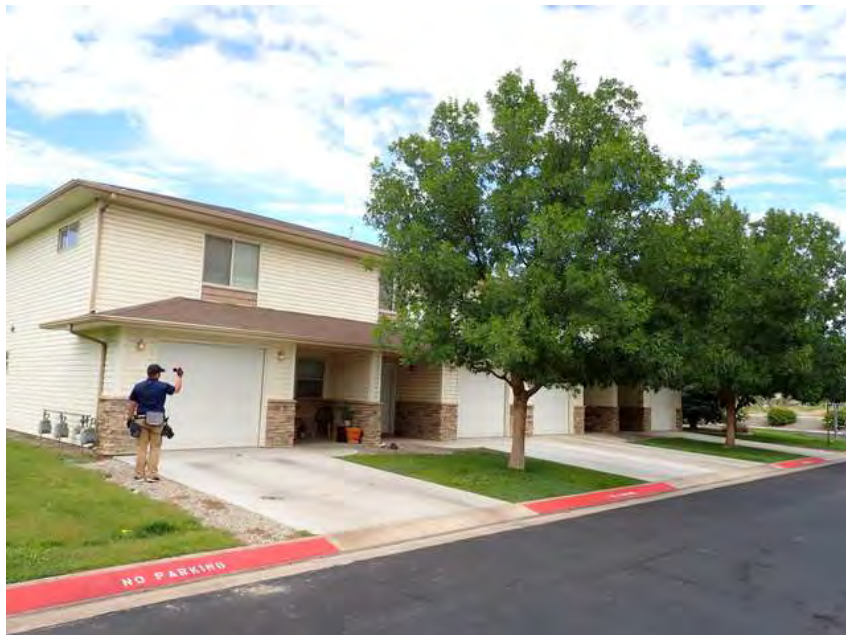
124. Building 7. Front overview.
