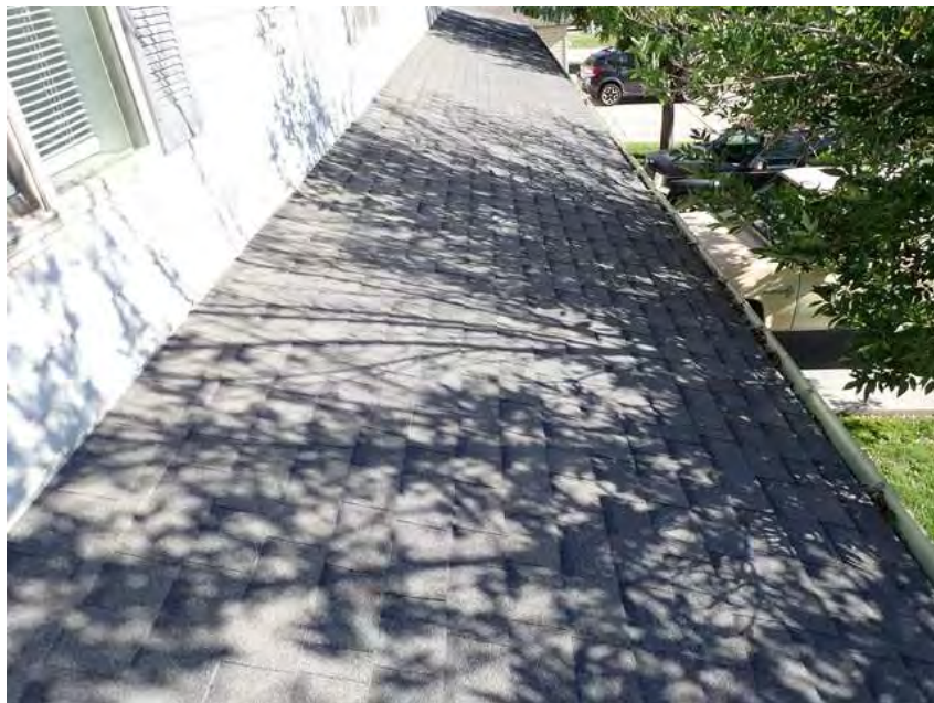
228. Building 13. Lower roof overview.
