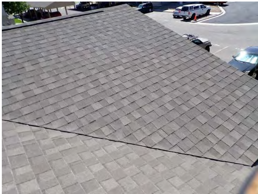
446. Club House. Roof overview.
