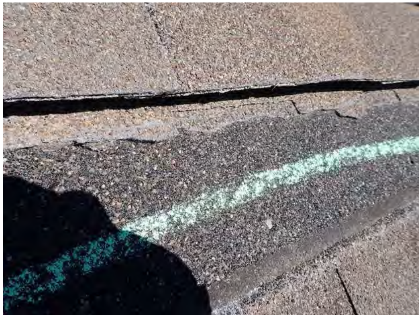
118. Building 6 Appears gray fibers at rip, suggesting an older crease resulting ultimately in a tear.
