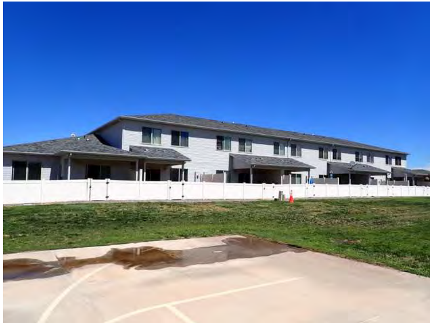
307. Building 18. Back overview.
