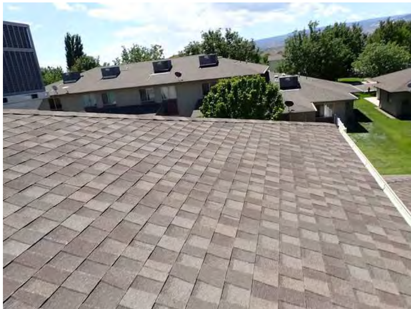
86. Building 5. Roof overview.
