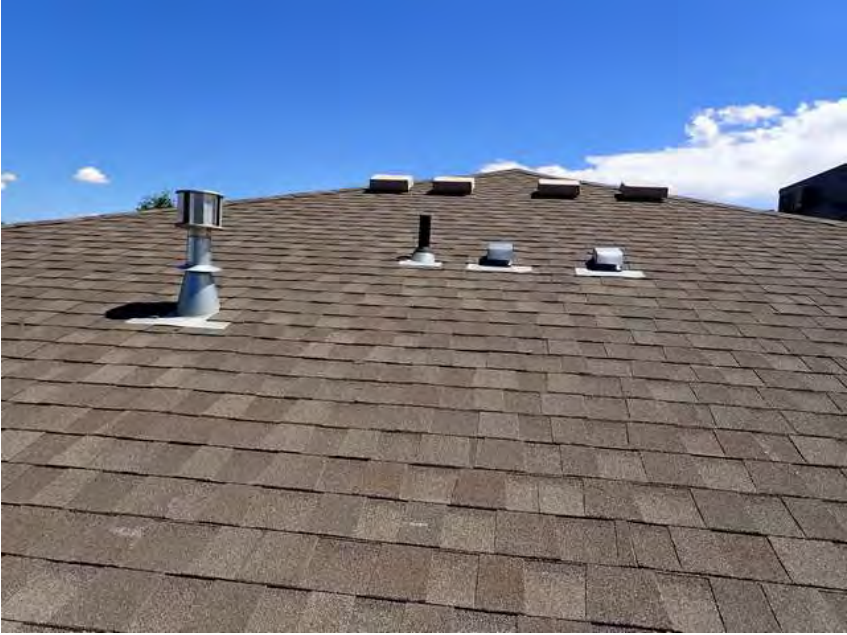
67. Building 4. Roof overview.
