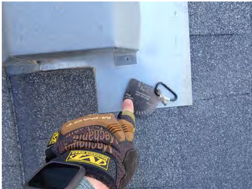
424. Building 24. Flashing made from steel.
