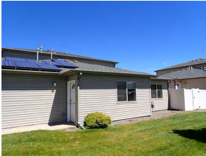
255. Building 15. Right overview.
