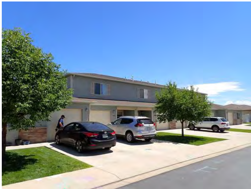
350. Building 21. Front overview.
