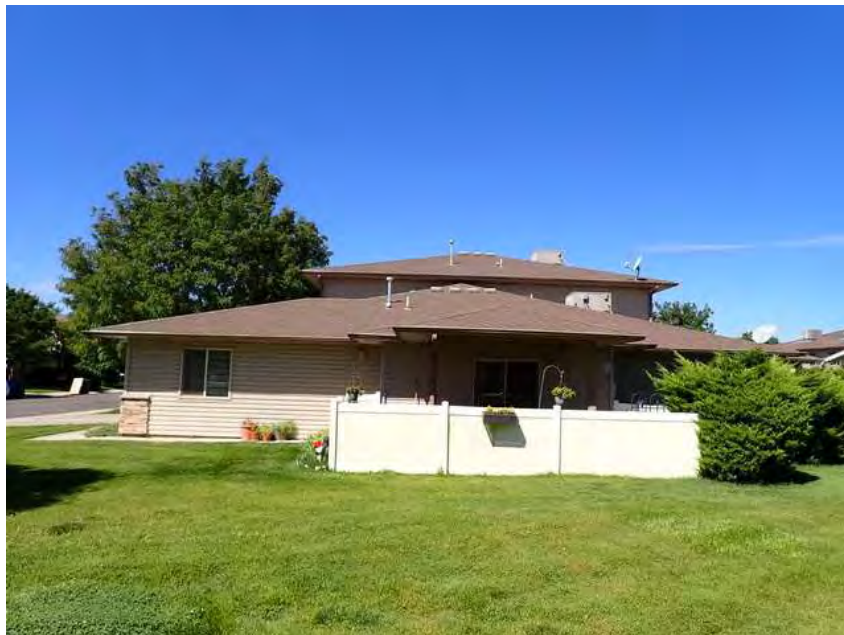
170. Building 10. Right overview.
