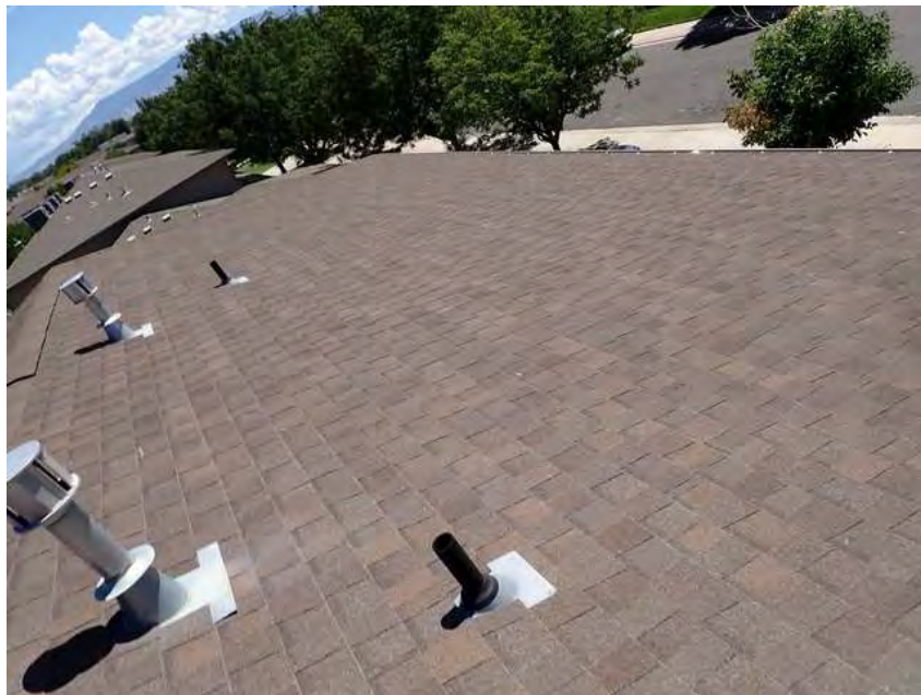
212. Building 12. Roof overview.
