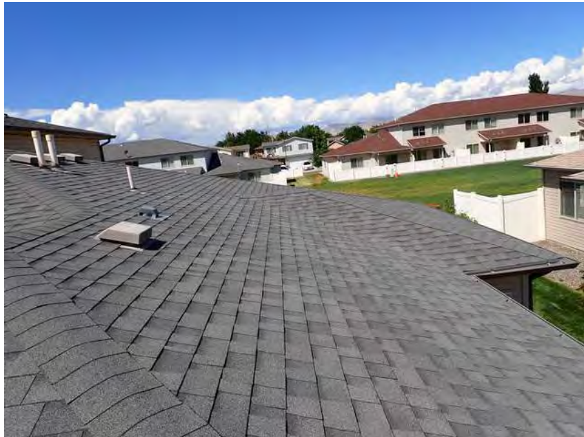
420. Building 24. Roof overview.
