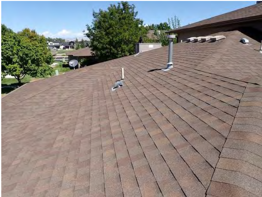
176. Building 10. Roof overview.
