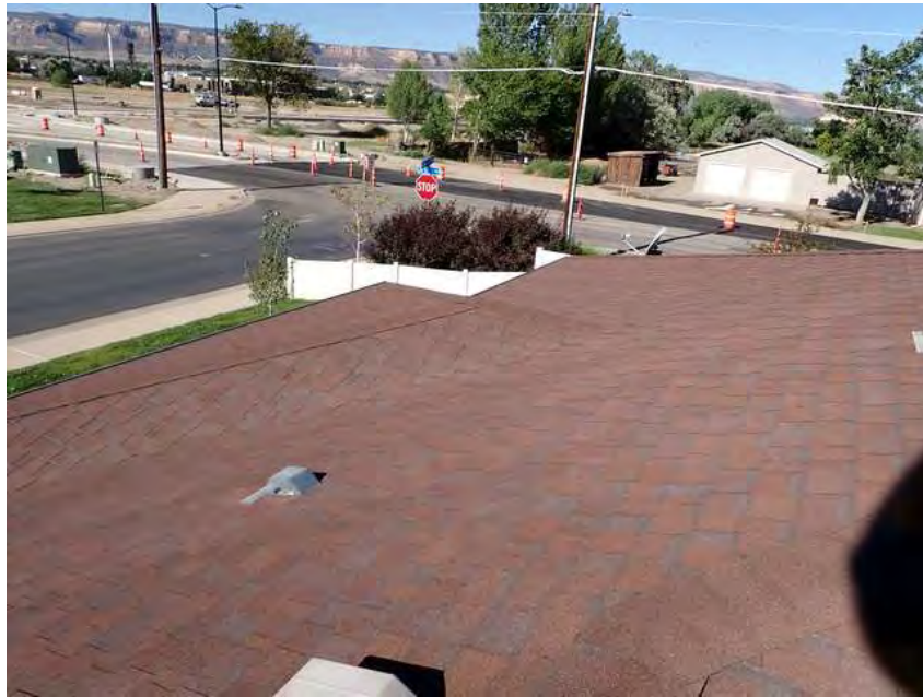
247. Building 14. Roof overview.
