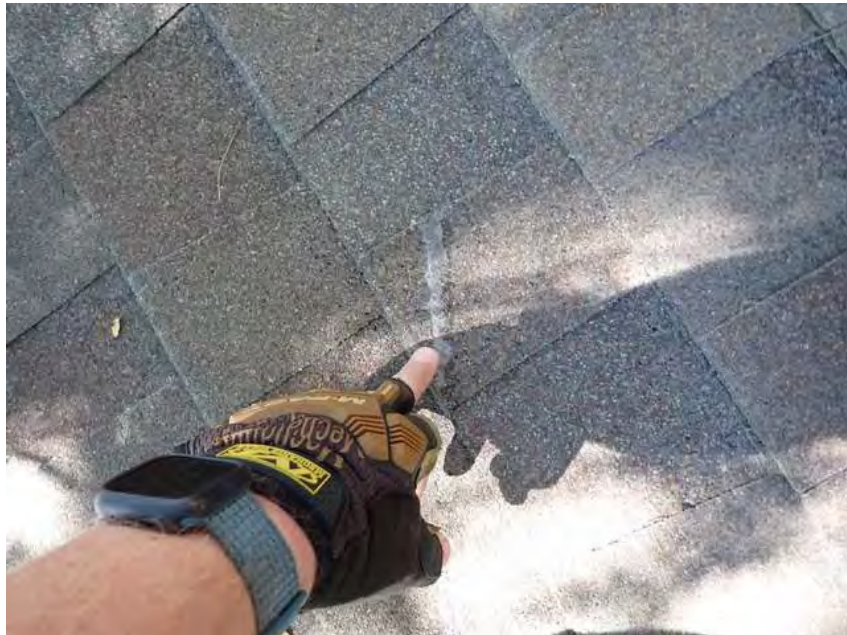
12. Building 1. Mar in granule coverage.
