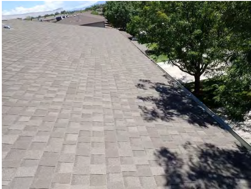
191. Building 11. Roof overview.
