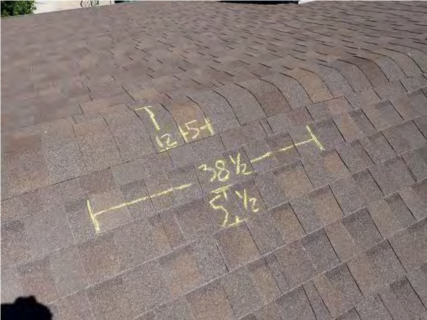
180. Building 10. Shingle dimensions.
