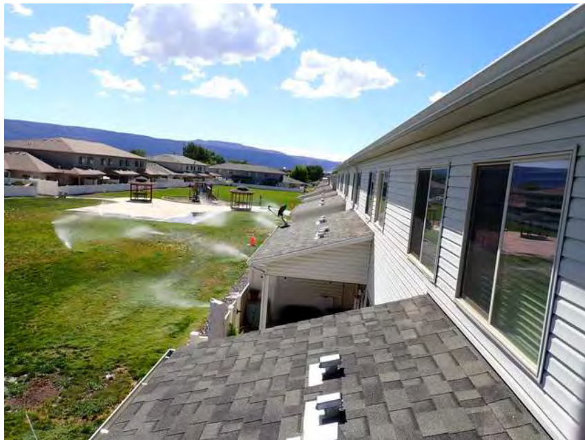
312. Building 18. Lower roof overview.
