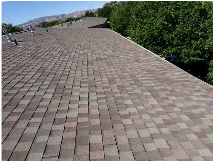
87. Building 5. Roof overview.
