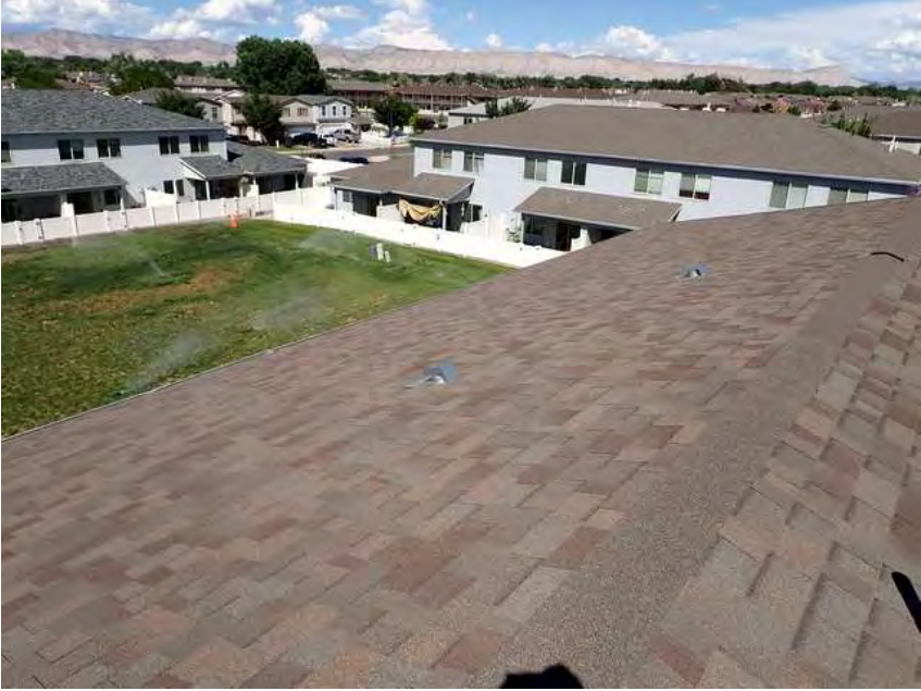
391. Building 22. Roof overview.
