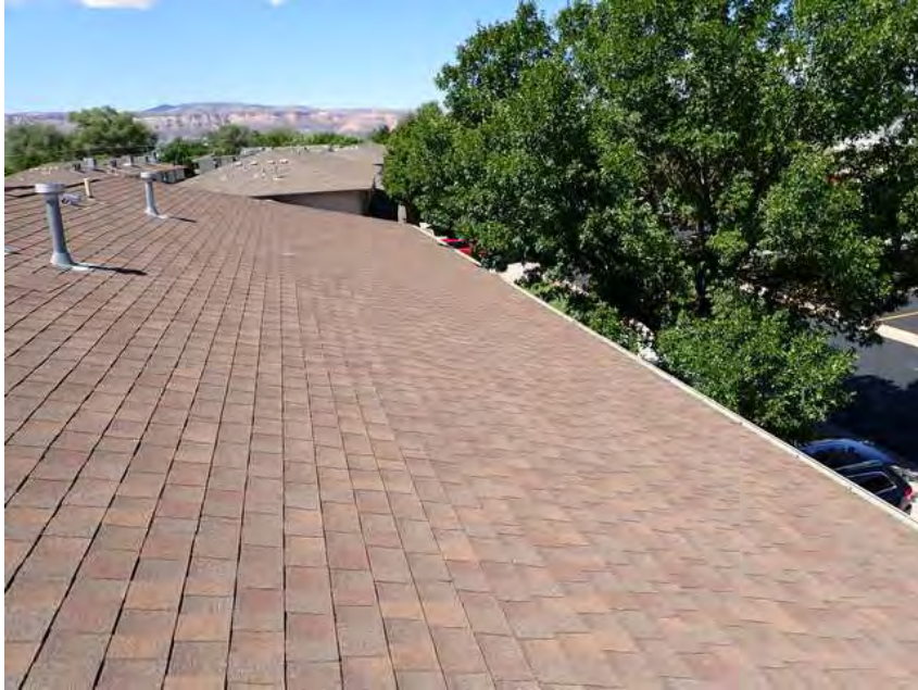
103. Building 6 Roof overview.
