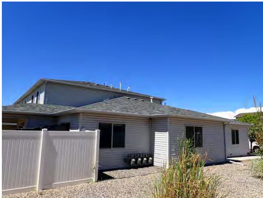
308. Building 18. Left overview.
