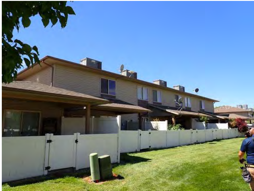
185. Building 11. Back overview.
