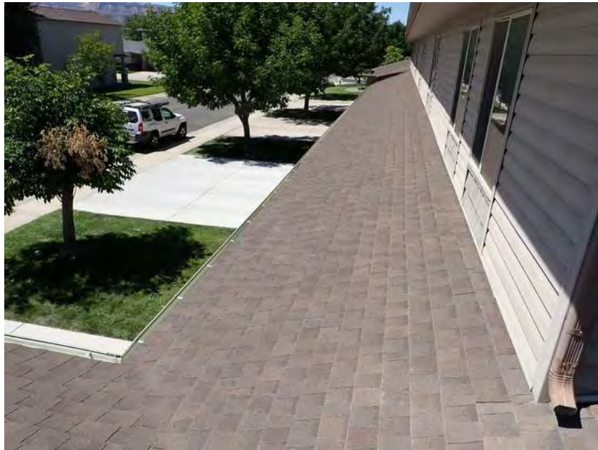
205. Building 12. Lower roof overview.
