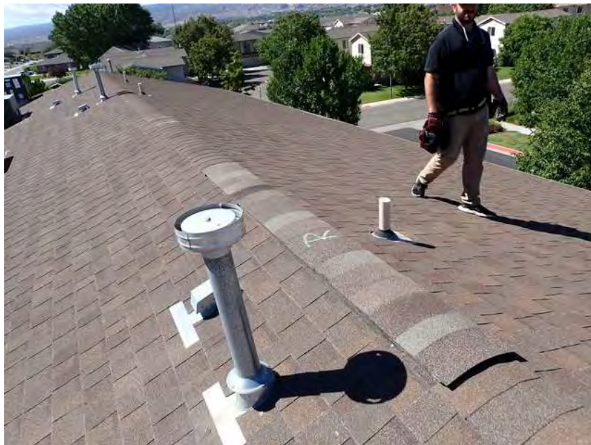
166. Building 9. Ridge cap repair.
