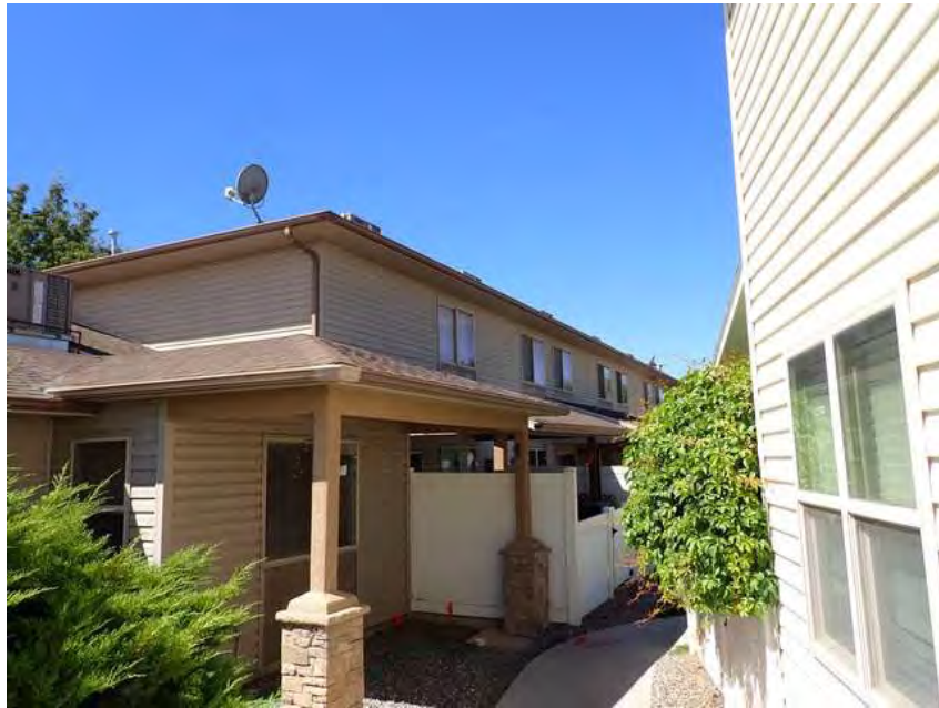
171. Building 10. Back overview.
