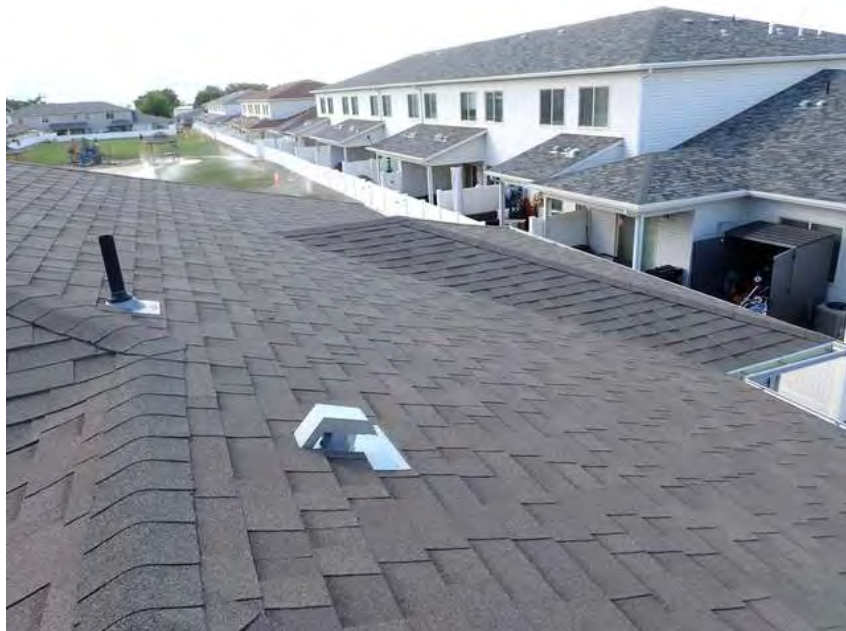
328. Building 19. Roof overview.
