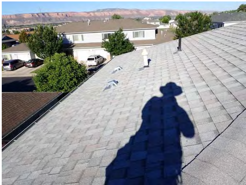
340. Building 20. Roof overview.
