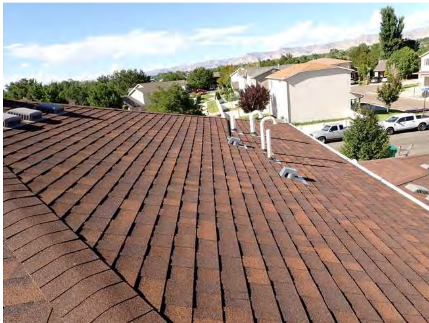
298. Building 17. Roof overview.
