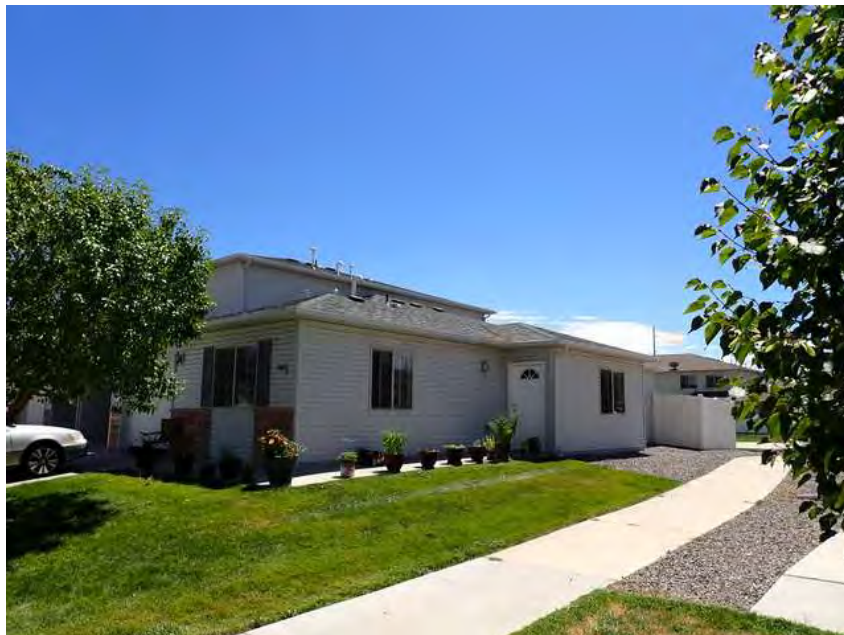
306. Building 18. Right overview.
