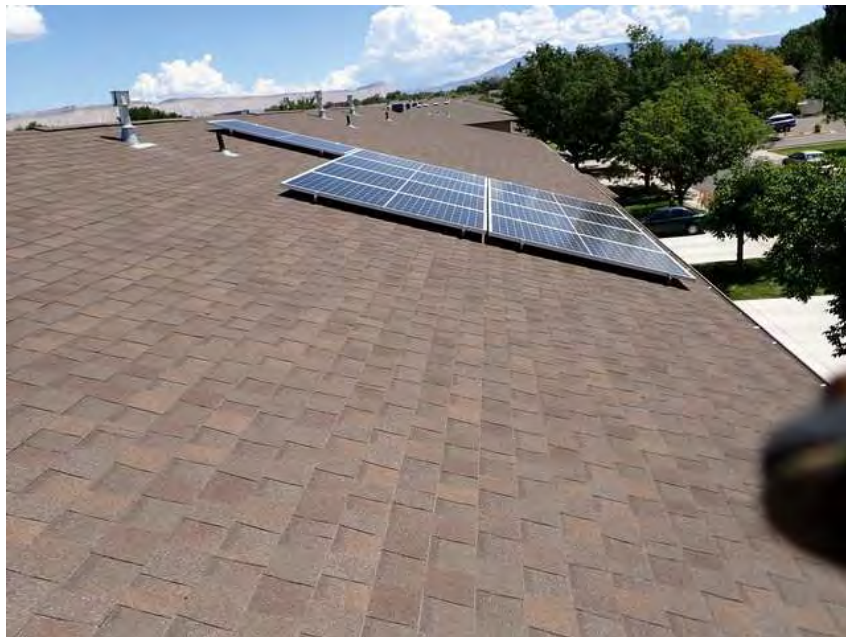
210. Building 12. Roof overview.
