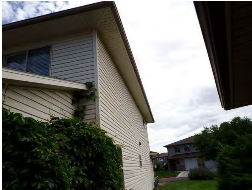
129. Building 7. Left overview.
