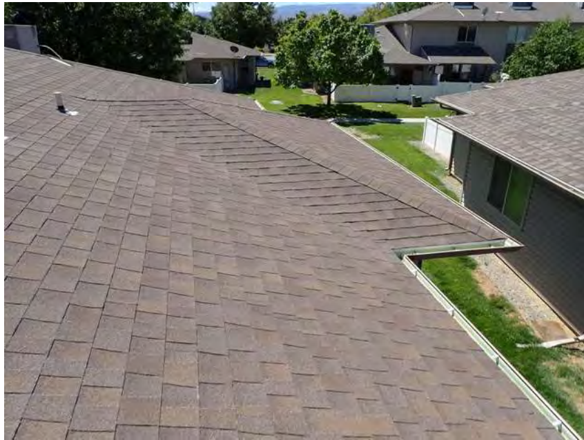
101. Building 6 Roof overview.
