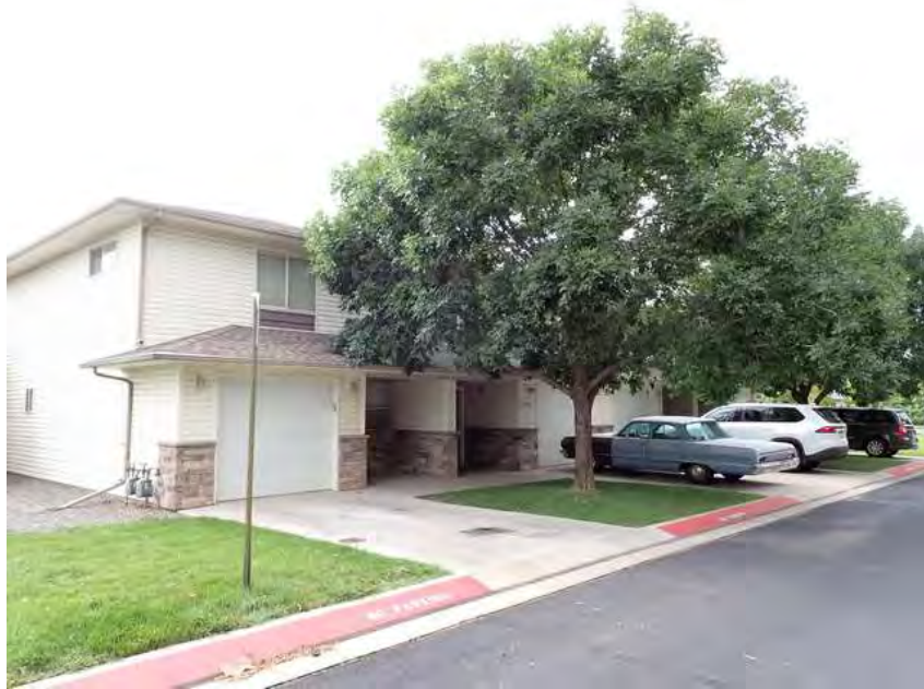
43. Building 3. Front overview.
