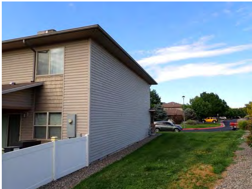
146. Building 8. Left overview.
