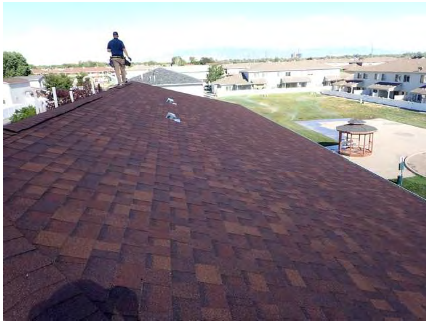
301. Building 17. Roof overview.
