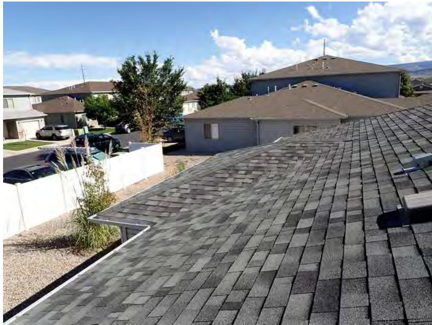
309. Building 18. Roof overview.
