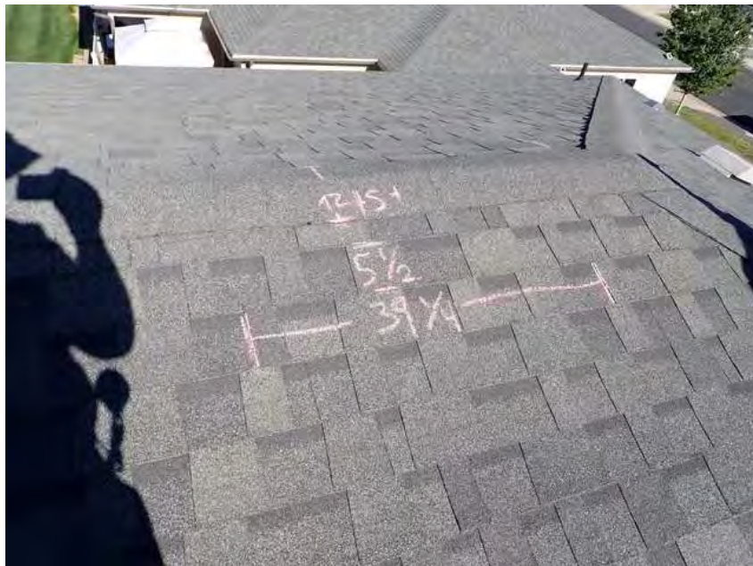
268. Building 15. Shingle dimensions.
