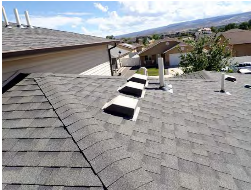
425. Building 24. Roof overview.
