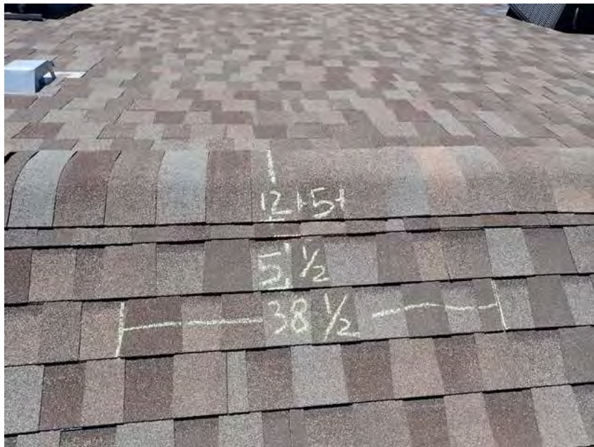
90. Building 5. Shingle dimensions.
