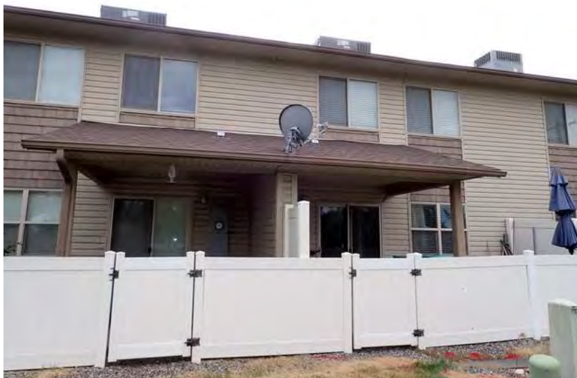
8. Building 1. Back overview.
