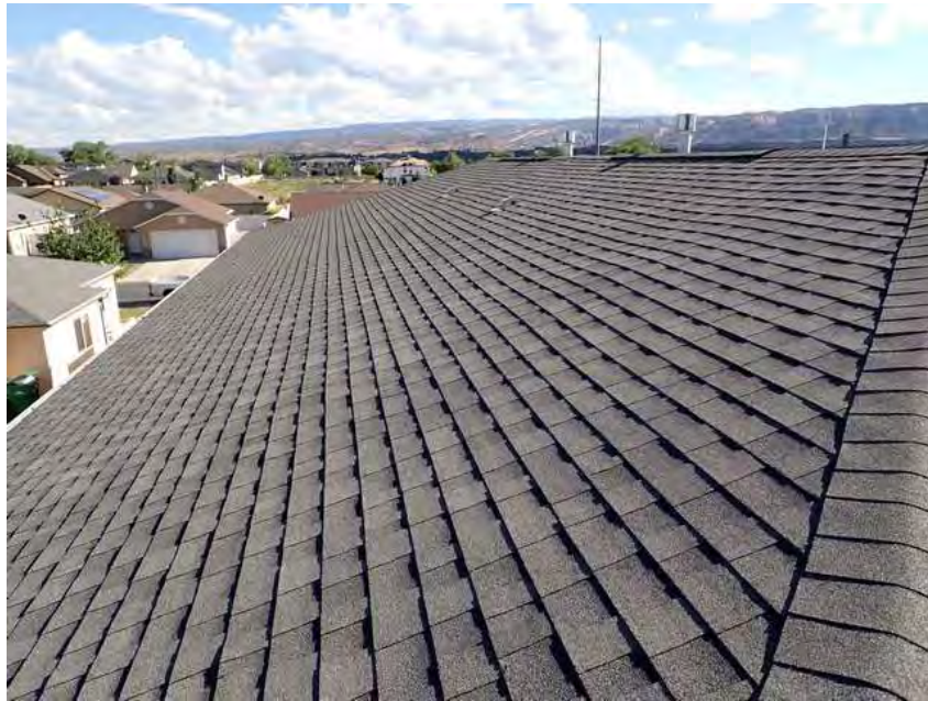
267. Building 15. Roof overview.
