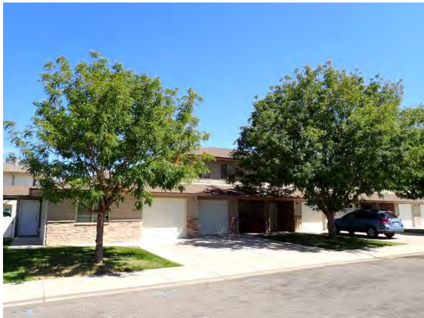
198. Building 12. Front overview.
