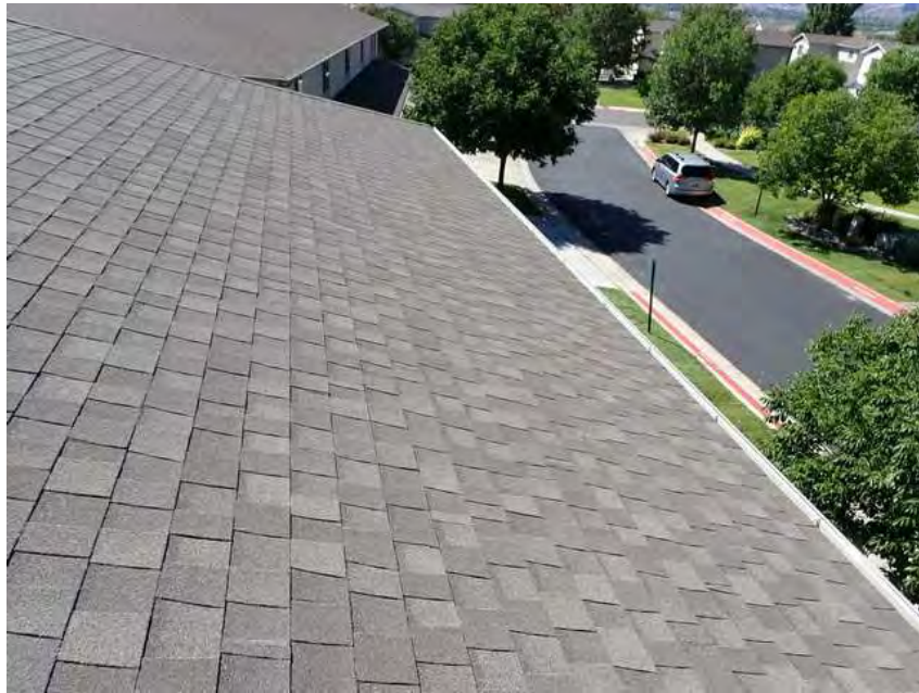
151. Building 8. Roof overview.
