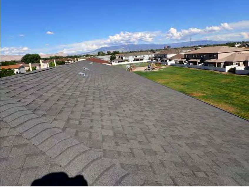
283. Building 16. Roof overview.
