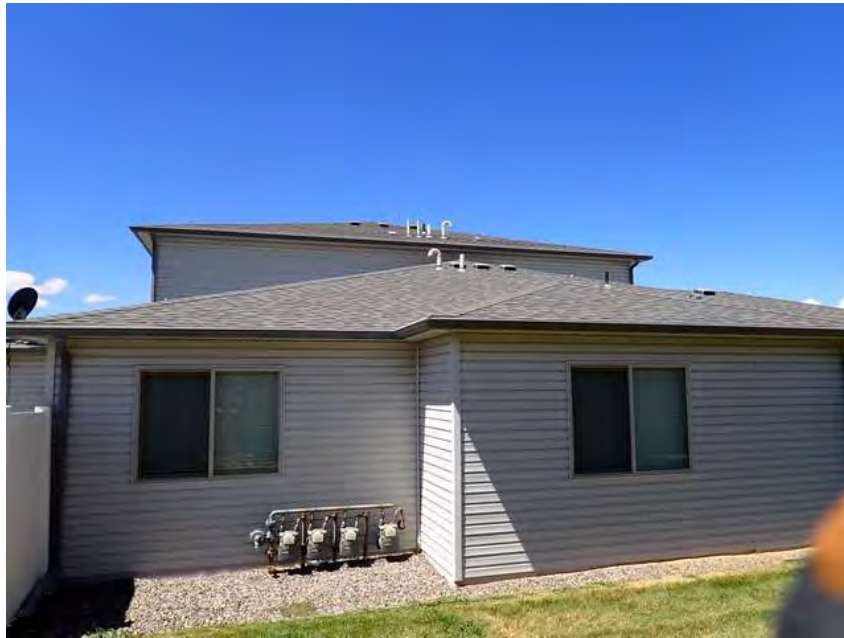
273. Building 16. Left overview.
