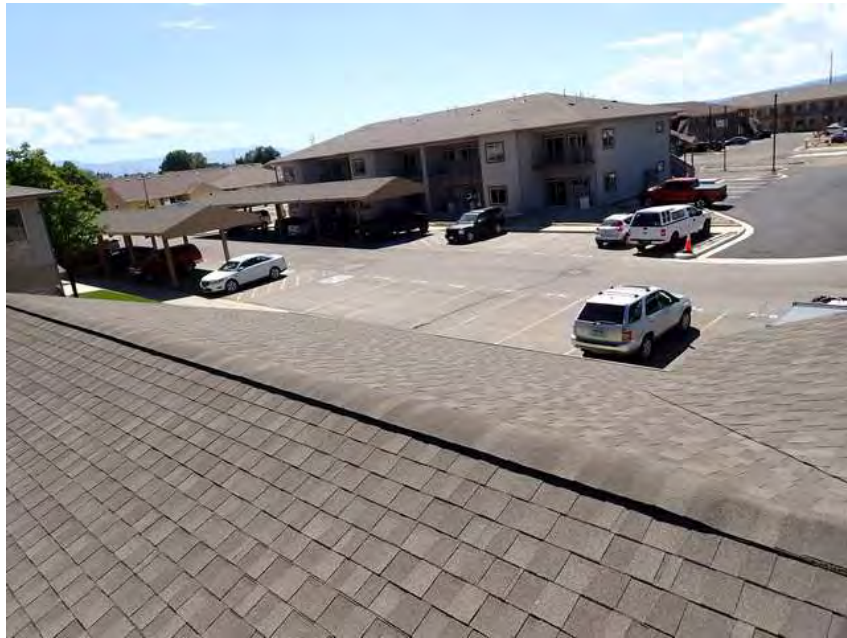
449. Club House. Roof overview.
