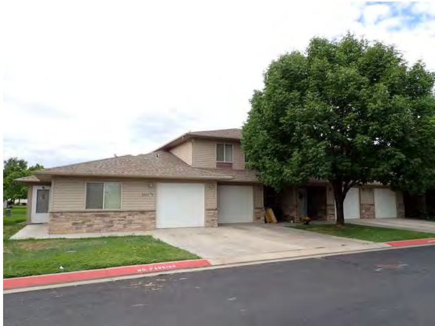
74. Building 5. Front overview.
