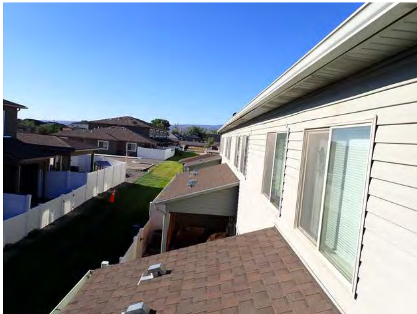
356. Building 21. Lower roof overview.
