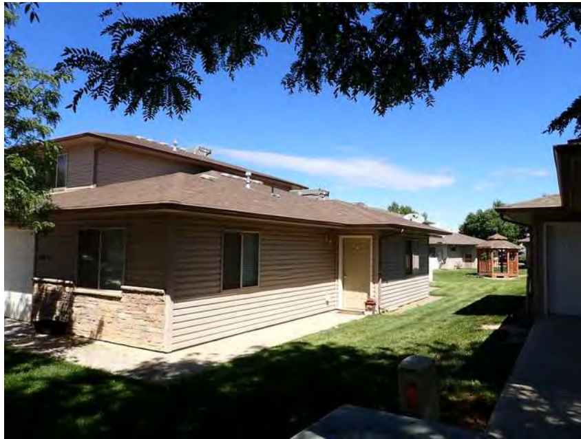
199. Building 12. Right overview.
