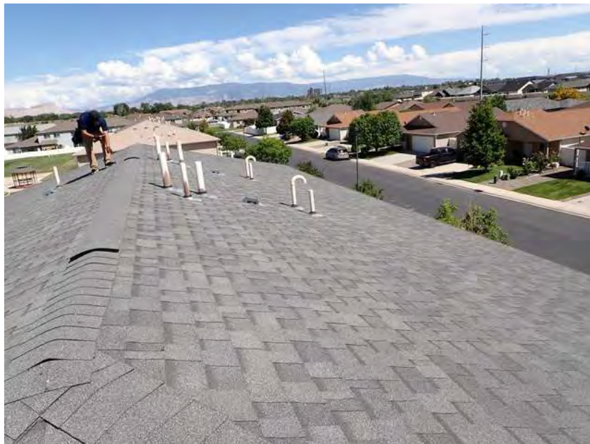
430. Building 24. Roof overview.
