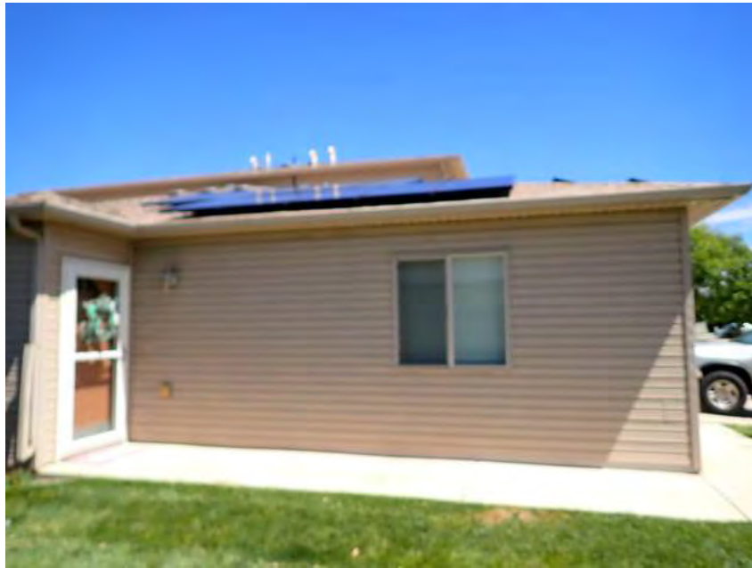
403. Building 23. Left overview.
