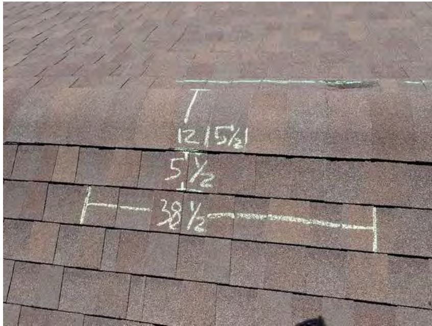
123. Building 6 Shingle dimensions.
