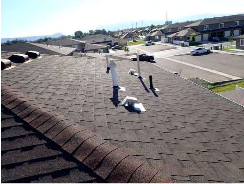
359. Building 21. Roof overview.
