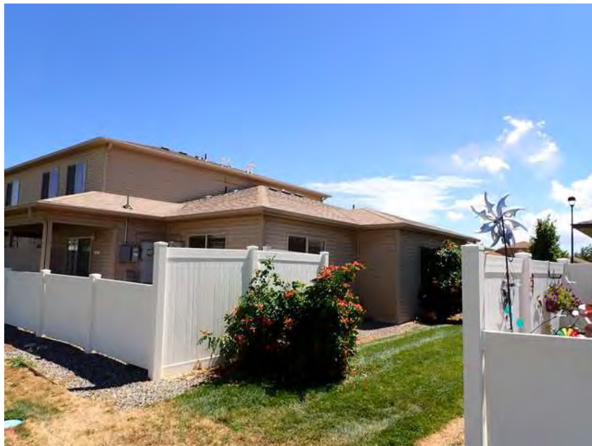
402. Building 23. Left overview.
