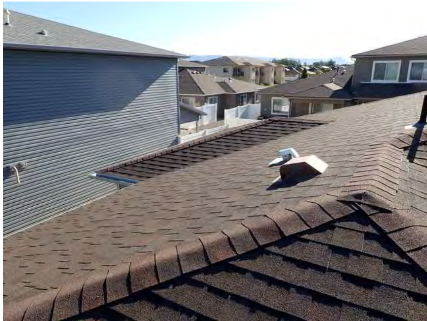
354. Building 21. Roof overview.
