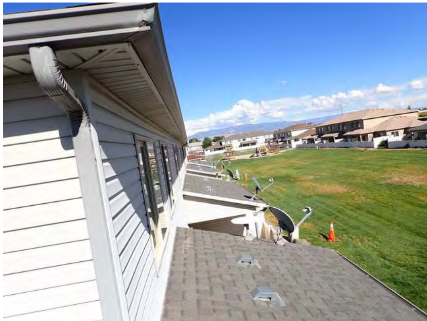
276. Building 16. Lower roof overview.
