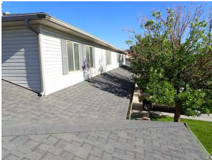
222. Building 13. Lower roof overview.
