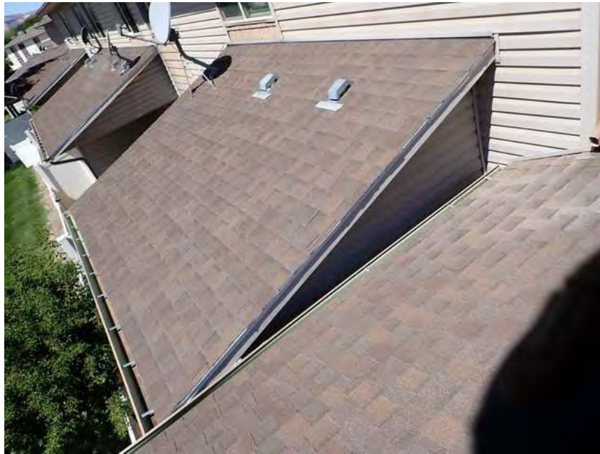
97. Building 6 Lower roof overview.
