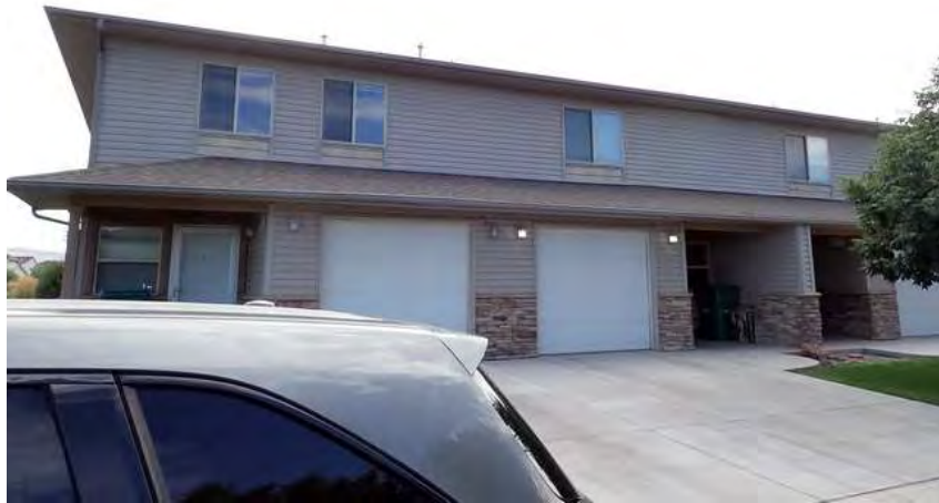
141. Building 8. Front overview.
