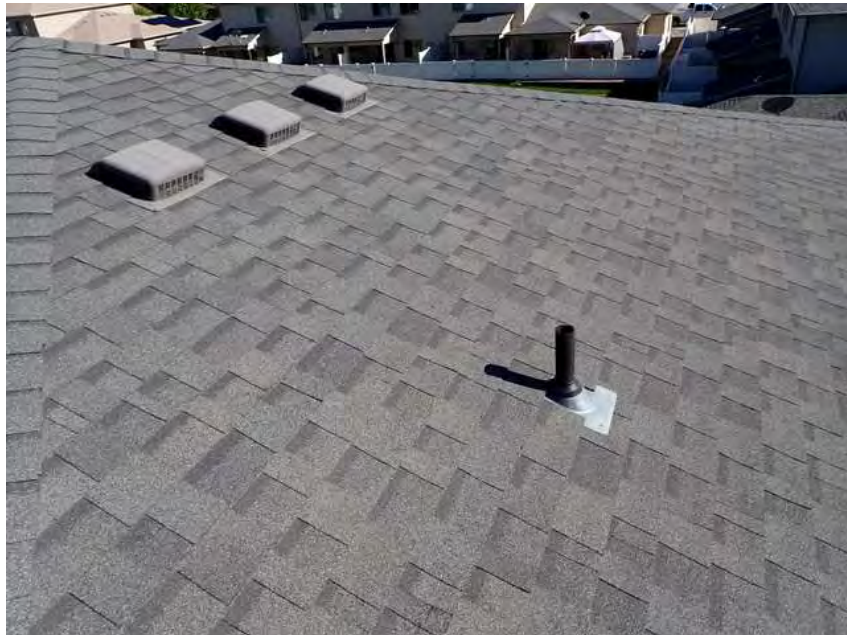
282. Building 16. Roof overview.
