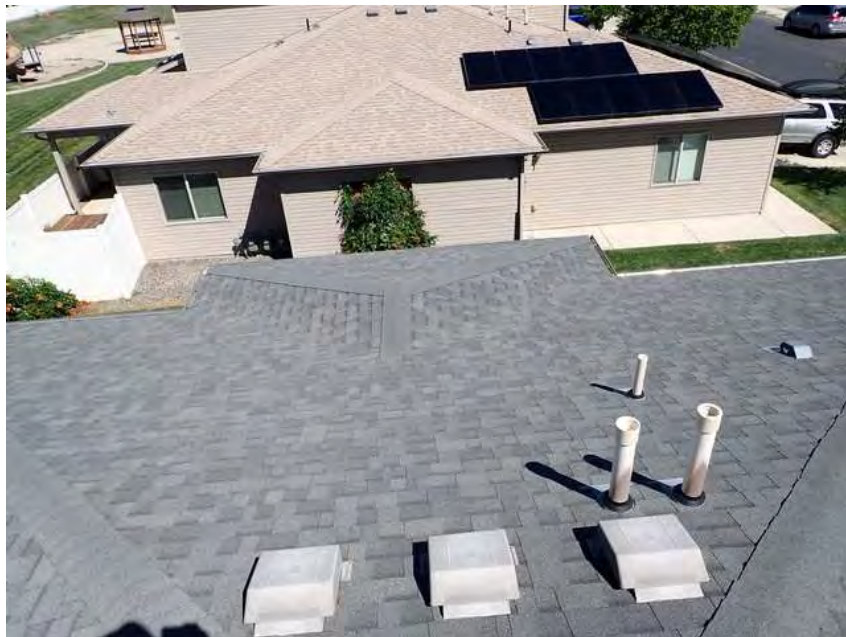
434. Building 24. Roof overview.
