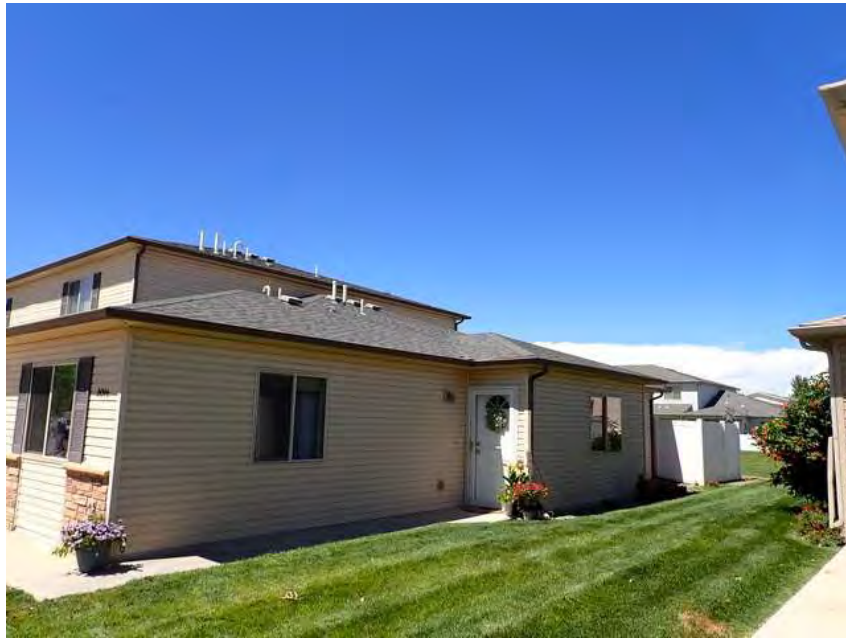
415. Building 24. Right overview.
