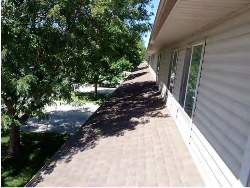
175. Building 10. Lower roof overview.
