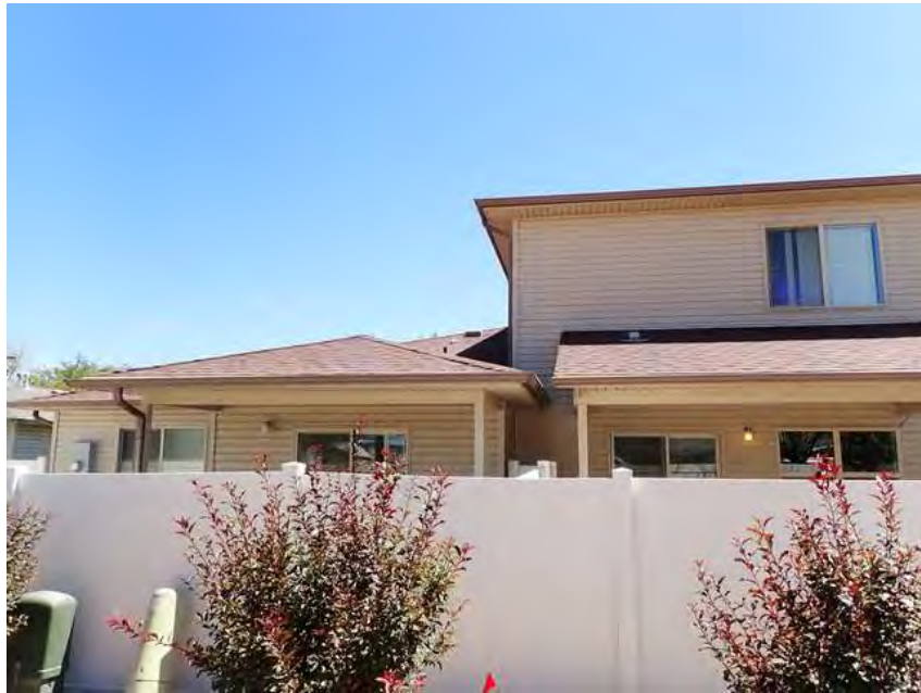
243. Building 14. Back overview.
