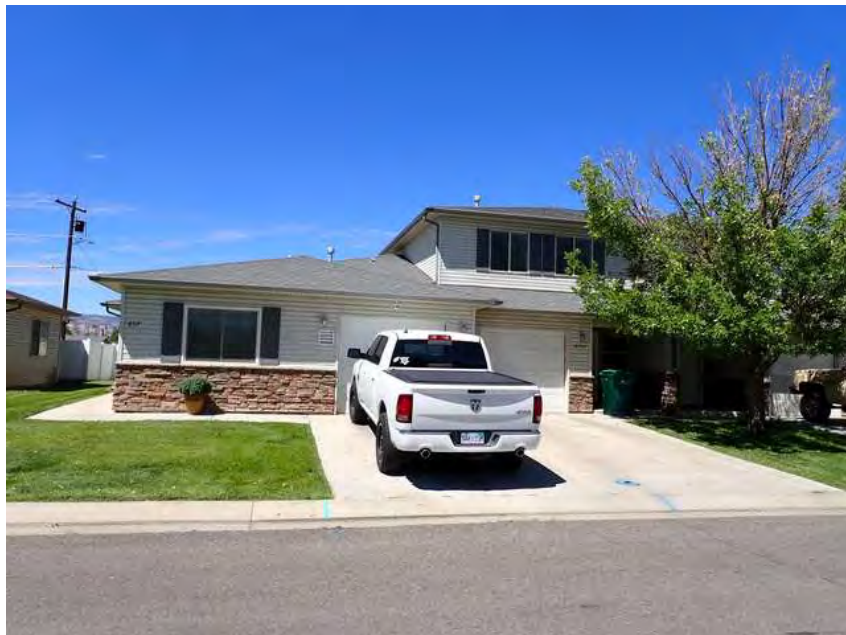
218. Building 13. Front overview.
