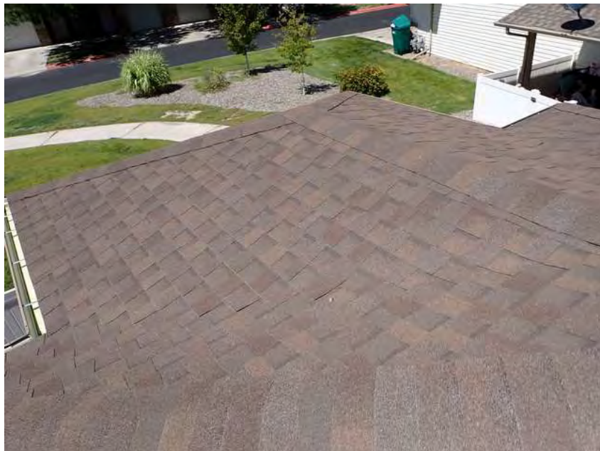
206. Building 12. Roof overview.
