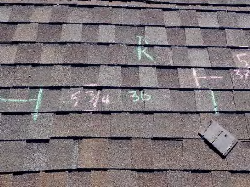
27. Building 1. Dimension of repair shingles.
