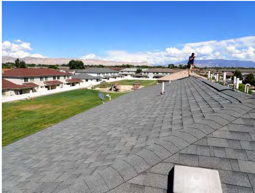
429. Building 24. Roof overview.
