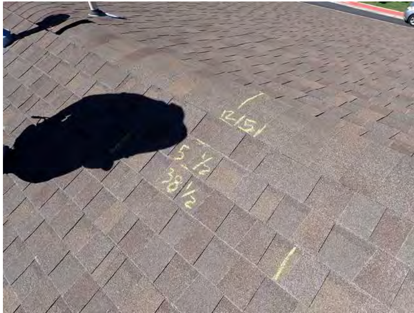
167. Building 9. Shingle dimensions.
