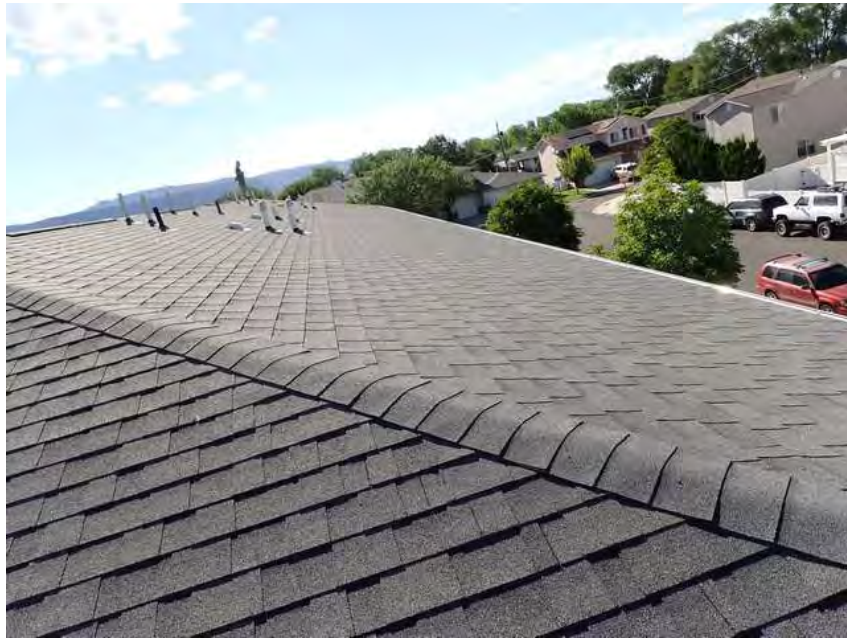
281. Building 16. Roof overview.
