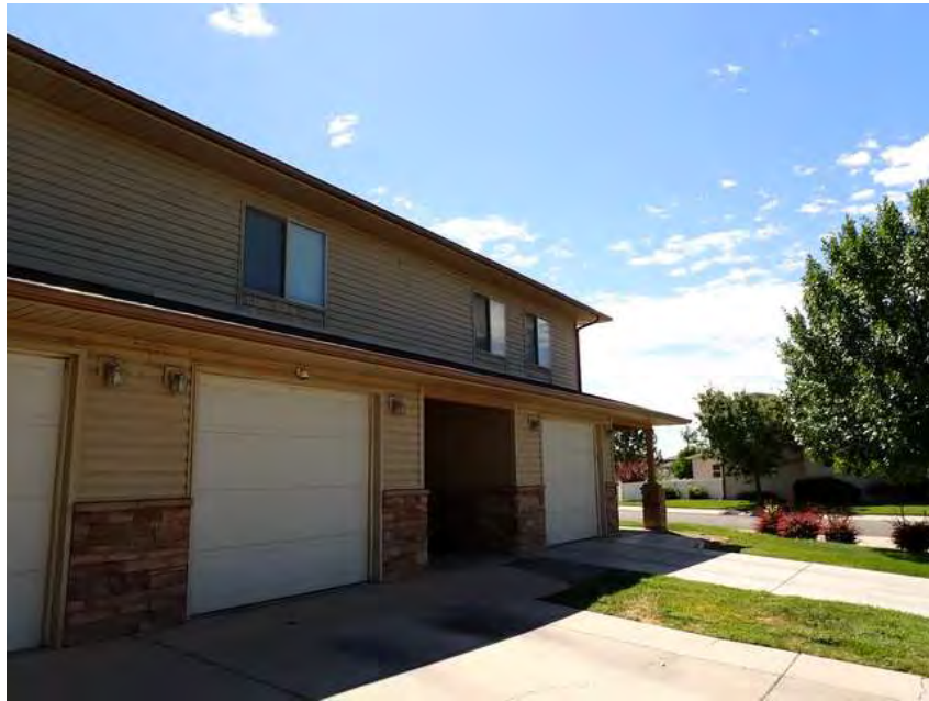
155. Building 9. Front overview.
