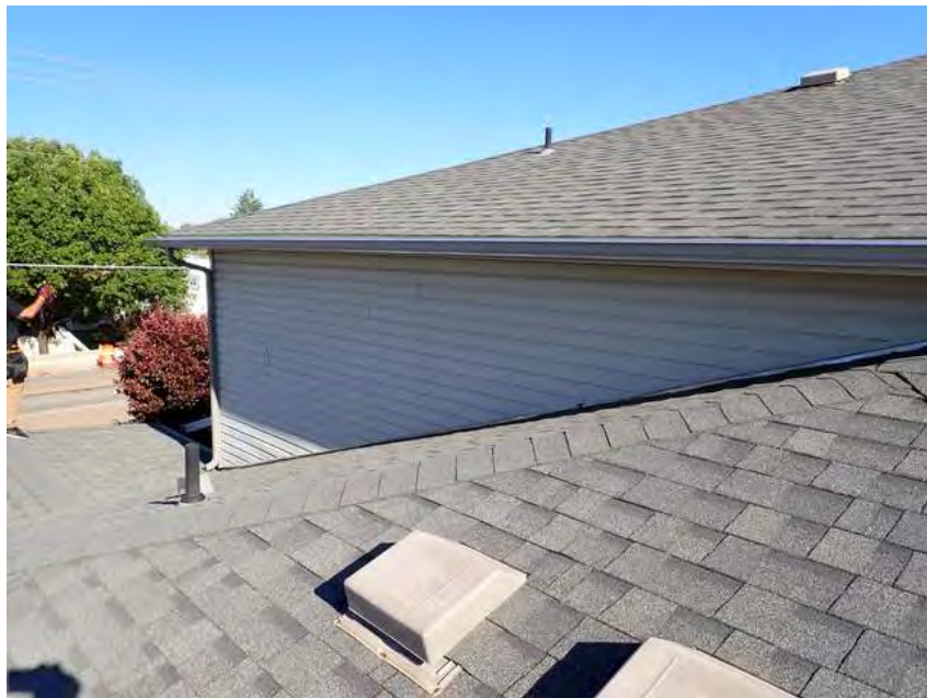
224. Building 13. Roof overview.
