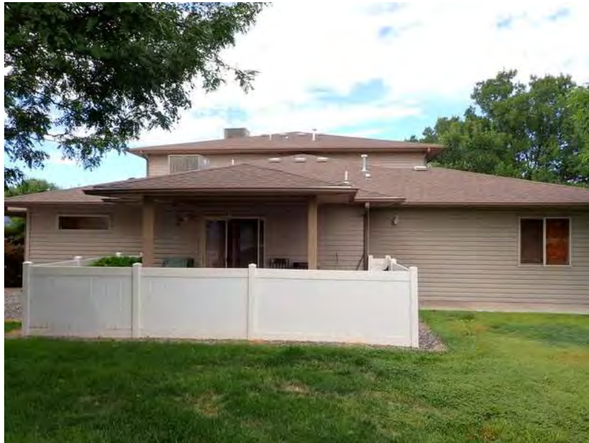
95. Building 6 Left overview.
