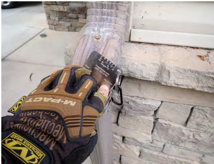
6. Building 1. Downspouts made from aluminum, typical throughout property.
