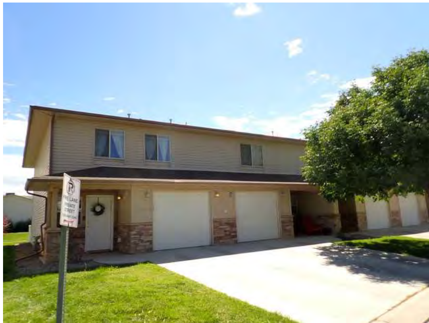
154. Building 9. Front overview.
