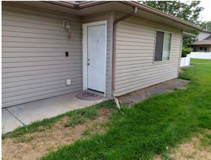
93. Building 6 Right overview.
