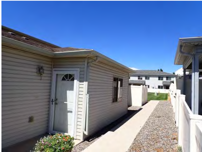
365. Building 22. Right overview.
