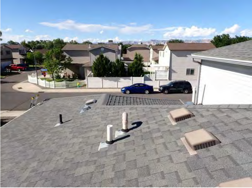
277. Building 16. Roof overview.
