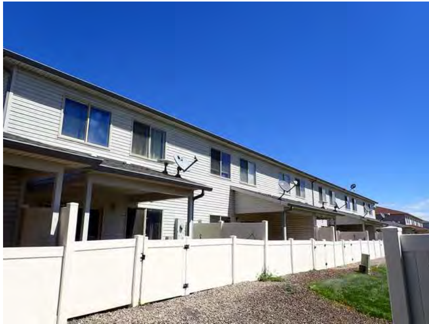
271. Building 16. Back overview.
