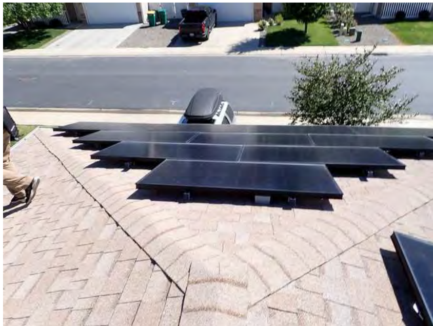
406. Building 23. Roof overview.
