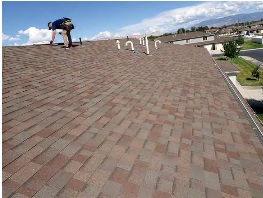
379. Building 22. Roof overview.
