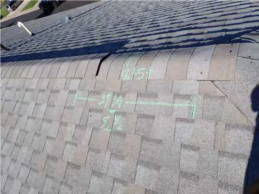
346. Building 20. Shingle dimensions.
