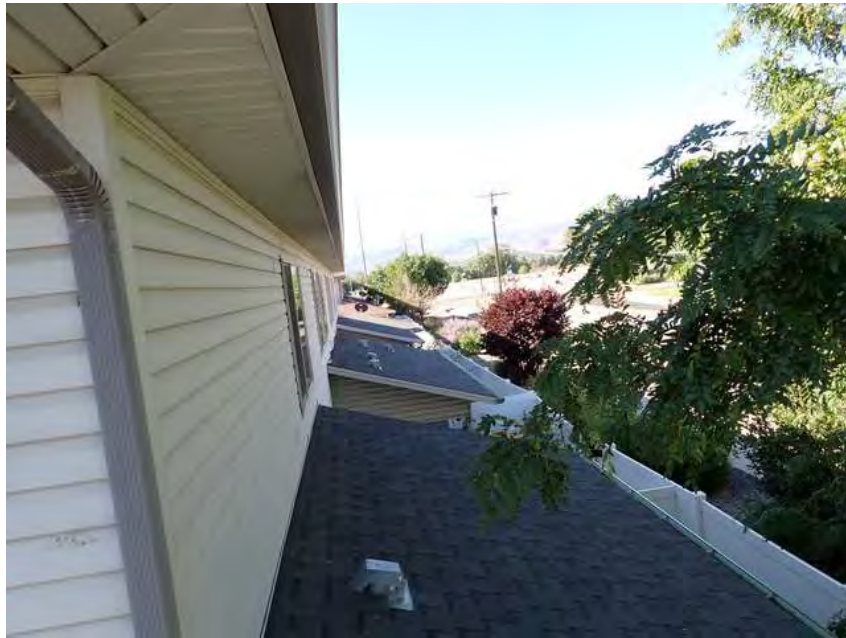
233. Building 13. Lower roof overview.
