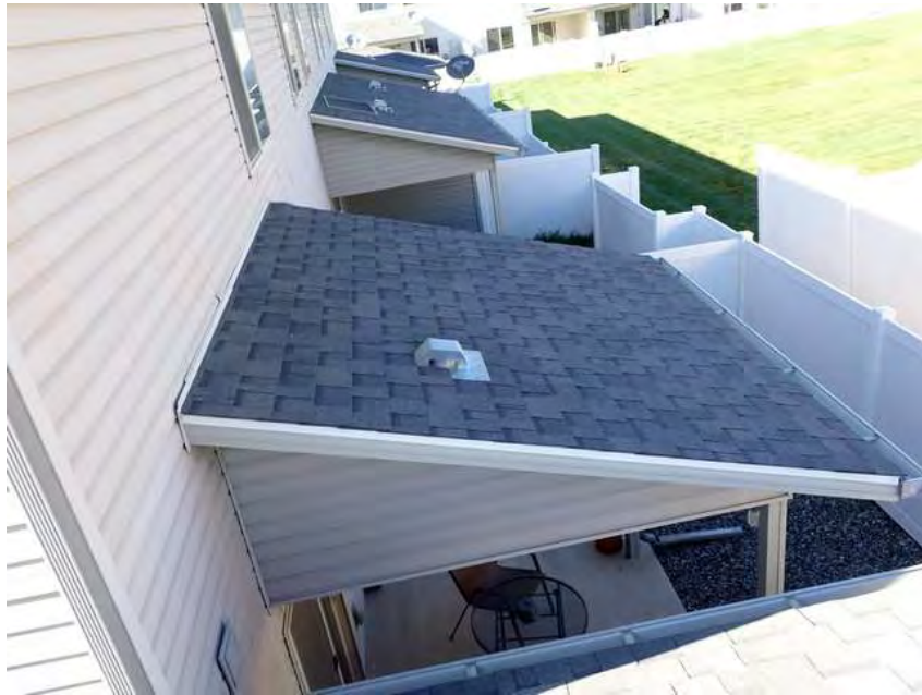
265. Building 15. Lower roof overview.
