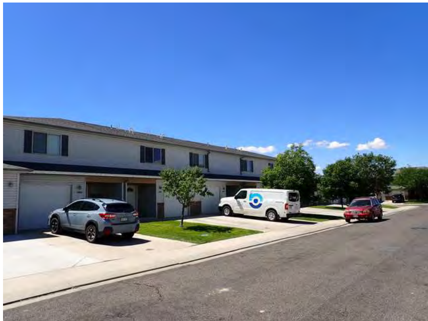
270. Building 16. Front overview.
