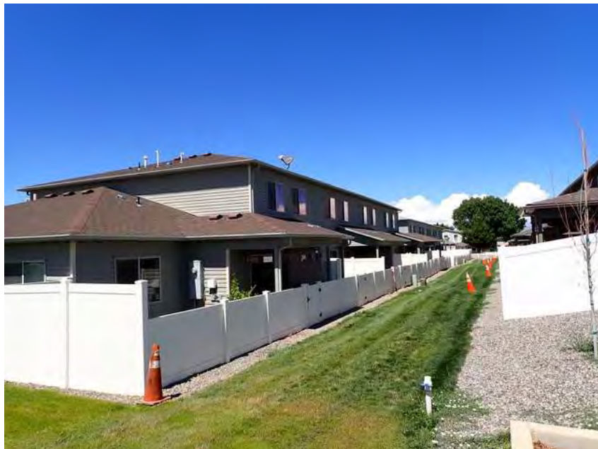
352. Building 21. Back overview.
