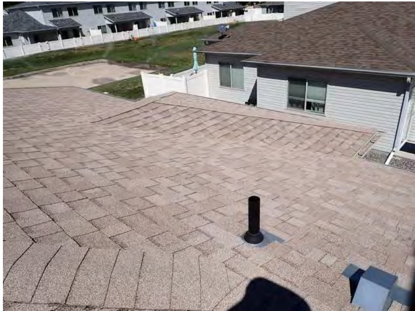
410. Building 23. Roof overview.
