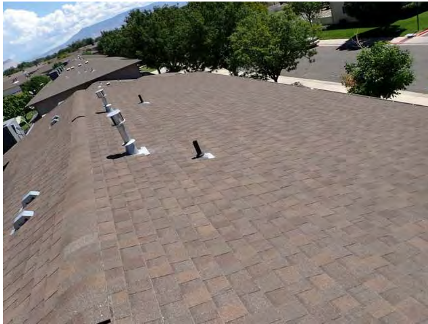
211. Building 12. Roof overview.
