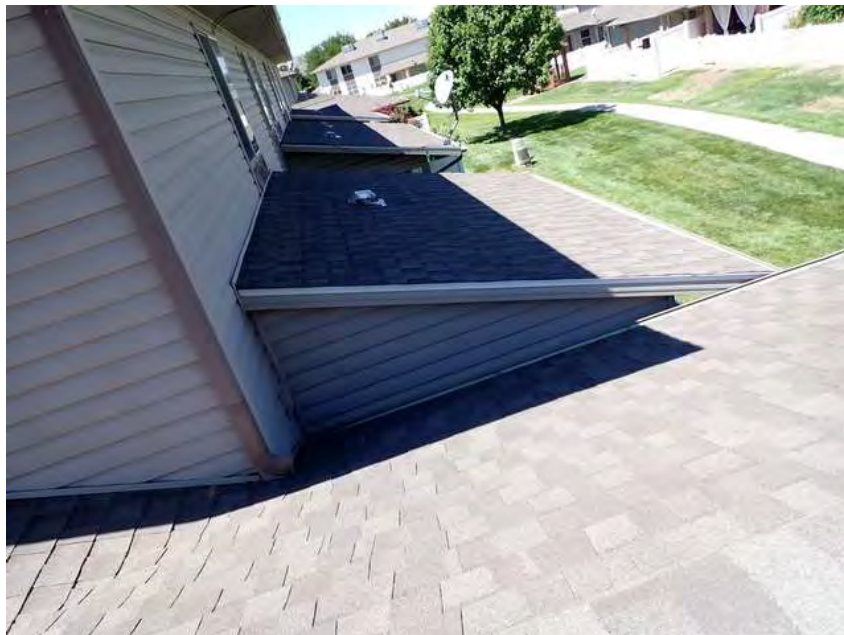
188. Building 11. Lower roof overview.
