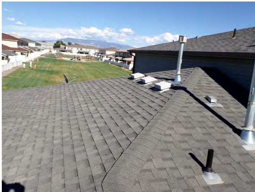
262. Building 15. Roof overview.
