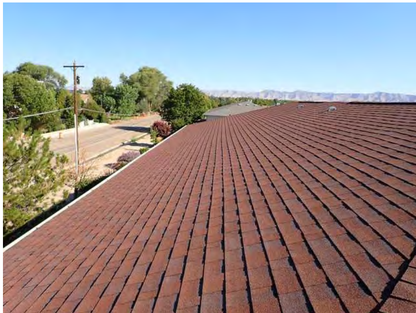
250. Building 14. Roof overview.
