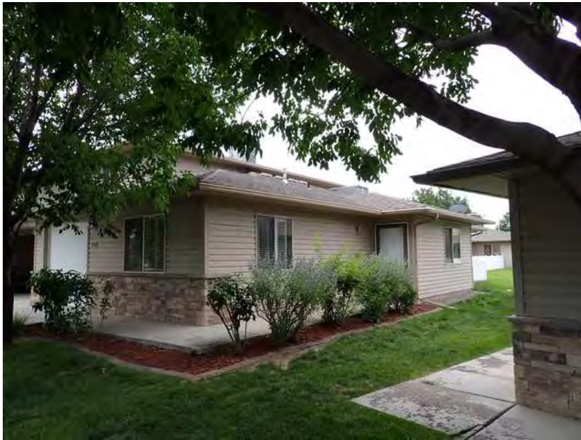
75. Building 5. Right overview.
