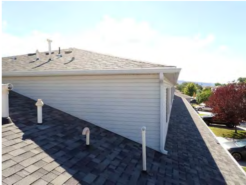
311. Building 18. Lower roof overview.
