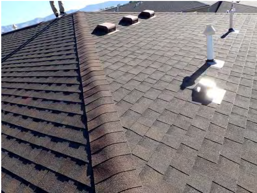
360. Building 21. Roof overview.
