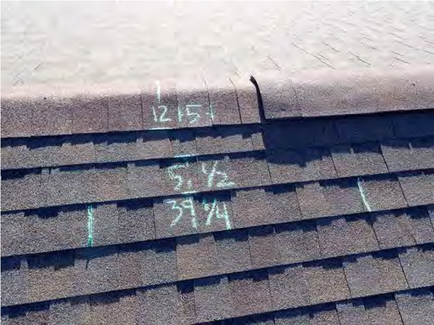
362. Building 21. Shingle dimensions.
