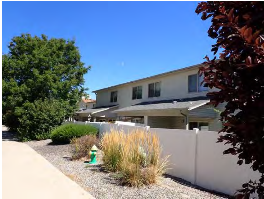
221. Building 13. Back overview.
