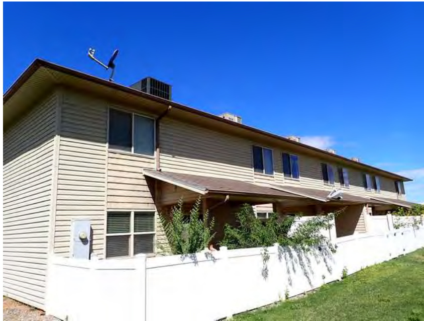
159. Building 9. Back overview.
