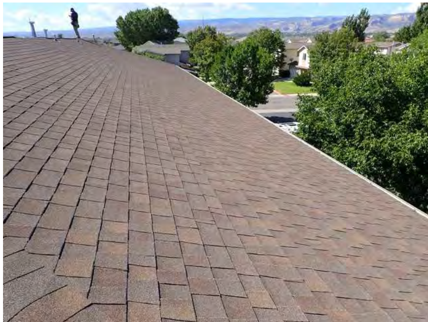
164. Building 9. Roof overview.
