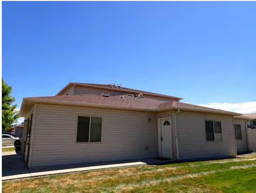
287. Building 17. Right overview.
