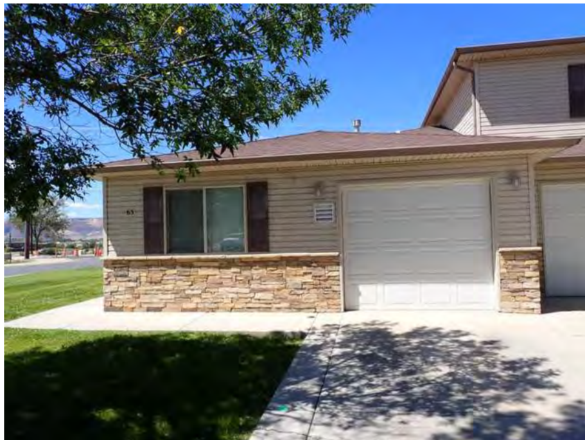
238. Building 14. Front overview.
