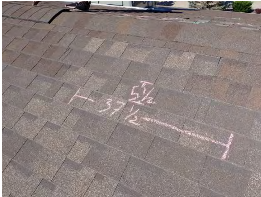
29. Building 1. Dimension of repair shingles.
