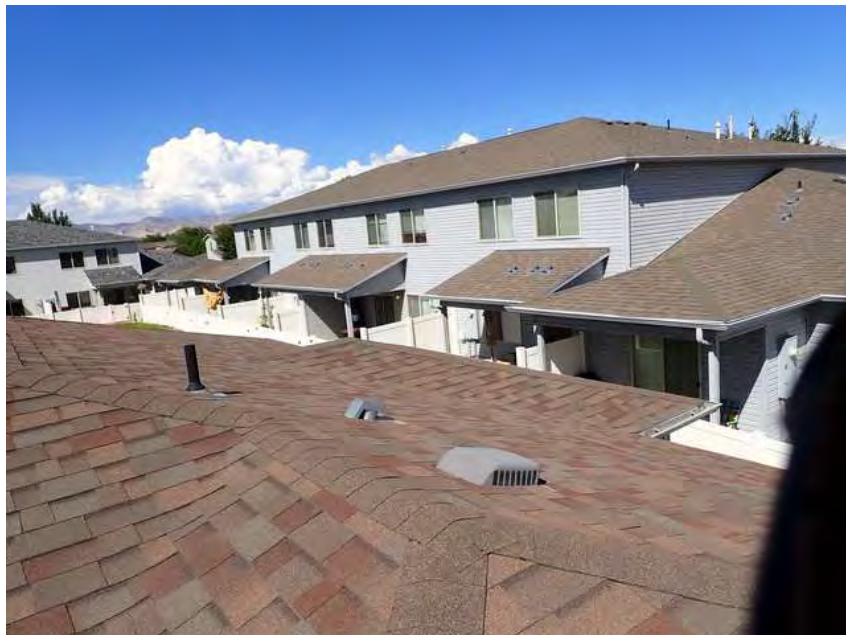
376. Building 22. Roof overview.
