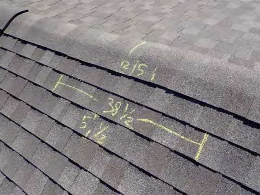
42. Building 2. Shingle dimensions.
