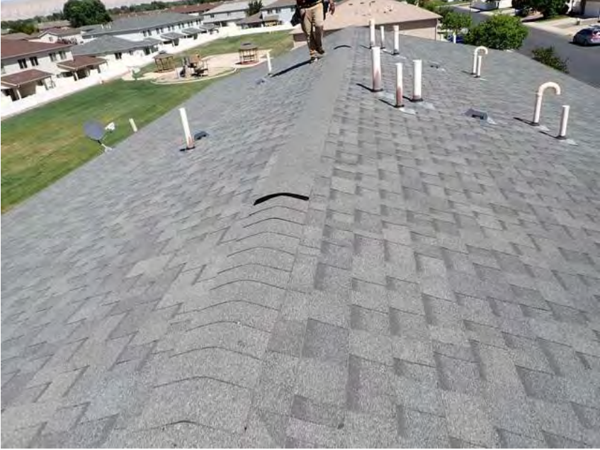
431. Building 24. Roof overview.
