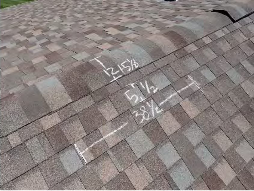
55. Building 3. Shingle dimensions.
