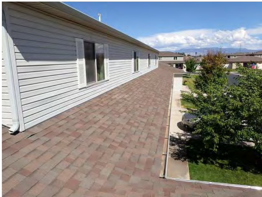
368. Building 22. Lower roof overview.
