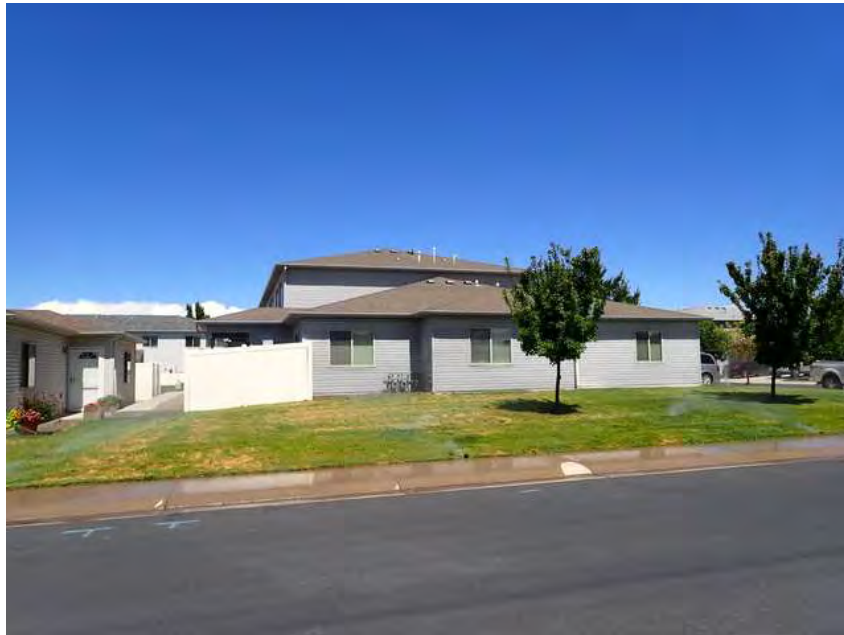
323. Building 19. Left overview.
