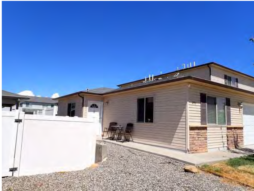
419. Building 24. Left overview.
